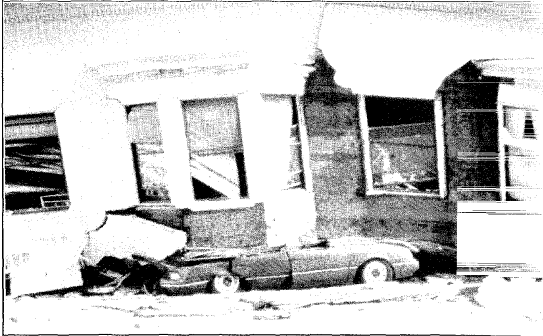
Damage During the Loma Prieta Earthquake
