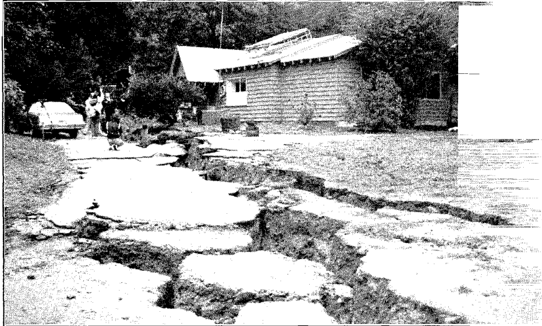
Ground Movement During the Loma Prieta Earthquake
