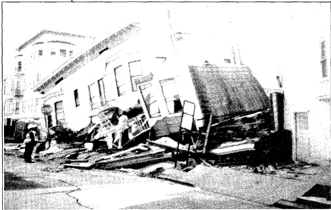
Damage During the Loma Prieta Earthquake
