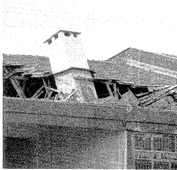
Photo 12 Toppled chimney (Erzincan Sanayi Sitesi)
