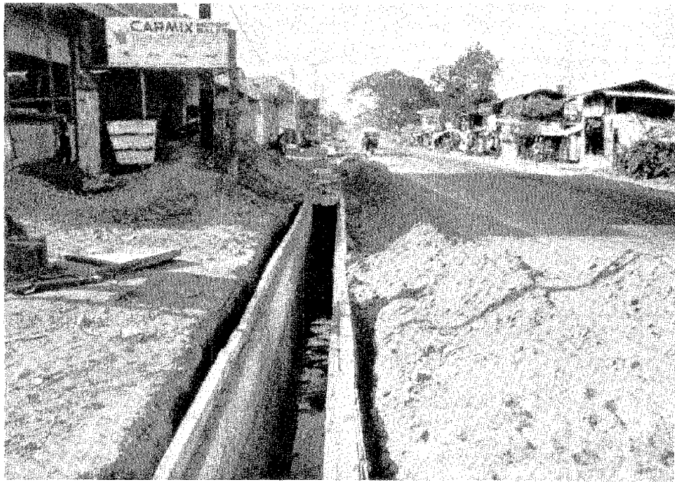
Photo 5 : Open Canal Under Construction
