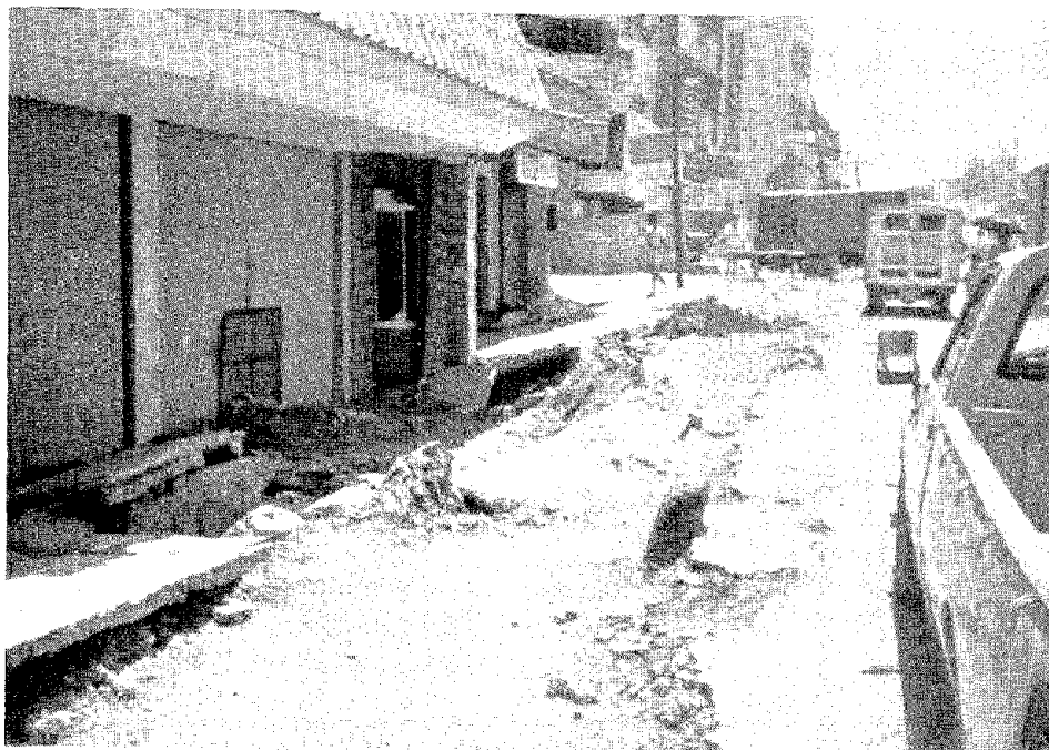
Photo 1 : Damaged Drainage Pipe
