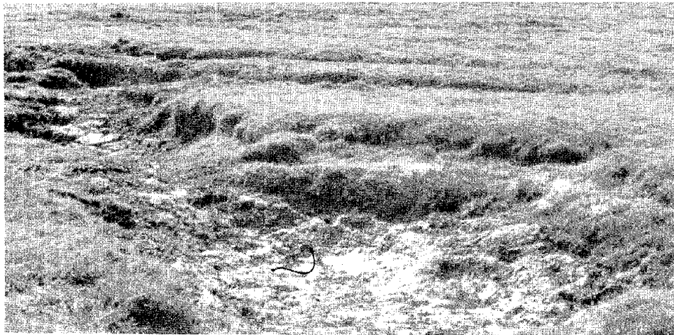
Photo 27 Ground failure at Karasu (note 1000 mm separations and partial subsidence)
