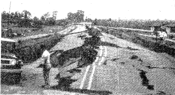
Photo 1 Fissures and lateral spreading of the road embankment on Route 32 near Siquirres
