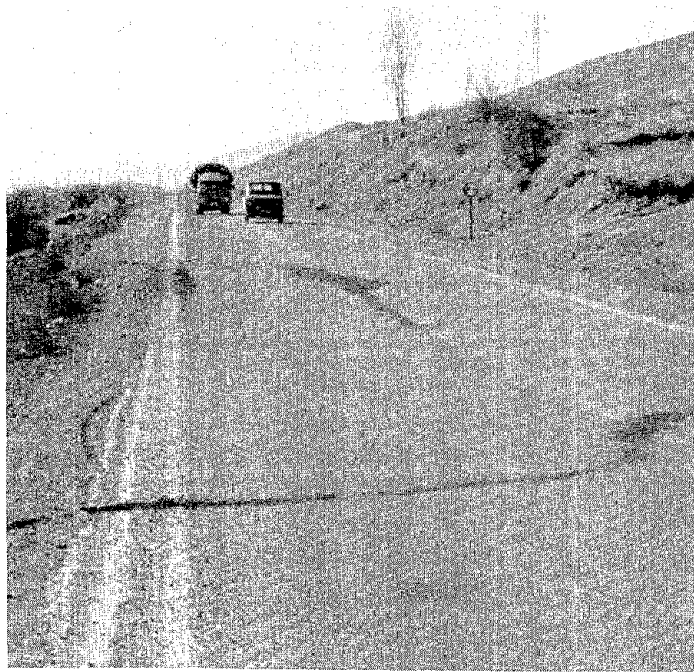
Photo 14 Displaced highway for Erzurum & Erzincan at Karasu
