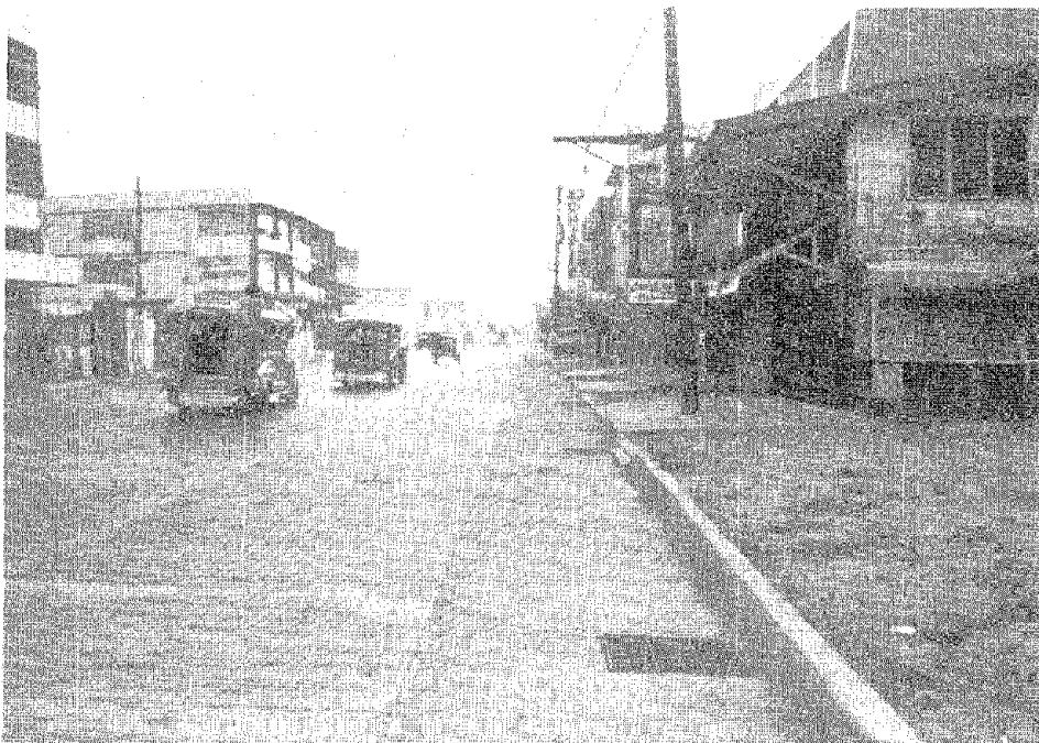
Photo 4 : Fully Reconstructed Roadway
