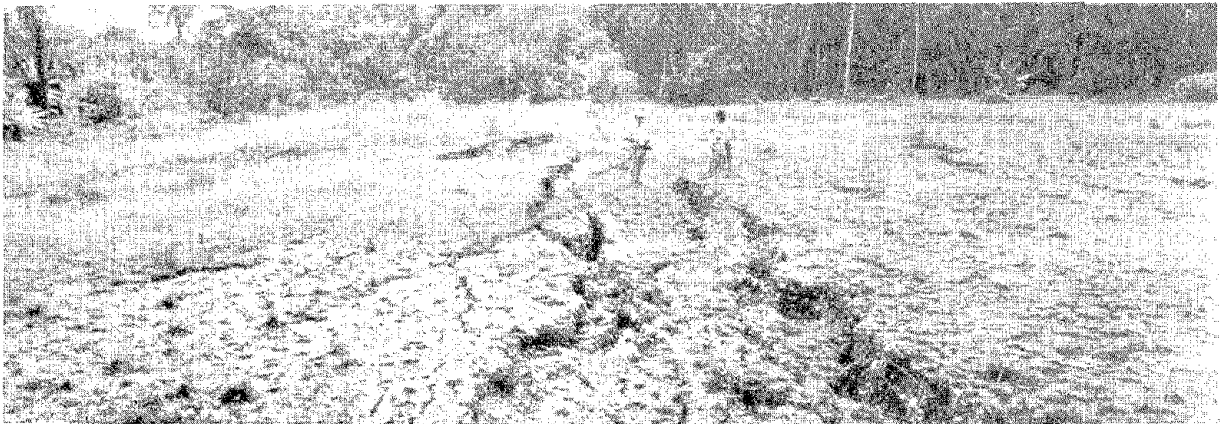
Photo 4 Ground failure of the embankment for the oil survey
