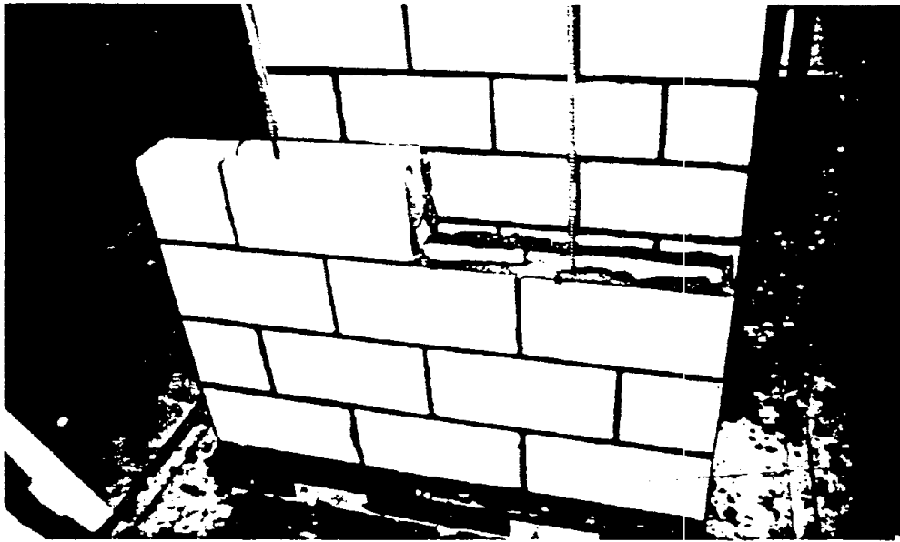
(a) Fully Grouted Walls
