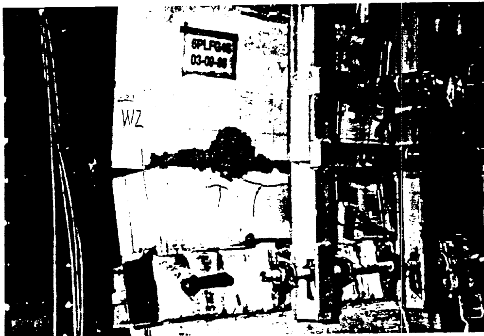
Figure 4.8 Spalling of Faceshell
