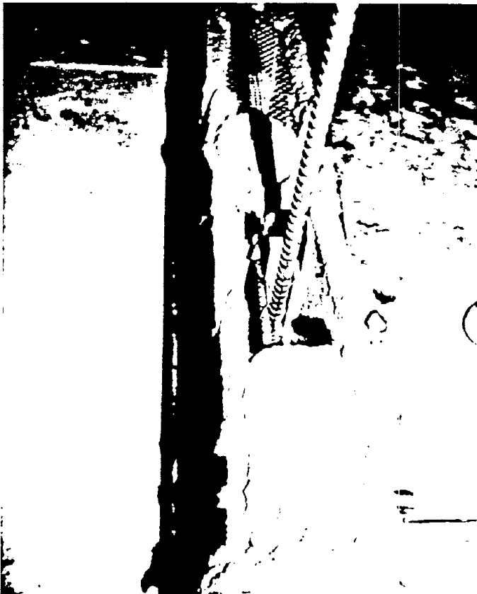
(b) Partially Grouted Walls
