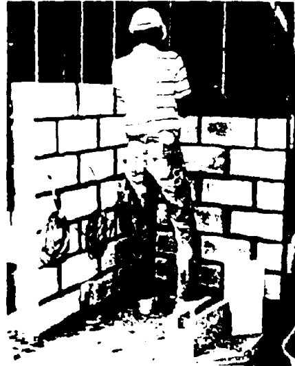
(b) Bottom Half Wall Completed
