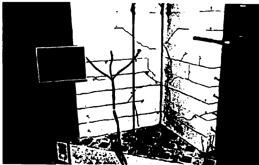
(b) Cracking Pattern in the Web
