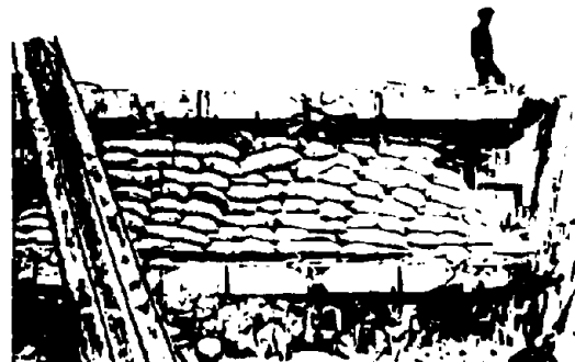
Overloaded commercial building
