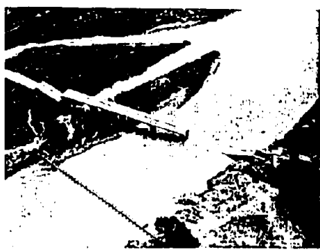
Figure 13. Collapse of the Lo-Gallardo Bridge during the 1985 Chile EQ [EERI 1986]
