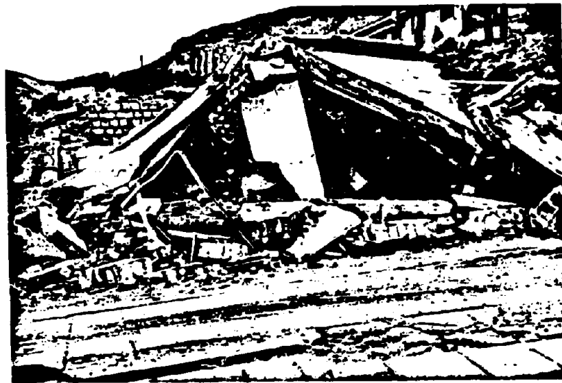
Figure 2. Collapsed hospital in Rostamabad
