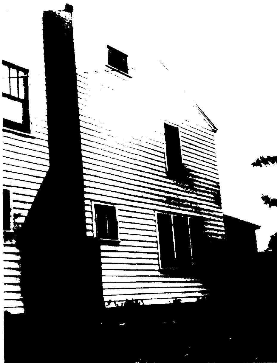
Figure 2: Currently, the only surviving photo of the 1944 earthquake damage is one of this chimney at the Nicola residence, 129 North Main Street. Over 90% of the chimneys in Massena were damaged or destroyed.
