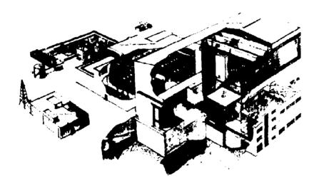
FIGURE 2 This facility in Tadotsu, Japan, houses a 15-m by 15-m table that can provide strong earthquake shaking to a 1,000-ton test specimen. In addition to the shake table with its actuating mechanism, this facility contains elaborate control equipment, data-recording equipment, and computers. Ancillary facilities are housed in adjacent buildings.
