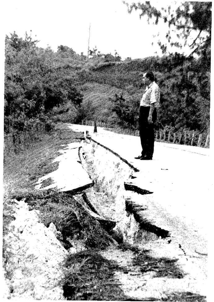
Figure 6-4: Soil failure in the form of slumping or spreading damaged roadways in certain locations on the island. Concrete beam bridges suffered minor cracking and slumping at abutments. Water mains attached to the sides of bridges tended to fail due to differential movement at the interface of abutments (arrow, below)
