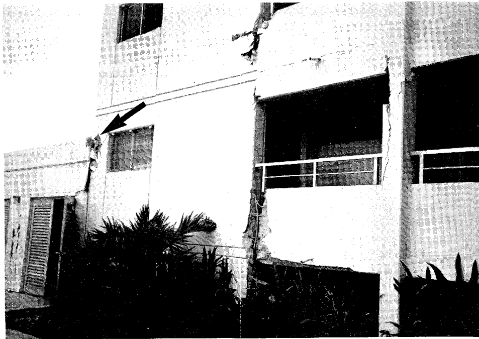
Figure 5-4: Shattered columns, shear cracking at spandrels, and pounding damage at the interface of the one-story mechanical building (at left) are seen along the front fact of the Alupang Cove.
