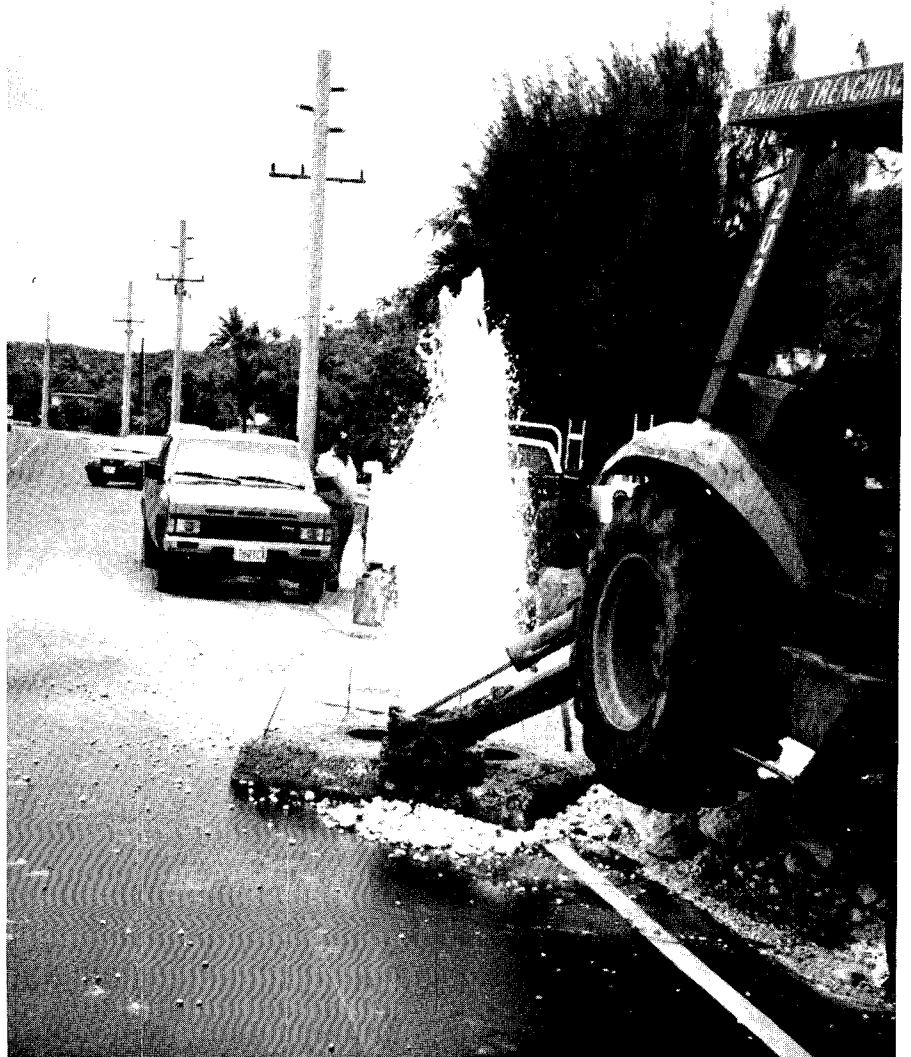
Figure 6-3: The Public Utility Agency of Guam (PUAG) reported no damage to their welded steel storage reservoirs or the Uguum Water Treatment Plant (above). Over 100 breaks occurred in the island's 500 miles of buried water mains. Repairs are underway to a broken main near Agana at right.
