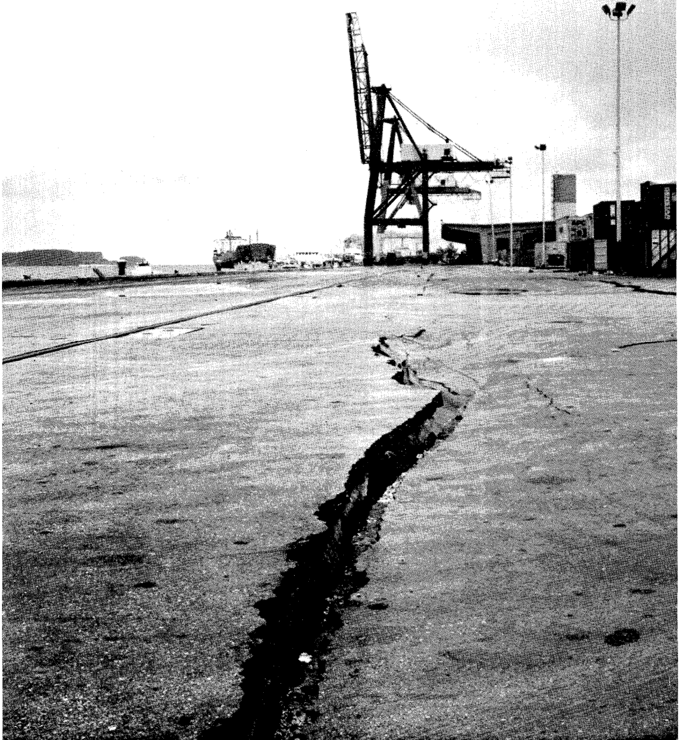
Figure 6-5: Perhaps the most serious effect from the earthquake was due to spreading of fill beneath the crane rails in the container handling section of the commercial port. Offset of the rails severely limits the travel distance of the gantry cranes, curtailing off-loading of container ships, the primary source of supply to the island.
