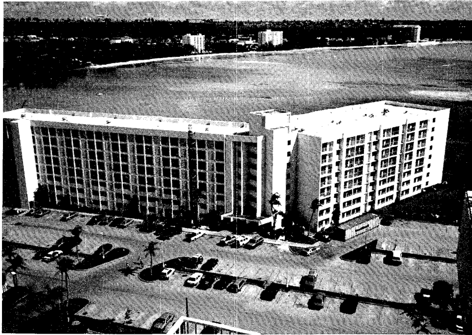
The Alupang Cove Condominium Complex suffered effects typical of mid-to high-rise buildings in the tourist area.
