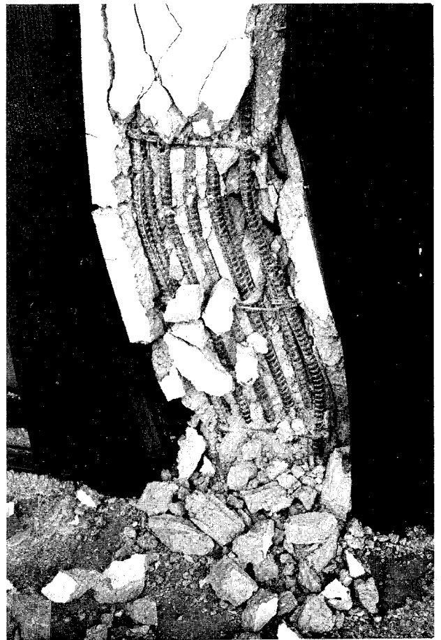
Figure 5-3: The Grand Hotel near Tumon Bay suffered the most extensive damage of low-rise structures on the island. A soft first story effect shattered columns at the base of the building and shifted the upper three floors nine inches relative to the ground.
