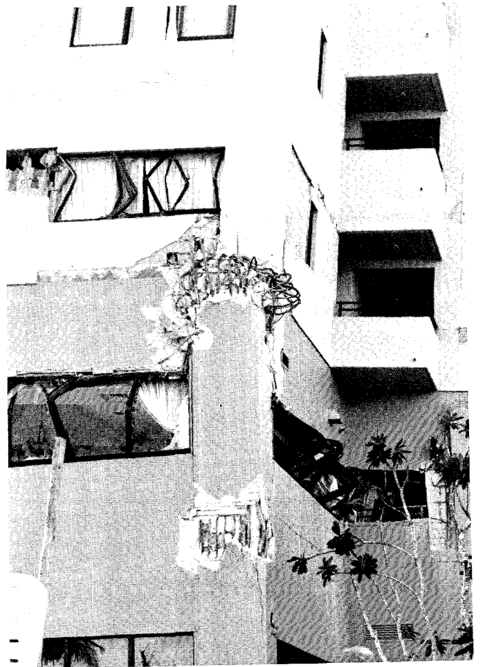
Figure 5-2: A partial collapse occurred in the seaward wing of the Royal Palms Condominiums. A discontinuity in masonry in-fill at the second floor concentrated shear on the corner columns.
