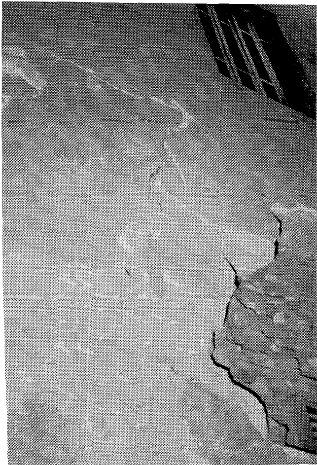
FIGURE 1-10 Fallen plaster exposed stone/mortar wall.
