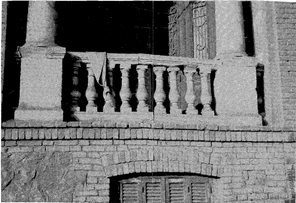
FIGURE 1-15 Dislocated stone balcony parapet (El-Khalaa district).
