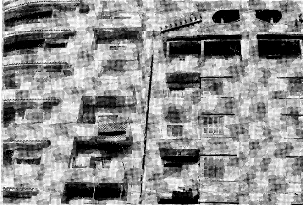
FIGURE 1-16 Open crack between reinforced concrete building 1 (Kadri St., Elsayyeda Zenab district).
