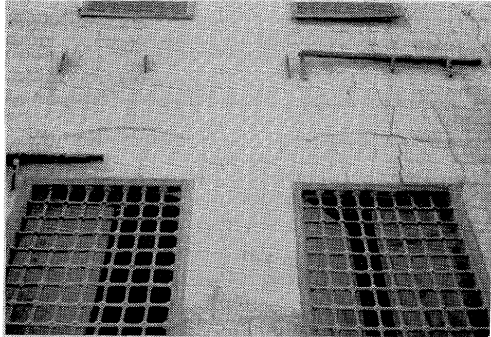
FIGURE 1-42 Sultan El-Ghuri Mosque: Cracks in mortar at keystone above window.
