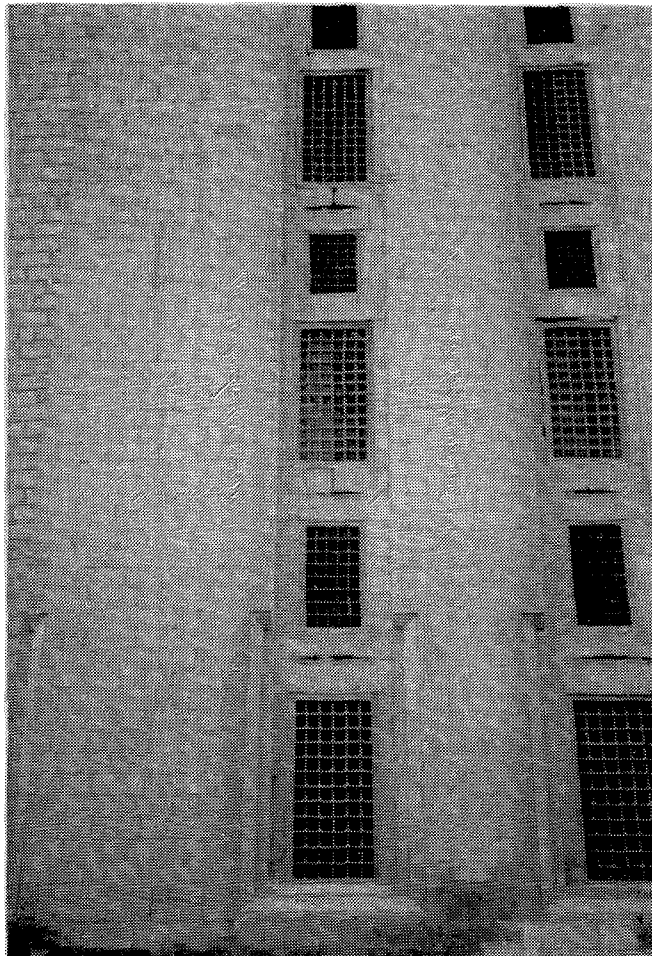
FIGURE 1-42 Sultan El-Ghuri Mosque: Cracks in mortar at keystone above window.
