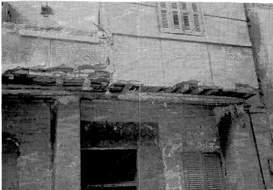
FIGURE 1-12 Fallen plaster along wood beam ceiling, Misr Elkadima district.
