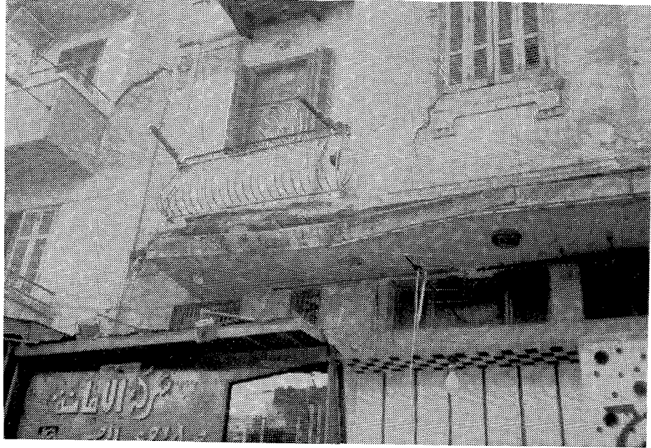
FIGURE 1-7 Shear crack at window corner (Elsayyeda Zenab district).
