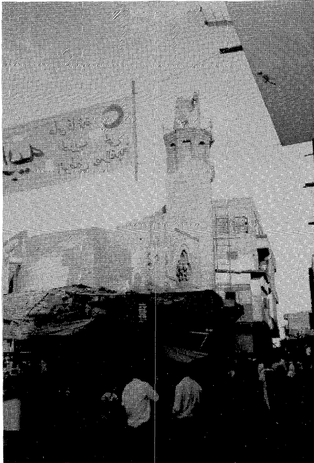
FIGURE 1-44 Partially collapsed masonry minaret top (Port-Said Street, Sayyeda Zenab district).
