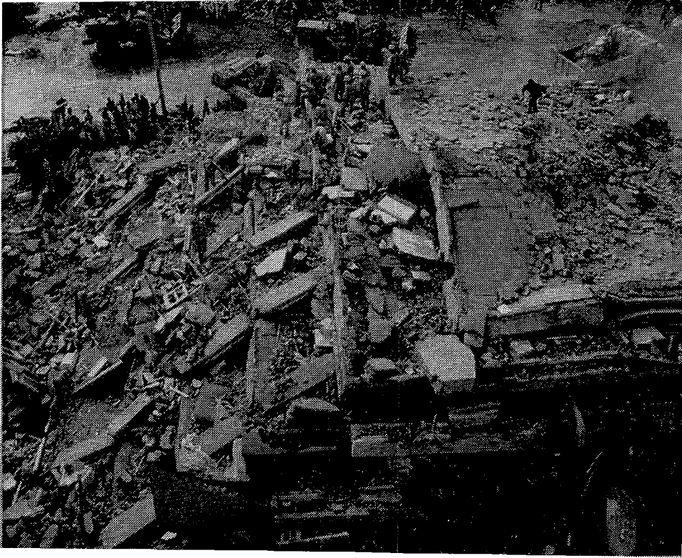
FIGURE 1-6 Collapsed 14-story reinforced concrete structure (Heliopolis district). [National Geographic, Vol. 183, No. 4, April 1993.]
