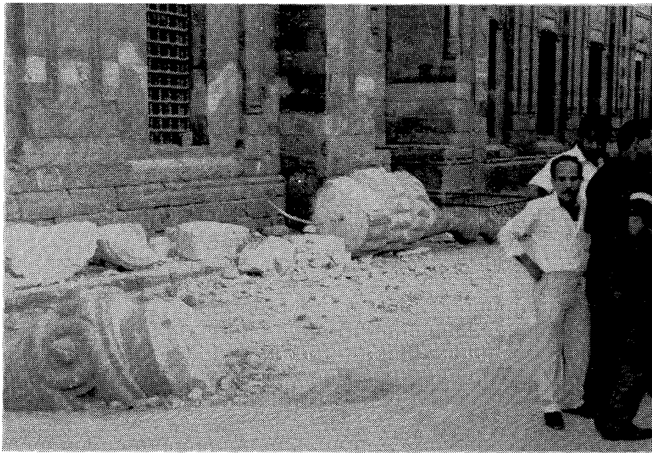
FIGURE 1-33a Toppled minaret tops (Al-Hanafi Mosque).
