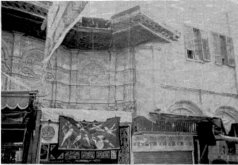
FIGURE 1-14 Fallen and dislocated heavy stone ornaments in an antique building in Elghouriah district.
