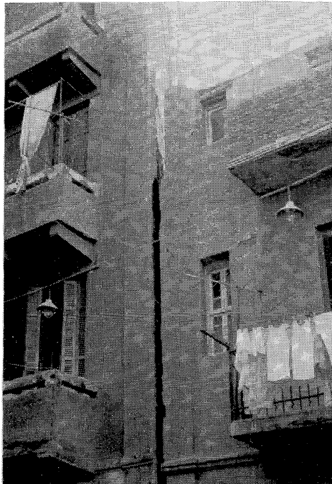
FIGURE 1-20 Open crack between reinforced concrete building 4 (Kadri Street, Elsayyeda Zenab).
