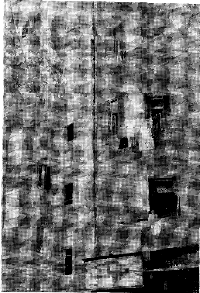
FIGURE 1-22 Open crack between reinforced concrete building 5 (Magless Elshaab Street, across from building of Figs. 1-17 and 1-18).
