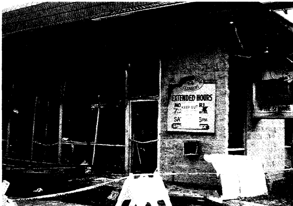
Figure 56 Fire damage in a single story commercial building.
