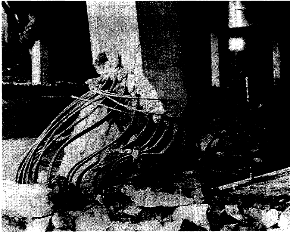
Figure 35 Damage to pier 3S-1 of State Route 118 at Bull Creek Canyon Channel, looking to the northwest
