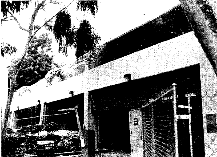
Figure 19 The cast-in-place concrete parking garage at the Kaiser Permanente Hospital complex in West Los Angeles collapsed in on itself. The moment frame that provided lateral resistance on the south face of the structure could not resist the out-of-plane forces apparently caused by the collapse of interior elements.
