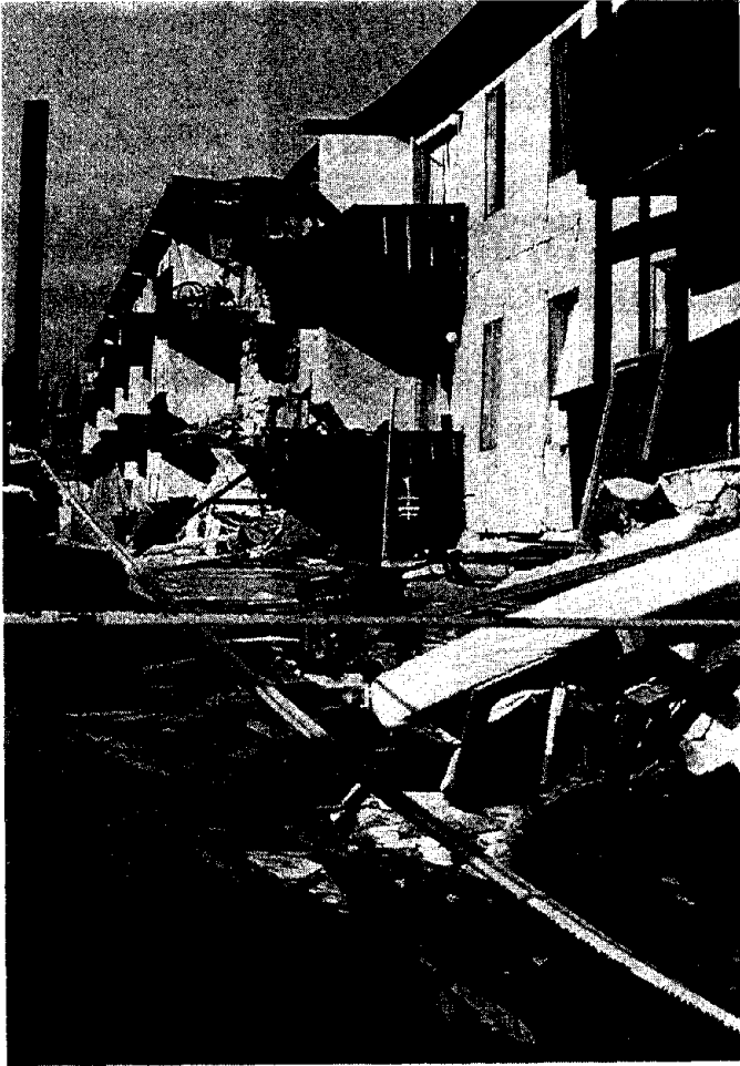
Figure 5 At the Northridge Meadows apartment complex near the epicenter the first story in several of the buildings collapsed, killing sixteen people. The second and third stories remained essentially intact. Large portions of the first story in these buildings were open space for parking. This type of collapse occurred in a significant number of similar apartment buildings throughout the affected area.
