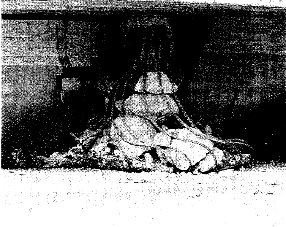
Figure 39 Northernmost pier of Bent 6 supporting westbound lane of I10 (west of Venice Blvd.)
