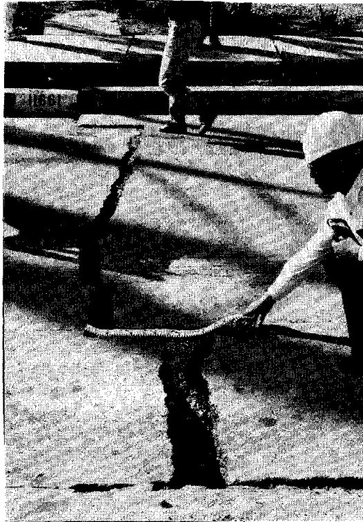
Photo 7.8 Lateral Movement of Pavement and Surface Soils as Large as 30 cm (Balboa Street, Granada Hill)
