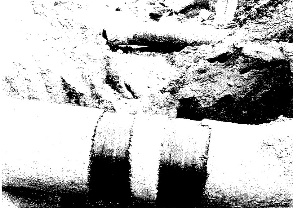
Figure 48 Ground extension along Balboa Boulevard resulted in the rupture of the same gas main and water main shown in Figure 47. The rupture of the gas main here caused a major fire that engulfed five houses.
