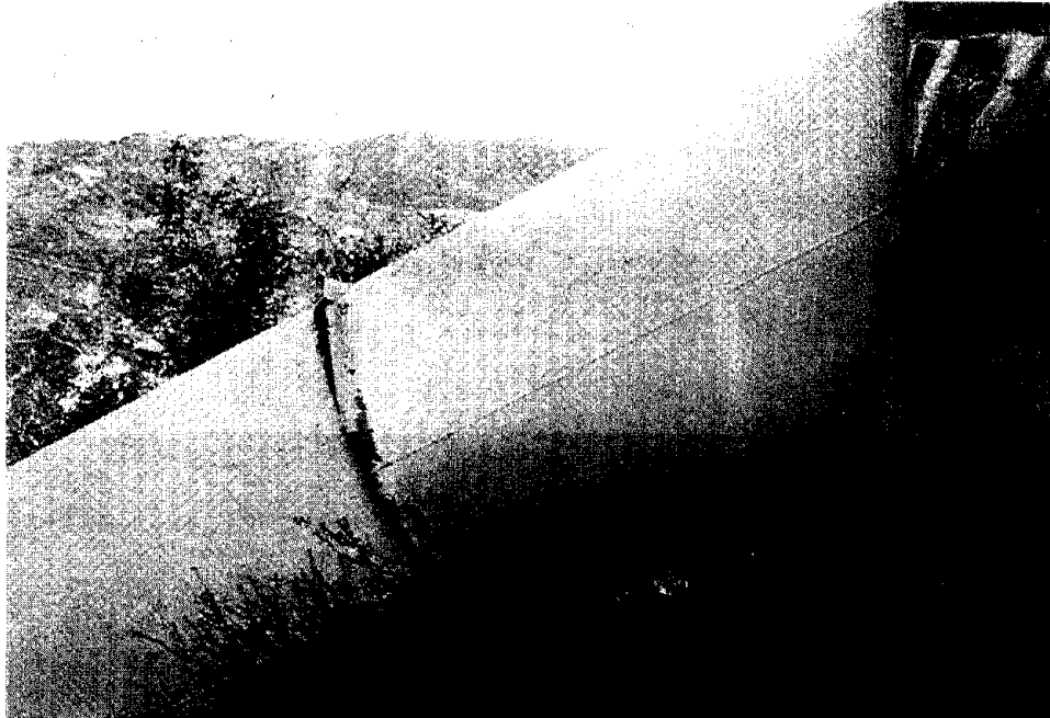
Figure 44 The steel pipeline at Terminal Hill separated from its supporting saddle at several places and pipe sections bulged at other locations along the alignment.
