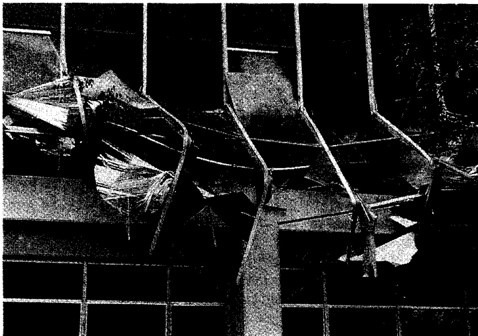
Figure 14 The second story of the concrete frame Kaiser Permanente office building on Balboa Avenue in Northridge completely collapsed. The first story was relatively undamaged, suggesting it was far stiffer than the story above.
