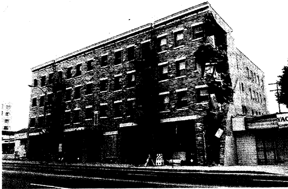
Figure 13 The corner of this rehabilitated unreinforced masonry apartment building in East Hollywood crumbled on all four stories.
