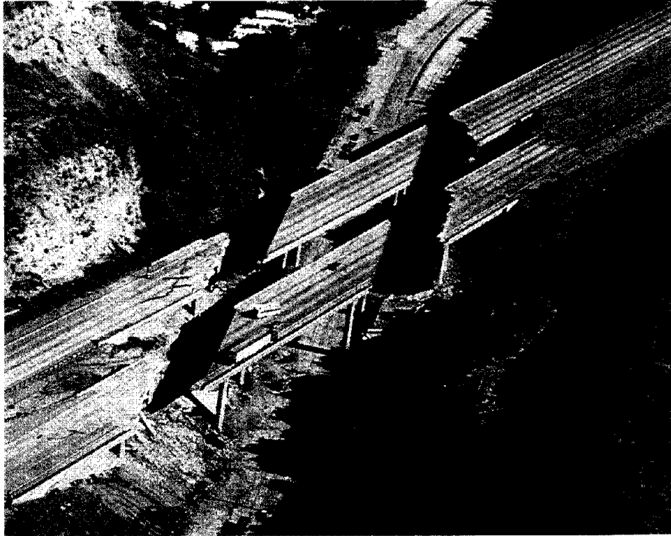
Figure 24 Aerial view of the bridge at Gavin Canyon, looking to the east, showing appearance of the four end spans shortly after demolition had begun
