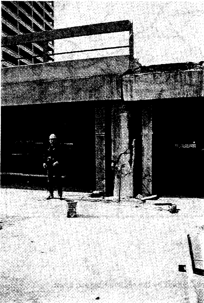
Figure 22 The exterior columns of the Trans World Bank parking garage, which had not been strengthened, were badly damaged.
