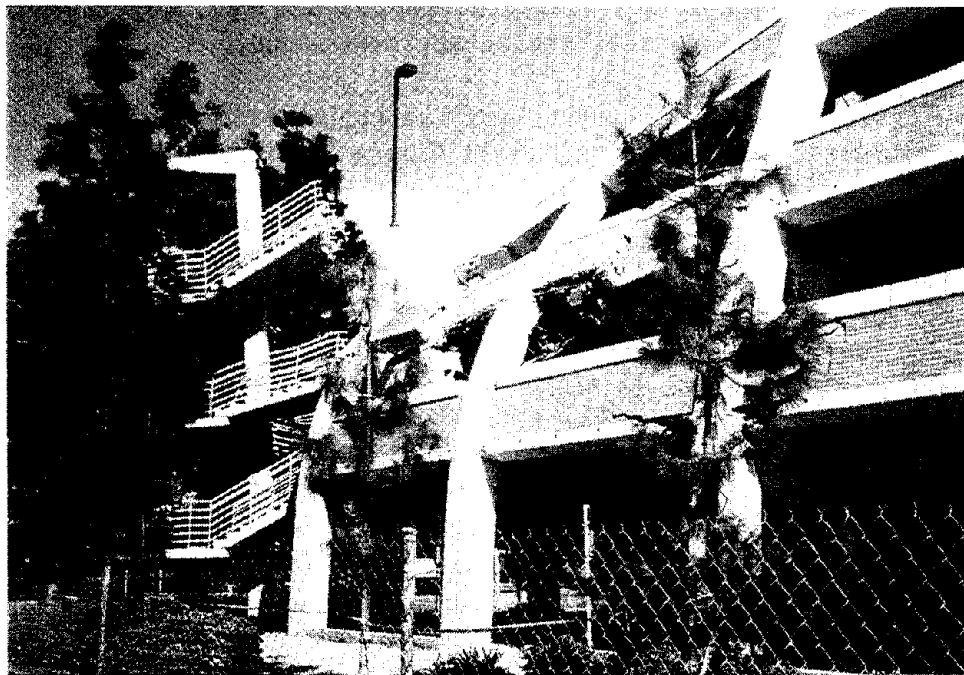
Figure 18 The three-year old four-level parking garage at the Northridge campus of California State University partially collapsed in the earthquake. The collapse apparently started at the interior, causing the exterior walls to be pulled in to the middle of the structure. Precast concrete "trees" were connected to form a moment-resisting frame at the exterior of the structure.
