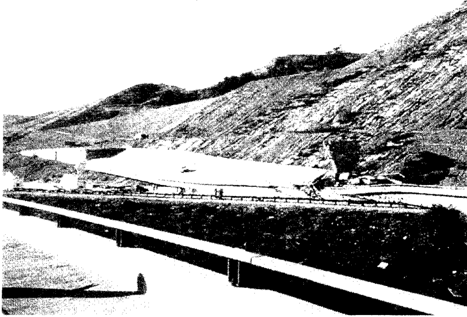
Figure 28 Overview of the collapse of the SR14/I5 Separation and Overhead, Ramp C, looking to the south at Abutment 1. Pier 3 can be seen at the right of the photograph (Courtesy of EERC)
