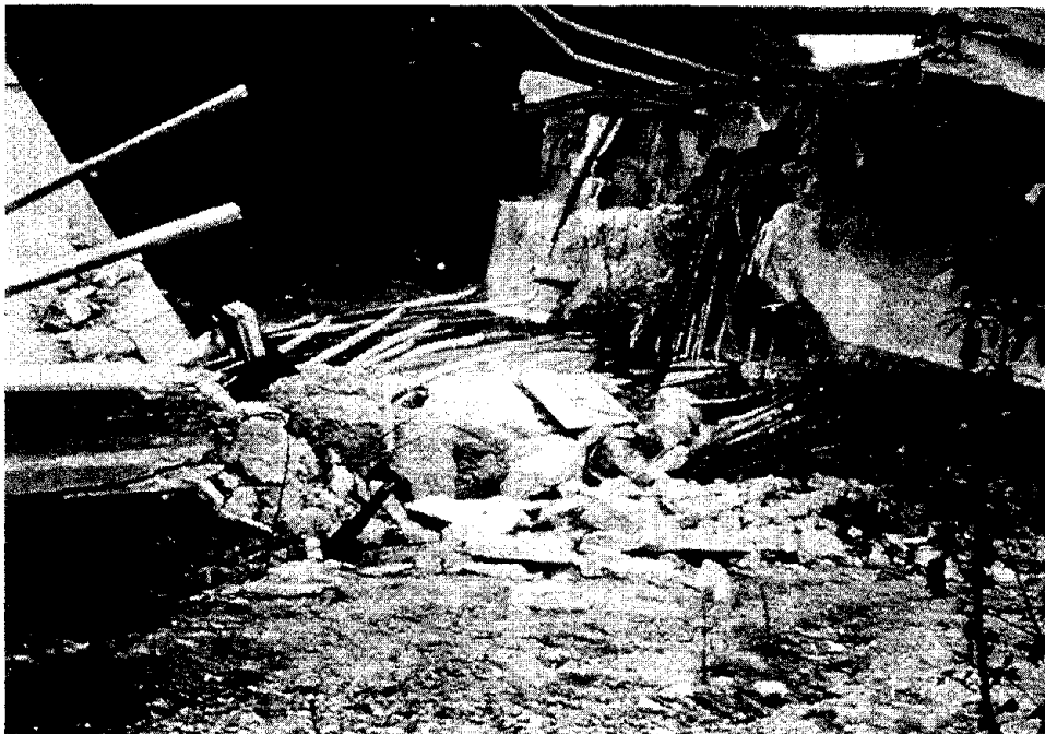
Figure 32 View of crushed Pier 2 and the hinge near Pier 2 (Courtesy EERC)
