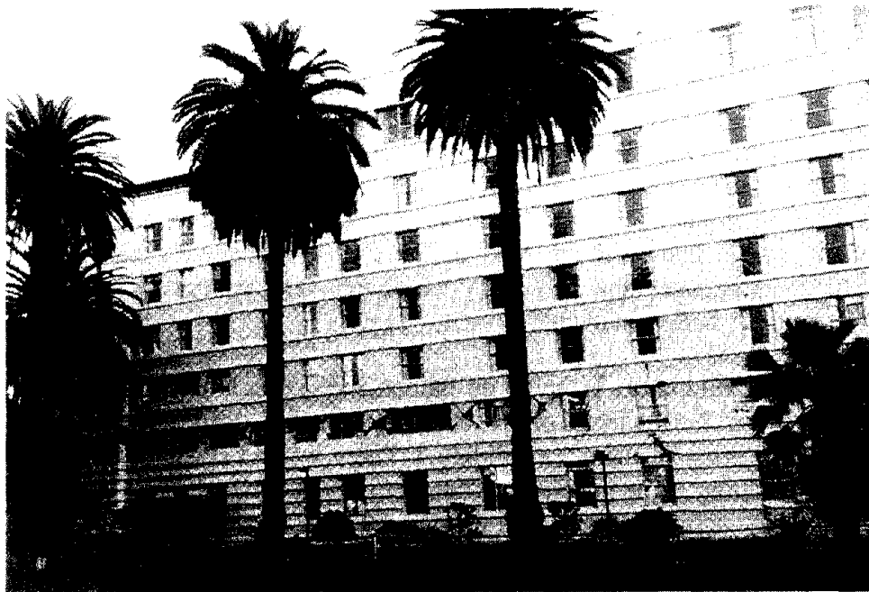
Figure 10 The seven-story northwest wing of St. John's hospital in Santa Monica experienced severe X-cracking in the piers between the second story windows.
