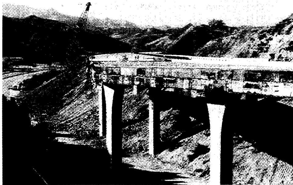
Figure 25 Ground level view of the southbound bridge at Gavin Canyon, looking to the northwest, showing the hinge bearing seat near Bent 3.
