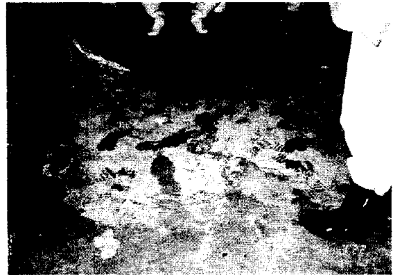
Photo.3 Floor Concrete Spalled Cracks in the Structure between Block 0 and the Connecting Corridor at Pirika Dam (Photograph in the Block 0 Direction from the Connecting Corridor)
