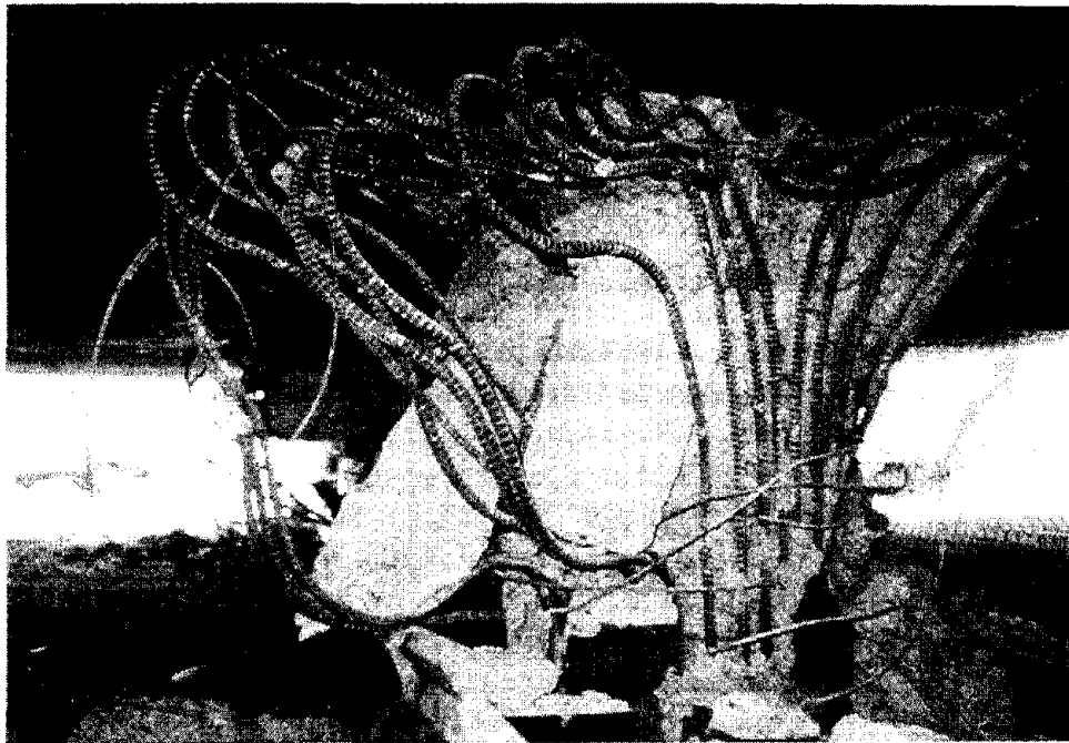
Figure 43. Failed column in Bent 3 of I10 at Fairfax Ave. (Courtesy of EERC)
