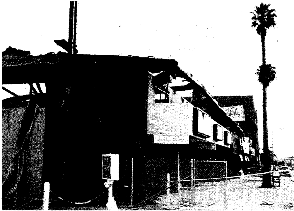
Figure 57 Fire damage in a two story commercial building.
