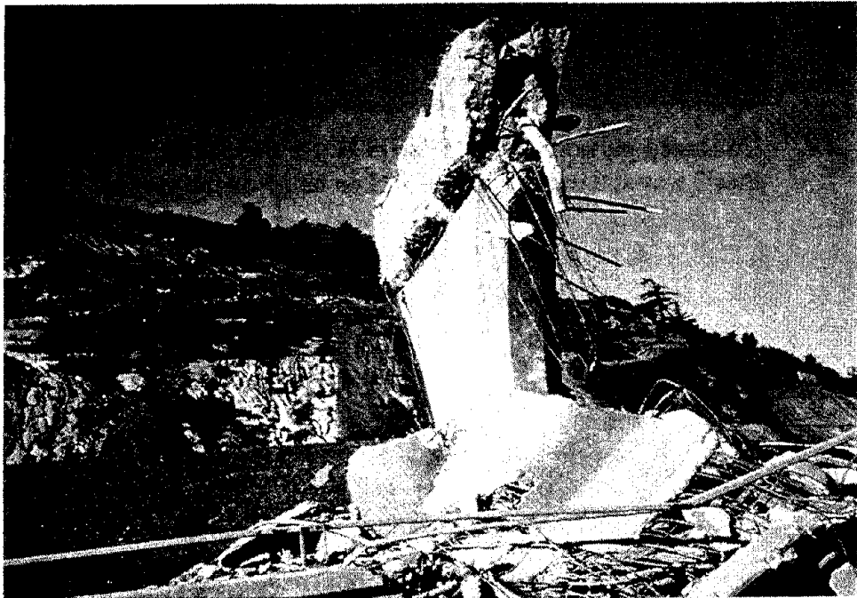
Figure 29 Damage at Pier 3 of the SR14/I5 Separation and Overhead, Ramp C, looking to the west (Courtesy of EERC)
