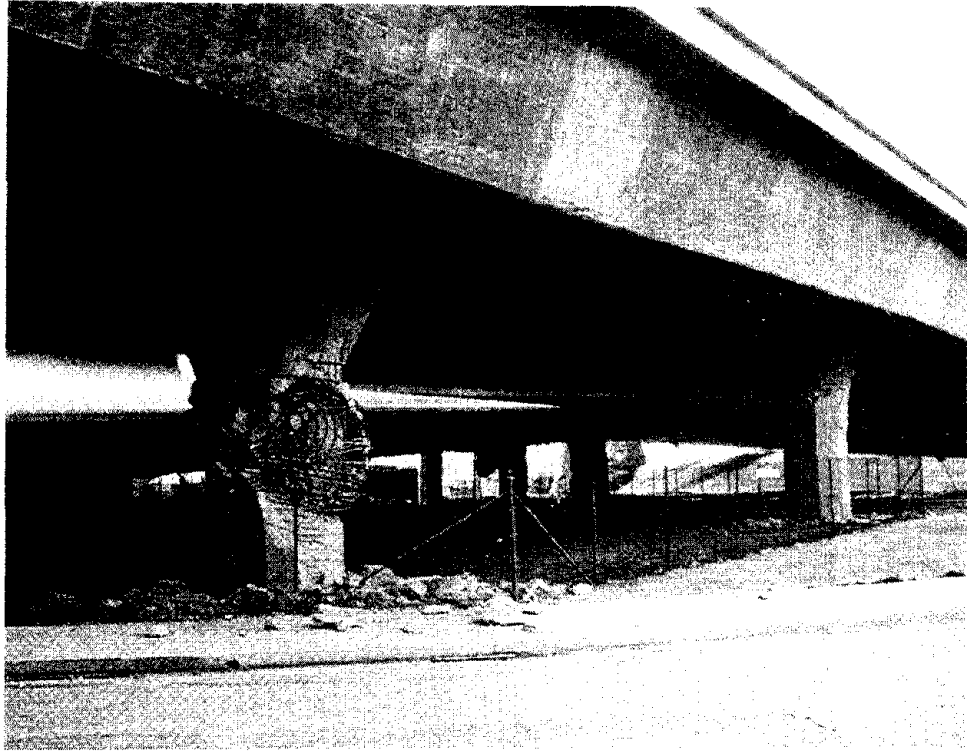
Figure 33. Damage to piers of the SR118 Mission-Gothic Undercrossing, looking to the northwest at the north face of the westbound bridge, Bents 3 (foreground) and 2.
