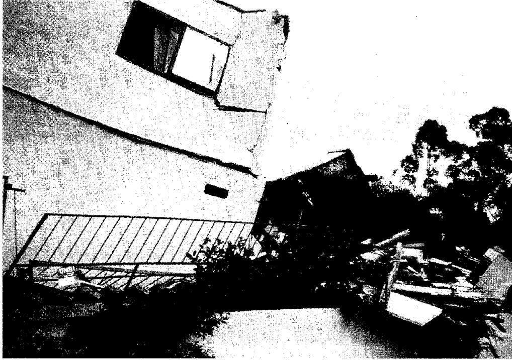
Figure 59 Partially collapsed apartment building with fire damage in the rear.
