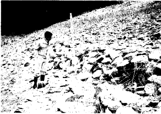
Photo.7 Bulging on the Upstream Slope of the Niwa-Ikumine Dam (Photographed on July 22)
