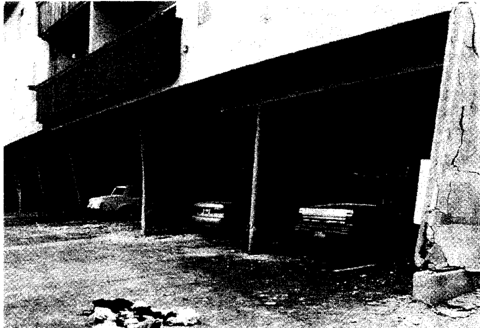
Figure 6 Steel pipe columns between parking bays supported the upper stories of the Northridge Meadows apartment buildings. Few of the buildings in the north half of the complex collapsed, but all were damaged.
