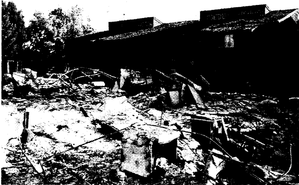
Figure 61 Multi-family residential building destroyed by fire.
