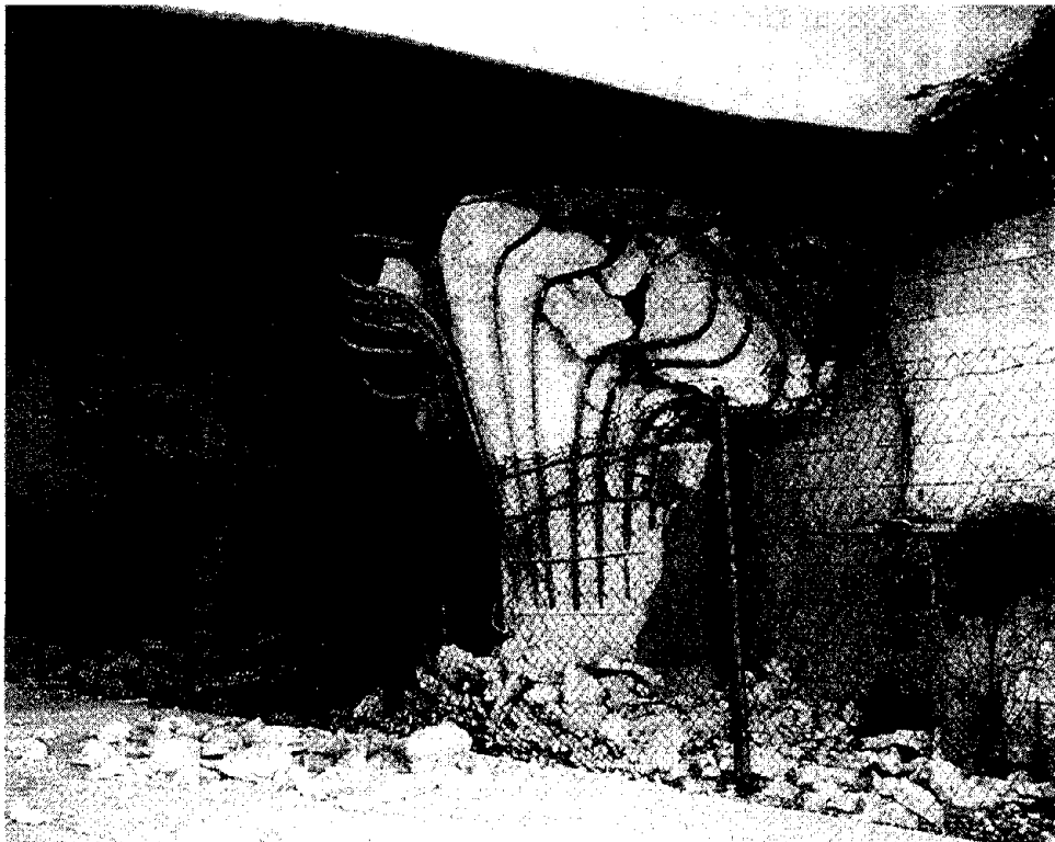
Figure 40 Piers of Bent 3 supporting eastbound lane of I10 at La Cienega Blvd.
