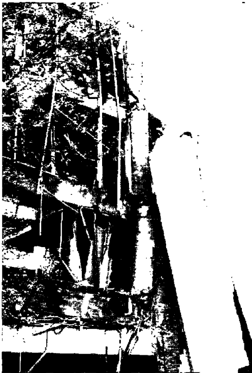
Fig. 6.3 Nonductile Reinforce Concrete (RC) Frame with Soft Story Mechanism
