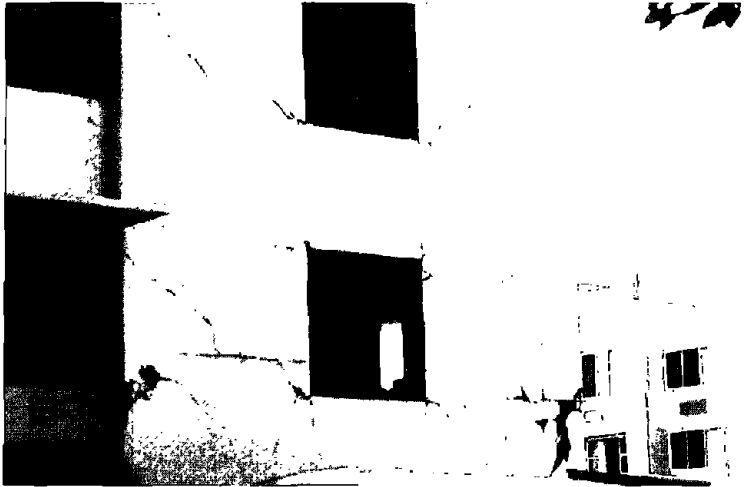
Fig. 6.5 Damage to Shear Wall of Dual Frame-Wall System
