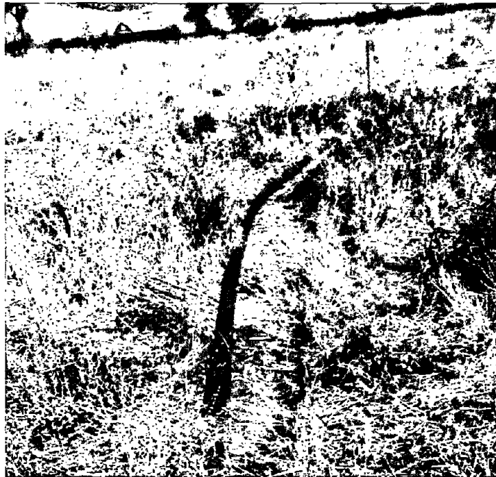
Fig. 4.3: Evidence of localized compression in Potrero Canyon. Note that originally straight pipe was pushed up and laterally; shortening across its length was 5 inches.
