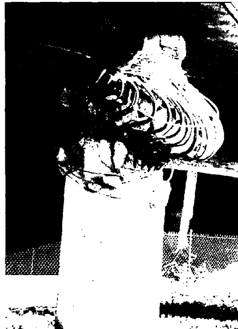
Fig. 5.9: Column Failure at Bent 2, Bull Creek Canyon Channel Bridge
