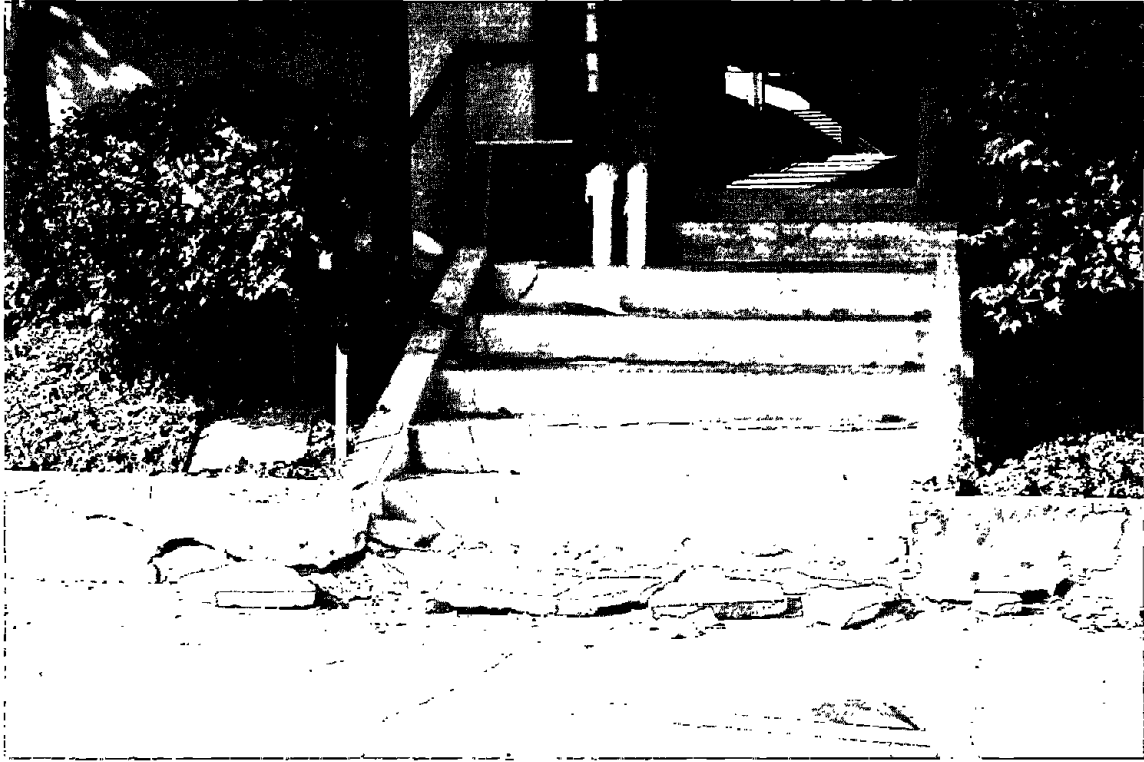
Fig. 4.7: Damage from lateral spreading, Northridge Hospital
