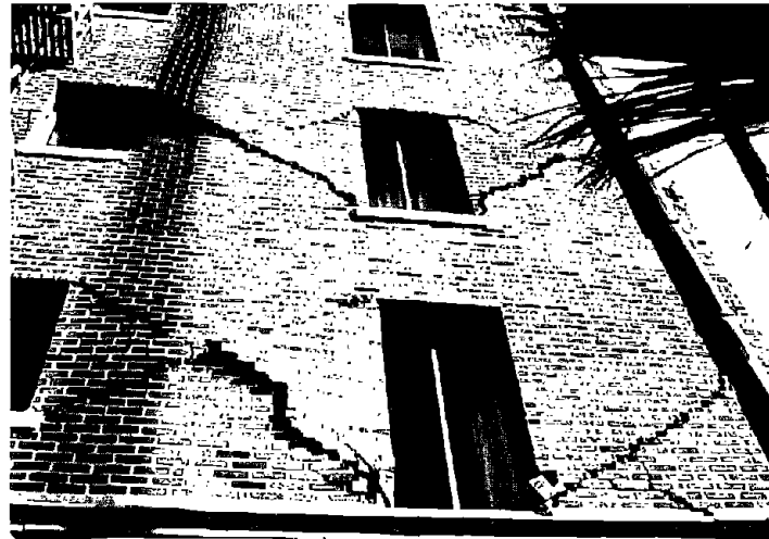
Fig. 6.14 Shear Cracking in Non-Bearing Masonry Wall
