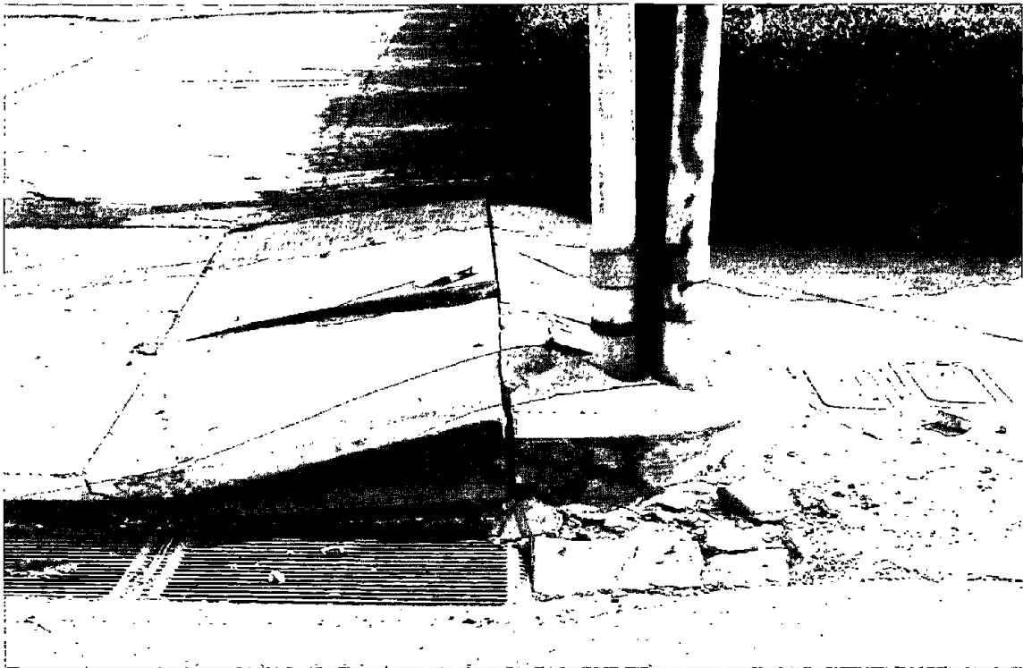
Fig. 4.8: Buckling of curb from lateral spreading, Northridge Hospital
