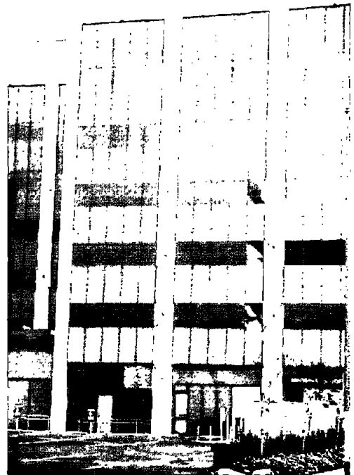
Fig. 6.4 Short Column Behavior in 6-story RC Moment Resisting Frame
