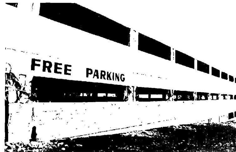
Fig. 6.8 Short Column Effect due to Partial Infill
