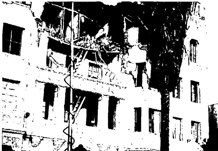
Fig. 6.15 Typical Shear and Out-of-Plane URM Failure
