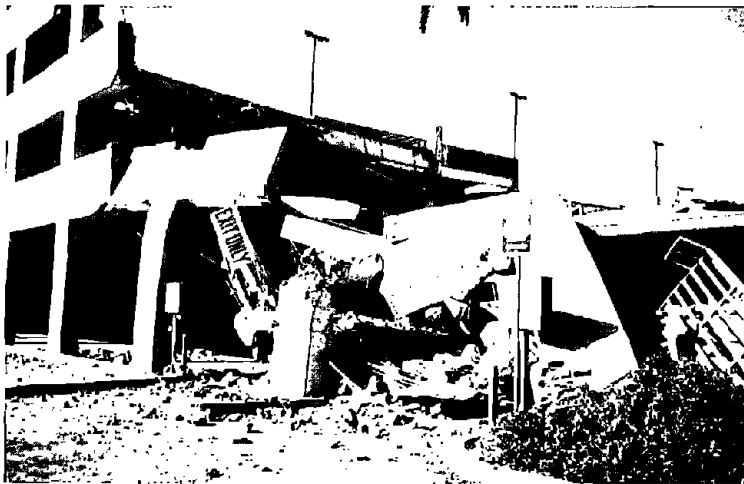
Fig. 6.7 Characteristic "Implosion" of Precast Parking Structure
