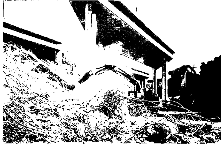
Fig. 5.19: Collapsed Spans at Gavin Canyon Undercrossing
