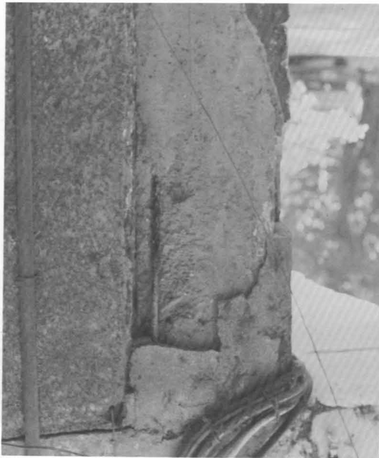
Figure 6: Crushing of Reinforced Concrete Corner Columns of a Seven Story Reinforced Concrete Frame Building with Infilled Walls
