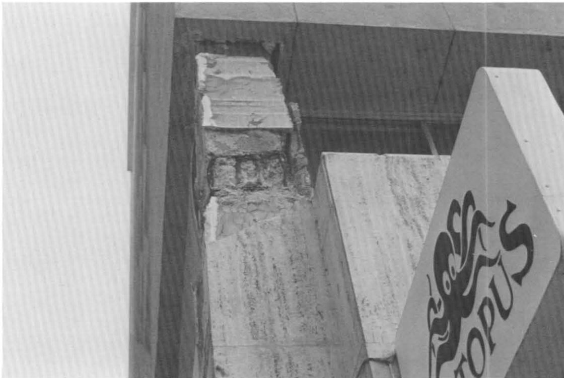
Figure 8: Crushing of Reinforced Concrete Corner Columns
