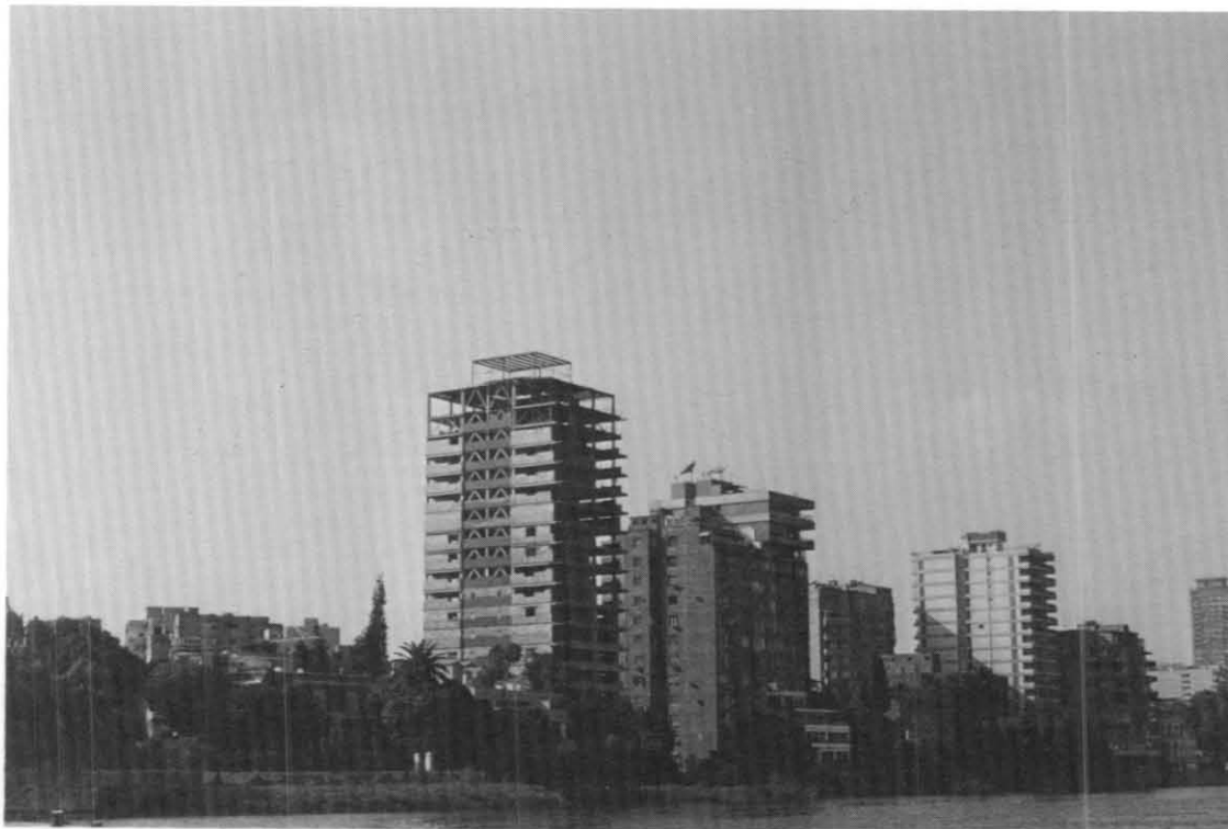
Figure 4: Reinforced Concrete High-Rise Building with Masonry Infilled Walls had Little or No Damage
