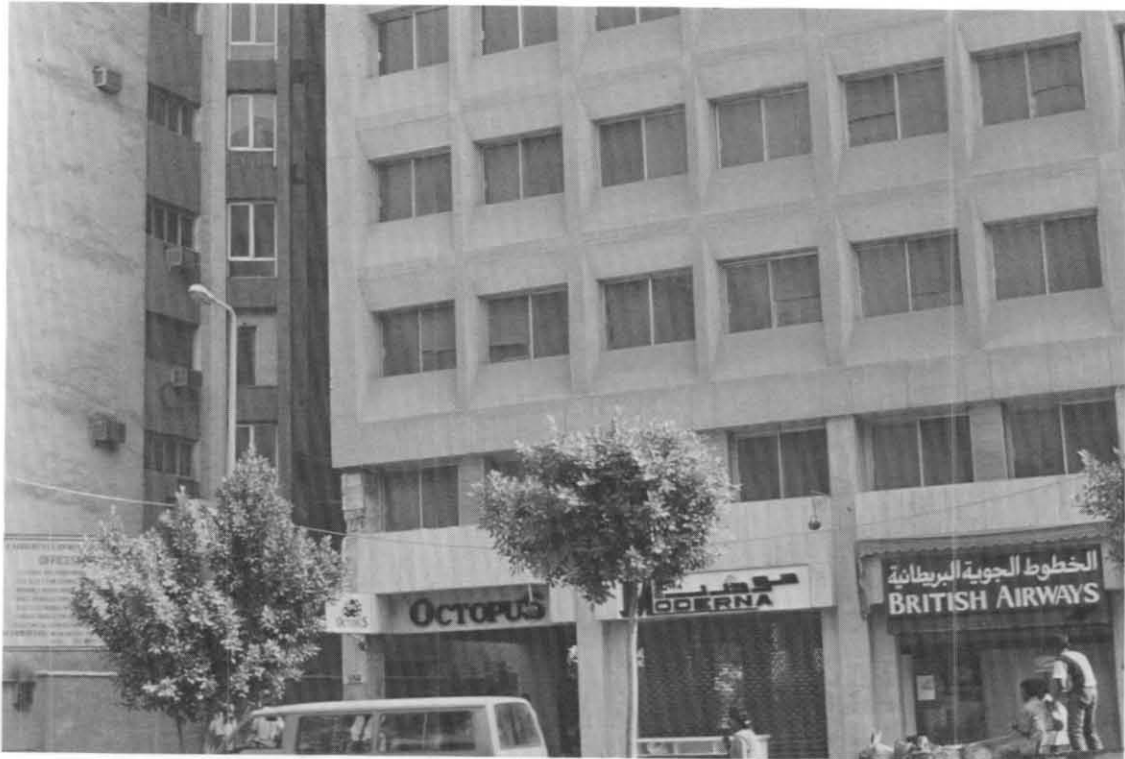
Figure 7: Twenty-two Stories Reinforced Concrete Building with Infilled Masonry Walls Suffered Crushing of Corner Columns
