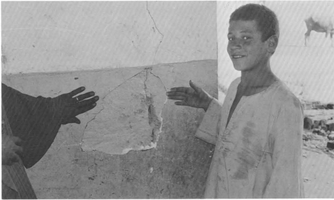
Figure 5: Infilled Masonry Walls Prevented Severe Damage to the Two Story School Near the Epicenter
