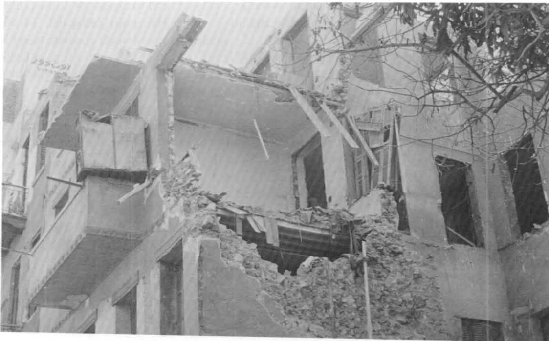
Figure 1: Collapse of Buildings in Cairo
