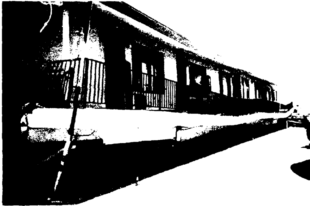
FIGURE 3-18 Wood Frame Apartment with Collapsed Carport on Reseda Boulevard in Northridge
