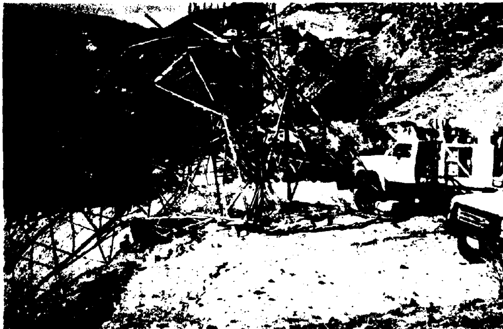
FIGURE 4-15 Several Electrical Transmission Towers Failed During the Earthquake - Foundation Distress was Observed at Most of the Failed Towers
