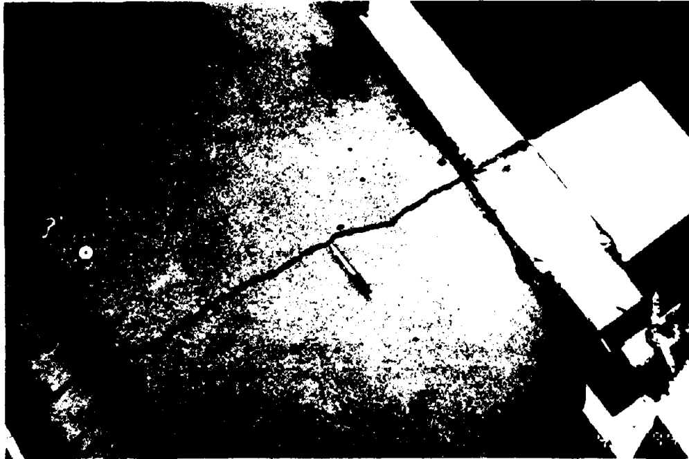
FIGURE 4-12 Typical Cracks (up to 1/2 Inch Wide) in Concrete Basins in the 15-mgd Wastewater Treatment Plant in the Santa Clarita Valley
