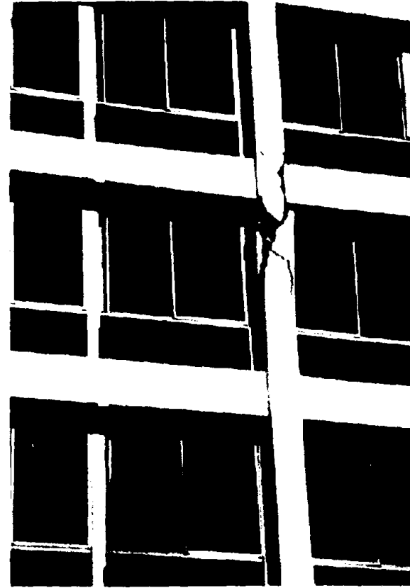
FIGURE 3-25 Damaged Columns in Seven-Story Hotel in Van Nuys
