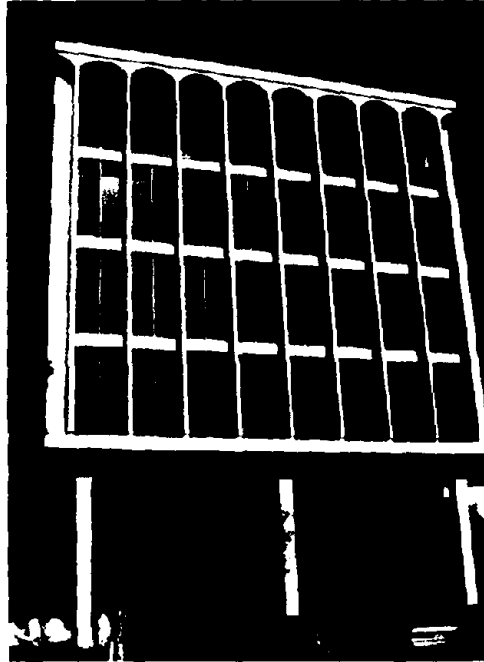
FIGURE 3-36 Five-Story Office Building Near Epicenter
