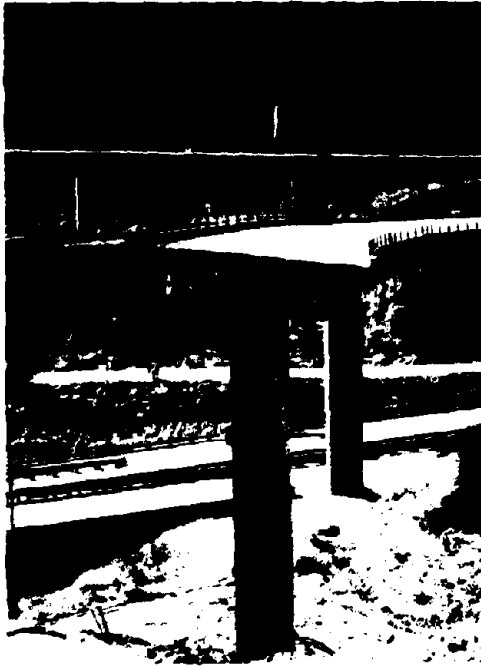
FIGURE 3-6 SR14/I-5 North Connector - Collapsed End Spans After Demolition
