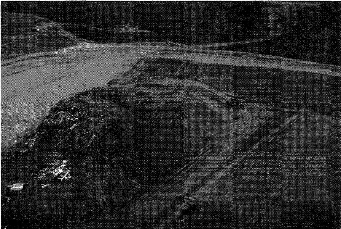
Fig. 6.77: Waste placement operations in Cell C, four days after the Northridge Earthquake
