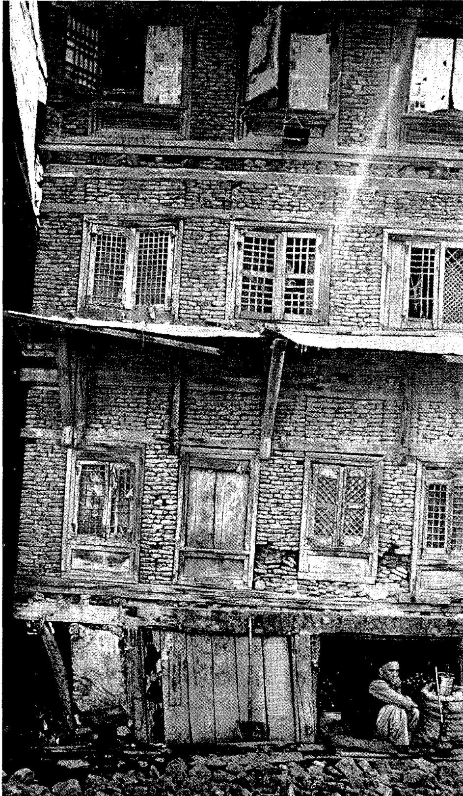
FIGURE 2: A BUILDING IN SRINAGAR, KASHMIR WHICH HAS SURVIVED MANY EARTHQUAKES BECAUSE OF ITS TIMBER RUNNER BEAMS. The ends of the floor joists can be seen penetrating the wall between the horizontal beams. There are no vertical supports in the masonry wall.
