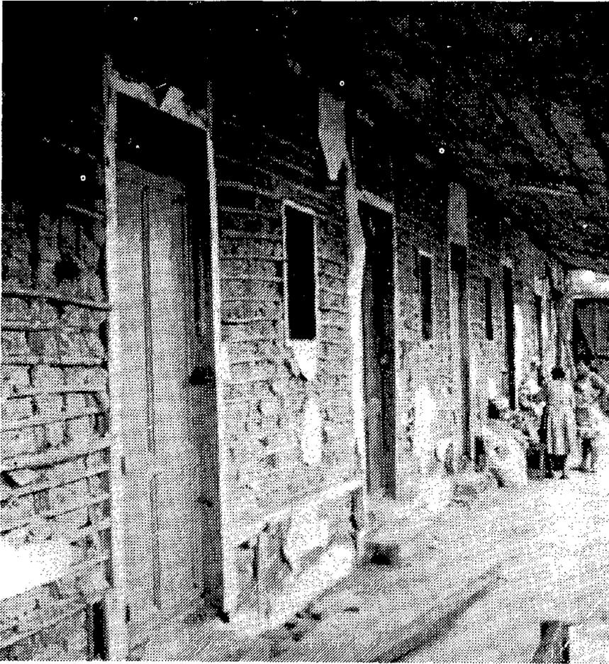
FIGURE 3: BAHAREQUE CONSTRUCTION IN EL SALVADOR AFTER THE 1986 EARTHQUAKE. The racking from the earthquake caused all of the stucco to fall off, but left the building standing.
