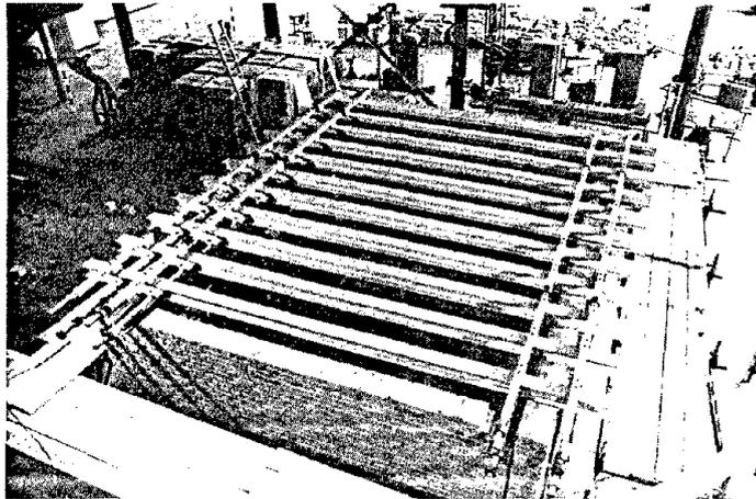
Fig. 4. View of the floor beams during construction. The longitudinal bars used to distribute the horizontal forces to the floor beams are visible
