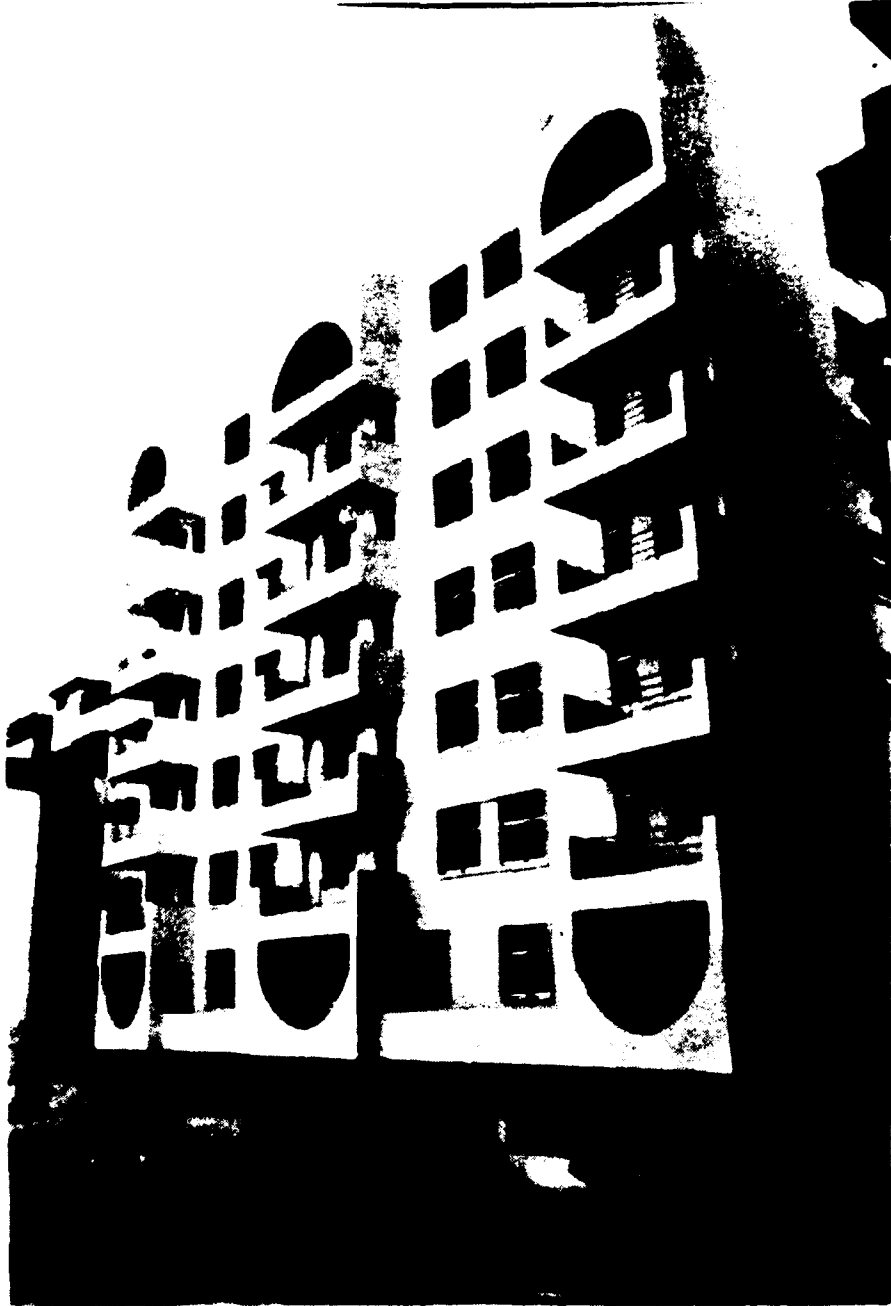
Figure 3: Photograph of Shantou Demonstration Building
