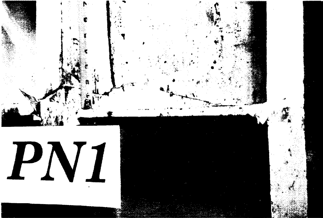
Figure 3-18. Cracks in Column Flange and Web
