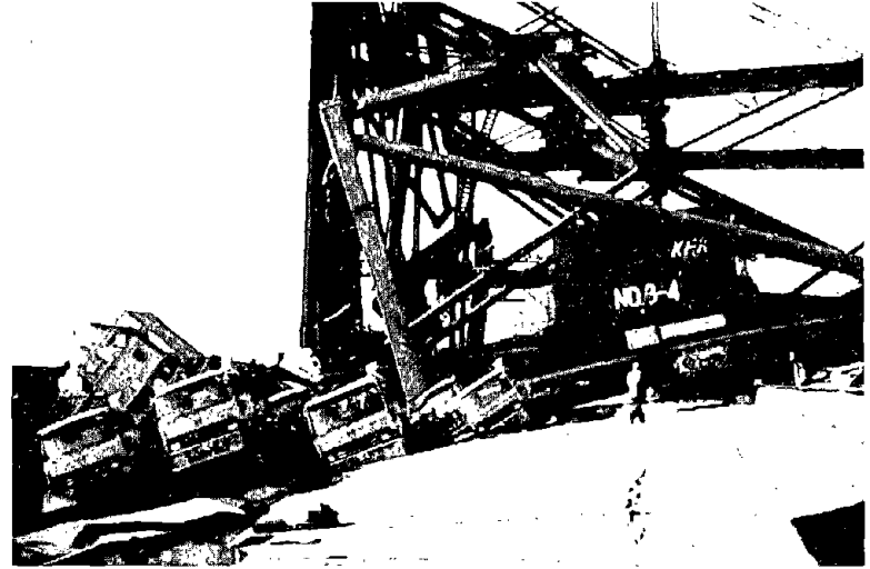
Figure 3.17: Collapse of crane due to lateral movement (~2 m) of quay wall on Rokko Island. Note settlement of 1-2 m also occurred behind wall.
