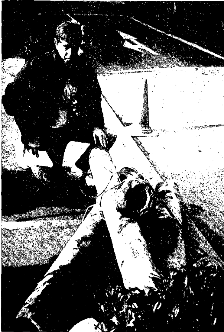
Figure 6.23: Rupture of 6 KV electric cable conduit in Kobe City. (Dr. T. Holzer in photo).
