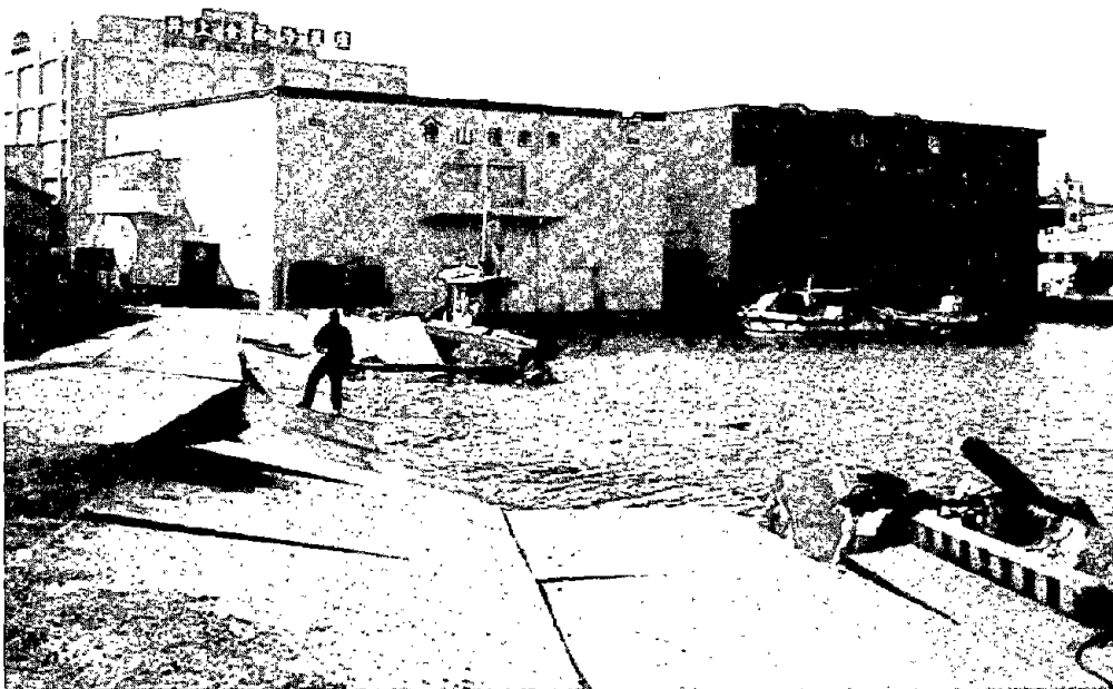
Figure 3.25: Damaged quay wall on west side of Tsukiji-cho.
