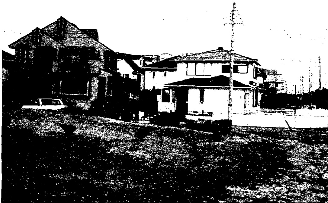
Figure 3.3: Relatively undamaged houses in a residential area in Ashiya. Note the evidence of lateral spreading caused by the liquefaction of the fill.
