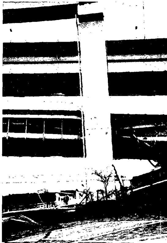
Figure 3.56: Tilting of support on Rokko Island causeway (~40 cm at top) led to drop of girder.
