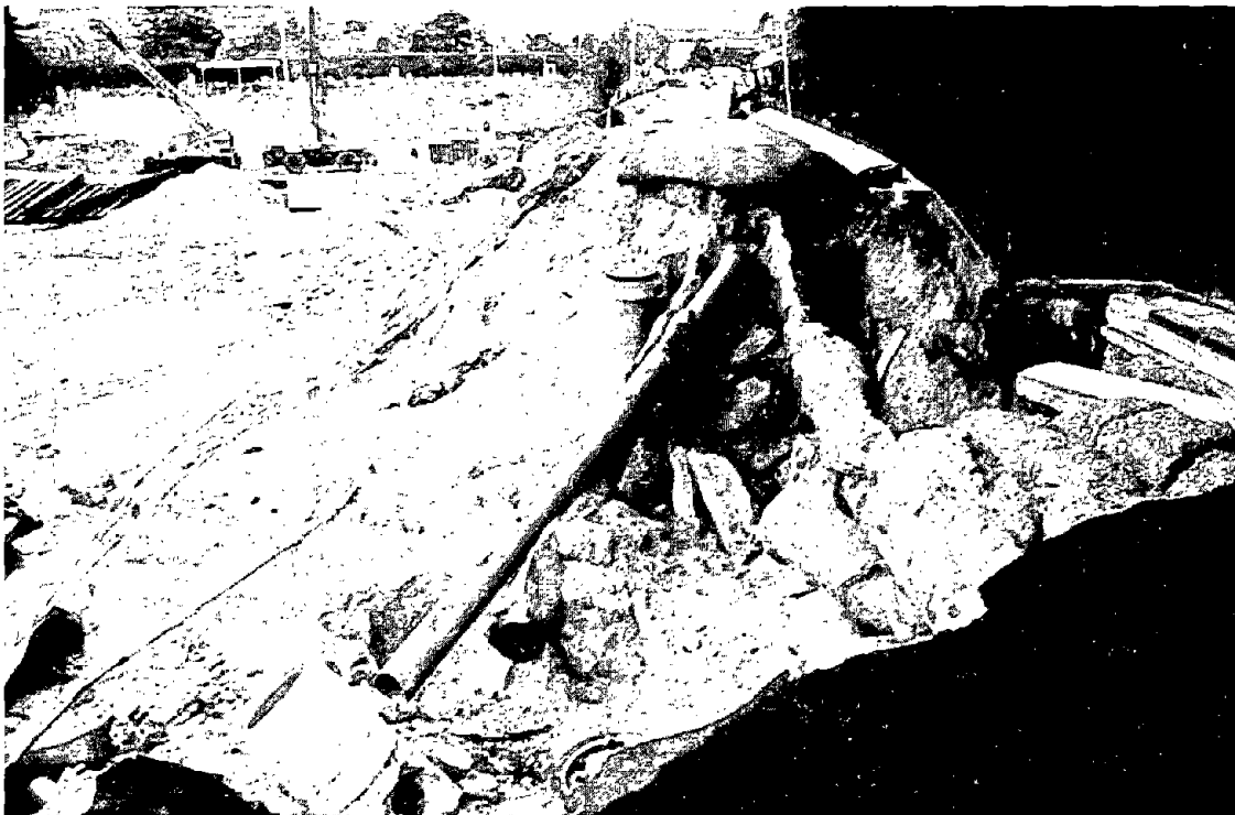
Figure 5.8: Failed perimeter roadway fill along Upper Niteko Reservoir.
