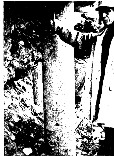
Figure 3.64: Excavated upper part of pile foundation beneath the tank shown in Figure 3.61.
