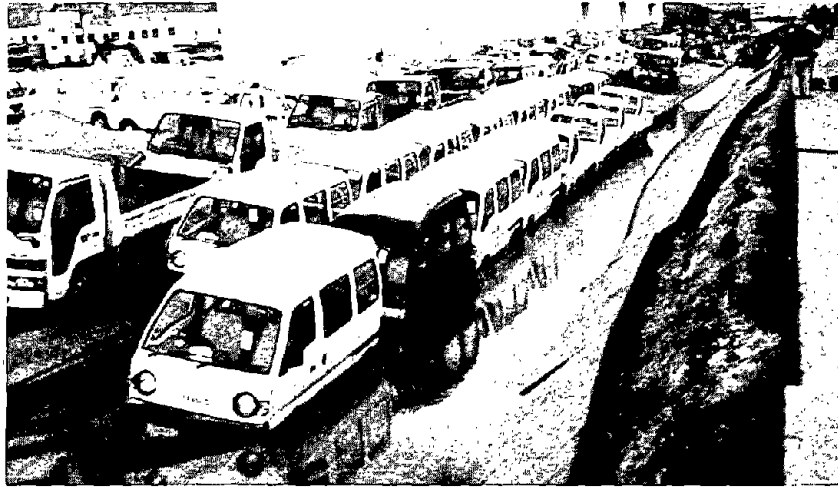
Figure 3.19: Vans and trucks ready for shipment before earthquake. Lateral spreading caused 1.5 m-2 m drop of paved surface and local flooding.
