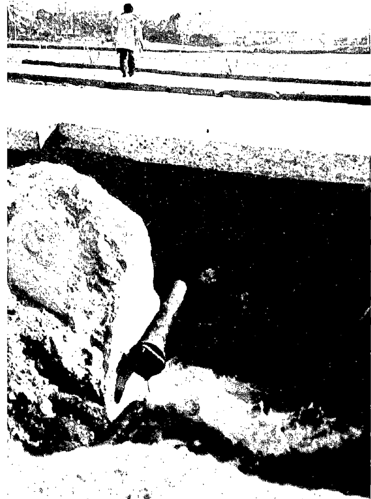
Figure 6.24: Rupture of electric conduit caused by seawall deformation adjacent to north side of Kobe Port Island Bridge.
