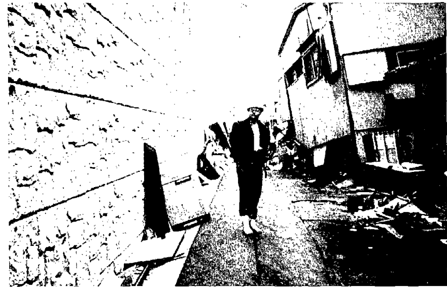
Figure 7.17: Post-earthquake view of the Tanata GRS-RW wall.
