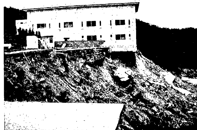
Figure 7.4: Head scarp of the Nigawa landslide. The stratification of soil below the pavement suggests that this upper material is fill. The foundation of the building is pile supported.
