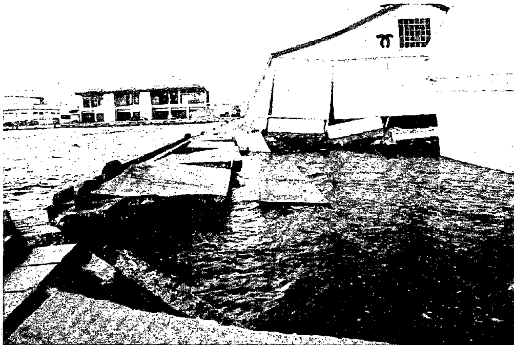
Figure 3.23: Damage to the end of Hyogo Pier No. 2.
