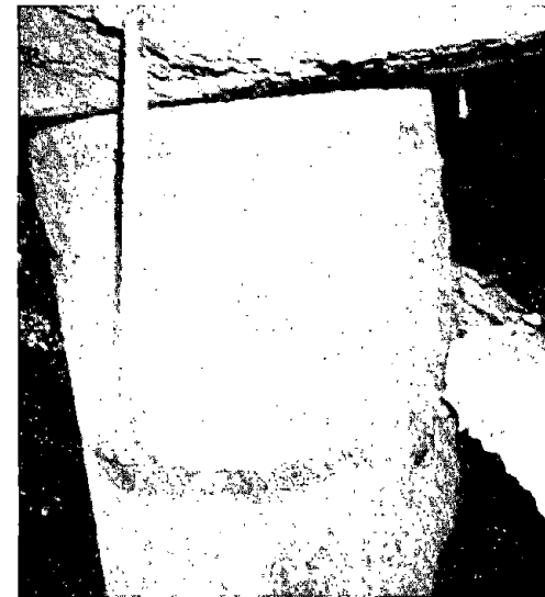
Figure 3.50: Shaft (0.5 m diameter) beneath larger ferry building was undamaged by liquefaction induced ground settlement and lateral spread.
