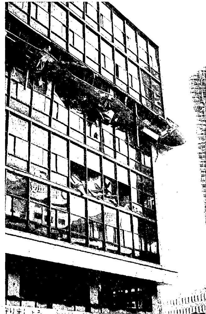
Figure 2.17: Building in central Kobe with mid-height story collapse in the fault-normal direction.
