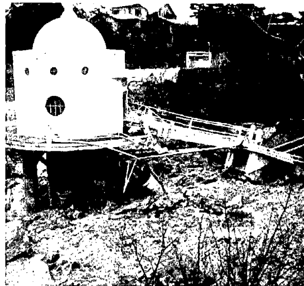
Figure 5.6: Downstream outlet tower at Upper Niteko Dam.
