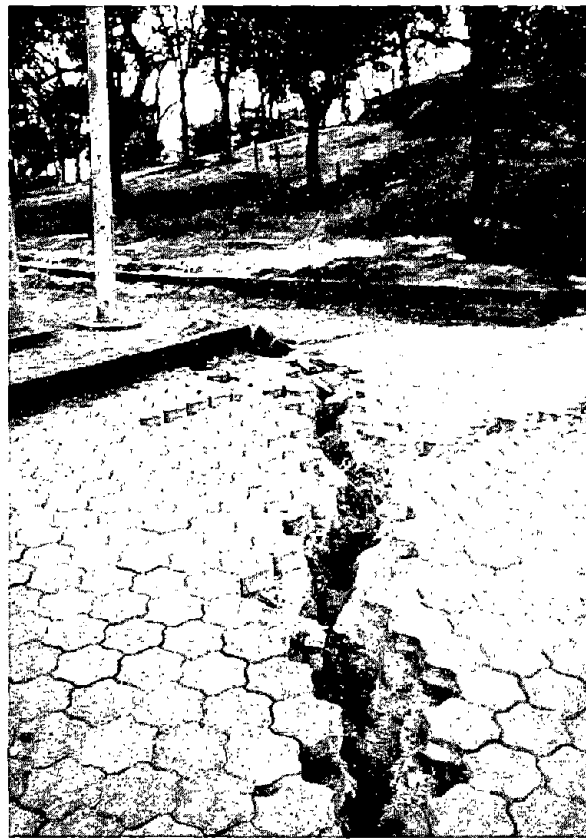
Figure 3.74: Fissures in Osakako park indicative of liquefaction, differential ground settlement, and lateral spread.
