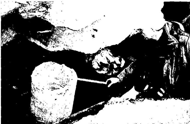
Figure 3.46: Sheared and translated hollow-tube pile which had little lateral resistance. Pile had supported warehouse building shown in Figure 3.44.
