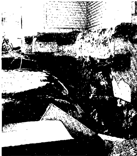
Figure 3.49: Lateral spread and graben exposed foundation walls and supporting shafts beneath the larger ferry terminal building (see Figure 3.48).
