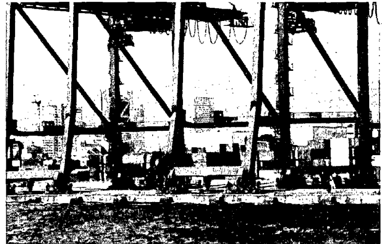
Figure 3.18: Buckled or plastically yielded crane legs due to about 2 m of spreading between crane rails as a consequence of lateral caisson displacement.
