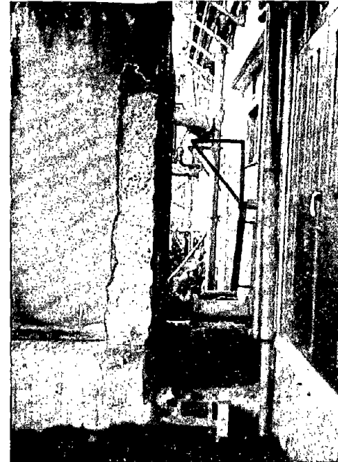
Figure 6.14: Severe lateral displacement at the inverted siphon of the plant. The pressurized pipeline siphon carried all sewage treated by the plant.
