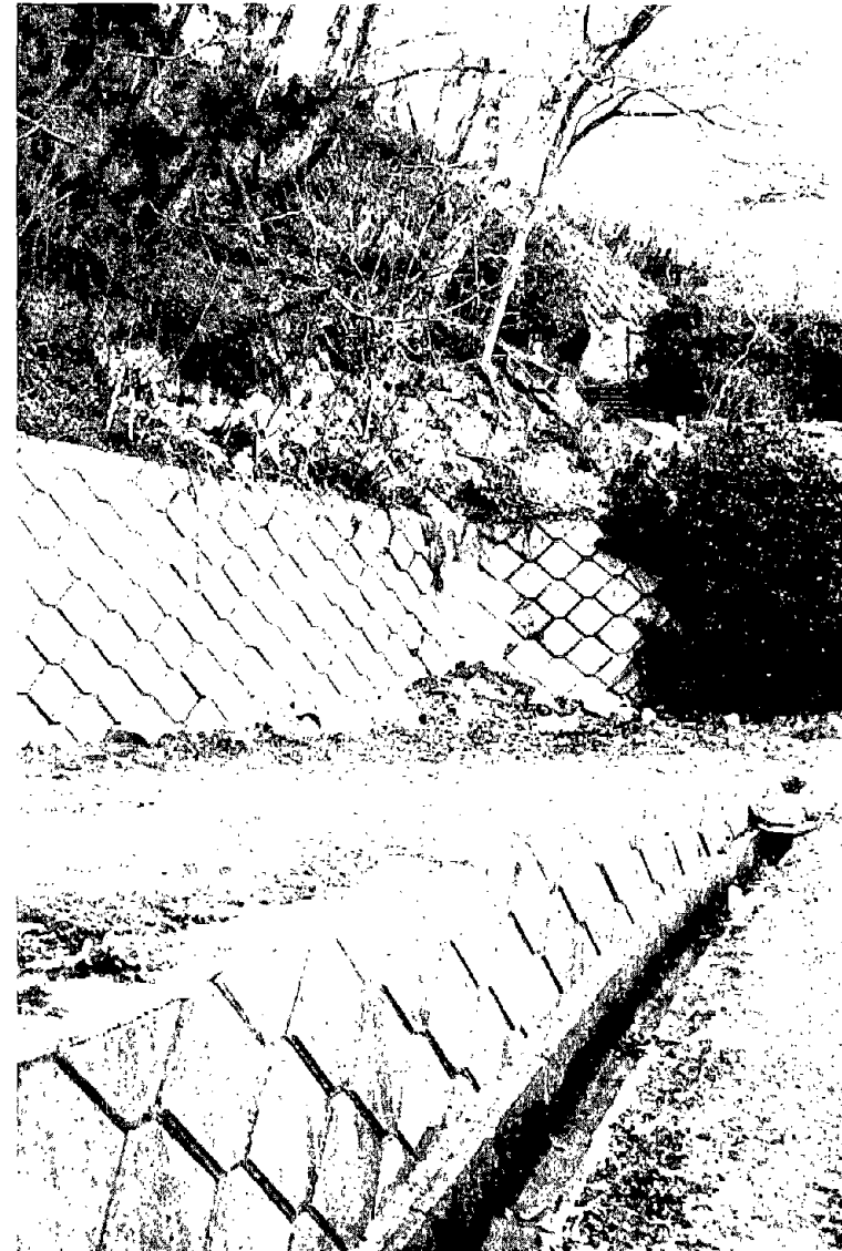
Figure 7.7: Freshly fallen rock at the base of a retaining wall in a residential area.
