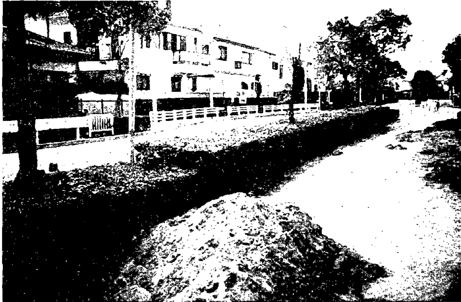
Figure 3.53: Modern Japanese houses in Ashiya constructed with wood studs and plywood sheathing similar to many U.S. single-unit houses. Liquefaction and ground oscillation occurred beneath area. Piles of sand in roadway are from residents clearing sand boil deposits from their gardens. The only damage noted in this area was slight tilting of a few houses.
