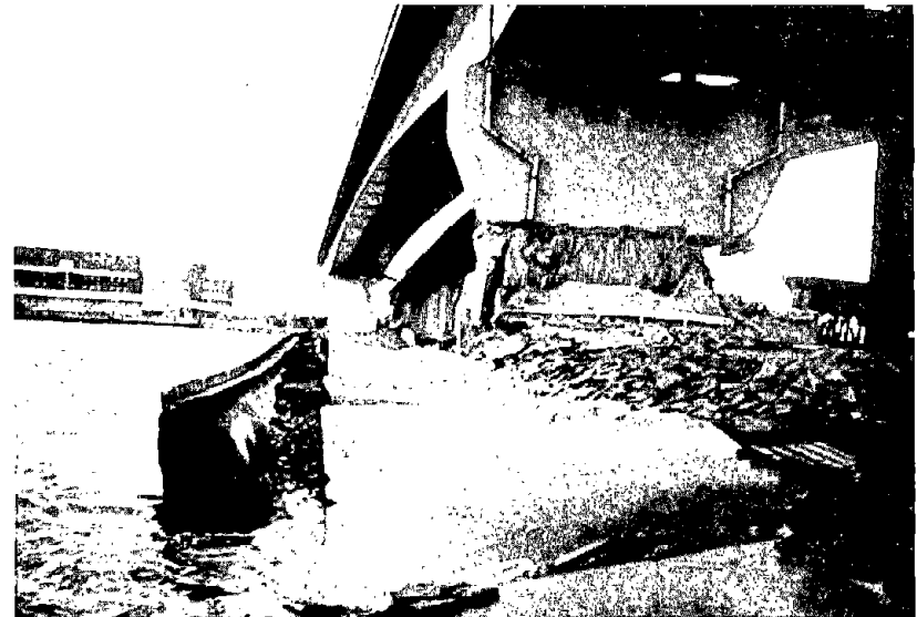
Figure 3.34: East bank of Maya-ohashi bridge: south side.
