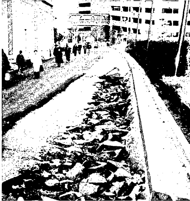
Figure 3.51: Lateral spreading on north side of Harborland ferry terminal.
