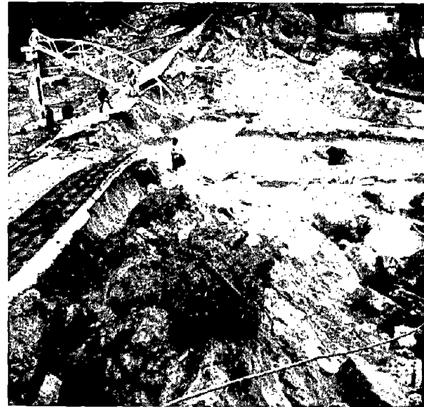
Figure 5.5: Crest alignment of failed Middle Niteko Dam.
