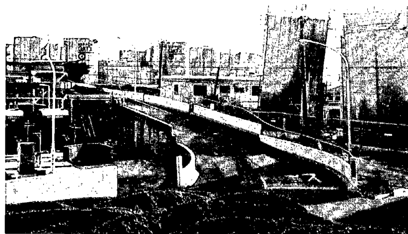
Figure 3.70: Listing tanks in the Nippon Gatx complex.
