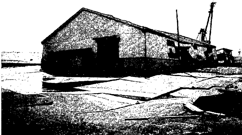
Figure 3.21: Damage to the end of Hyogo Pier No. 1
