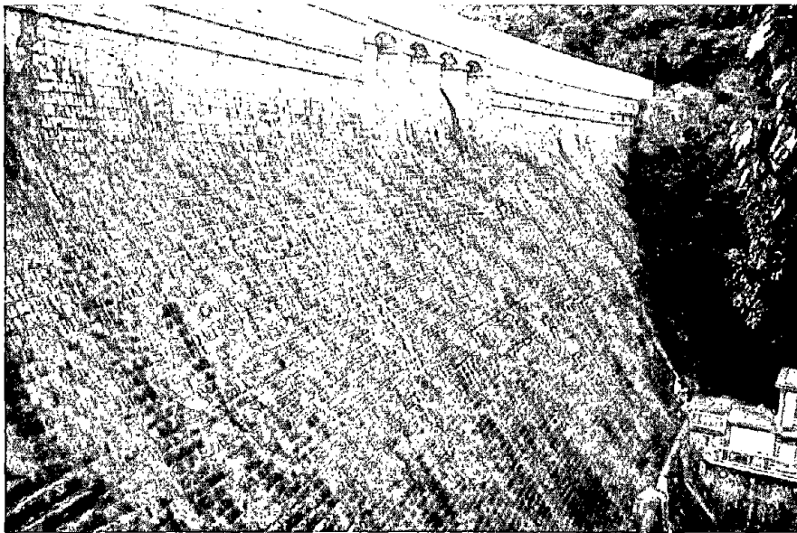
Figure 5.14: Downstream face of Karasuhara Dam.
