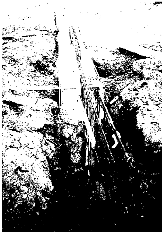
Figure 3.54: Foundation under construction for house in Kobe area. Note that perimeter and interior wall footings are well reinforced and tied together. Foundations of this type allowed houses in areas affected by liquefaction to survive the earthquake with no damage except for slight tilting of a few units.
