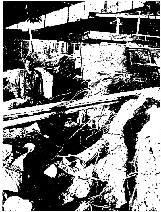
Figure 4.18: Large ground crack outside the southwest corner of Warehouse #21.
