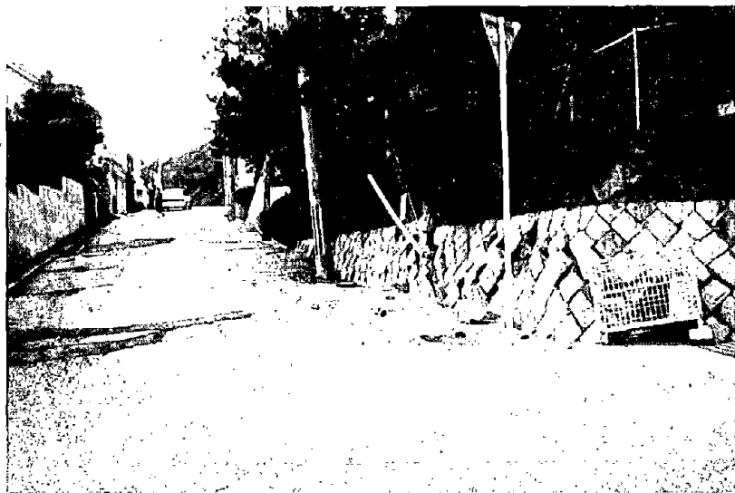
Figure 7.9: Pavement deformation and damage to rock retaining wall caused by seismically induced deformation of sidehill fill.
