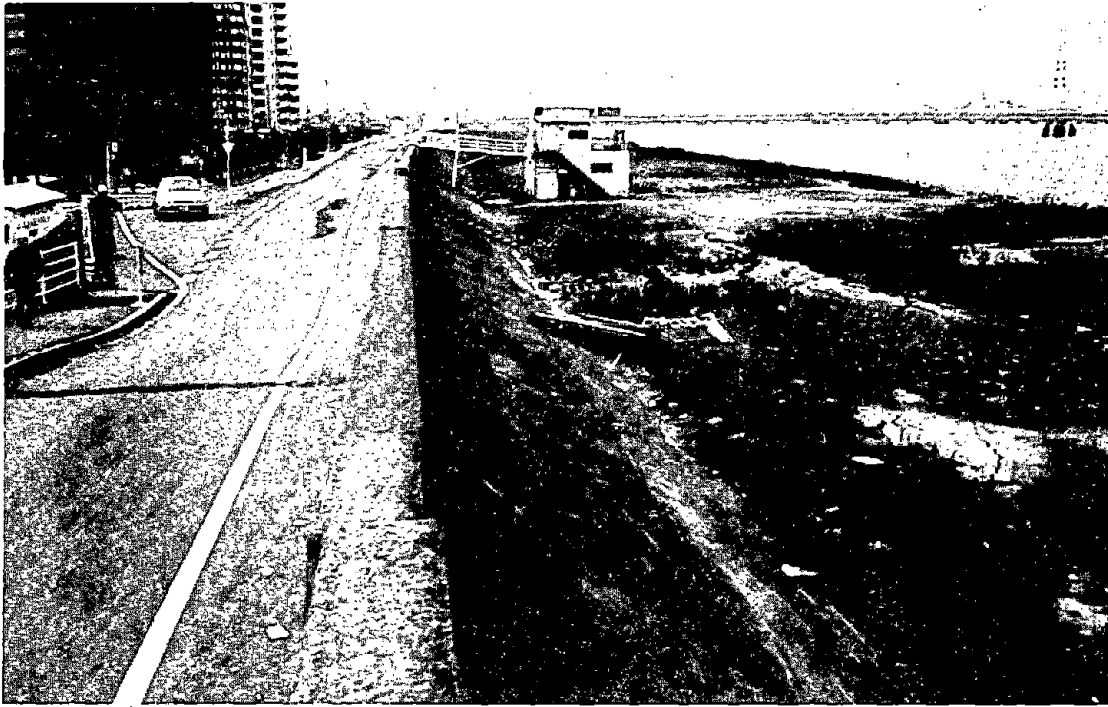
Figure 5.20: Moderately damaged Yodo River levee (note sand boils on exposed waterside foundation).
