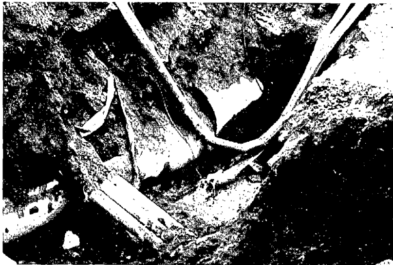
Figure 6.11: Weld rupture of 700-mm-diameter steel water trunk main on Port Island.
