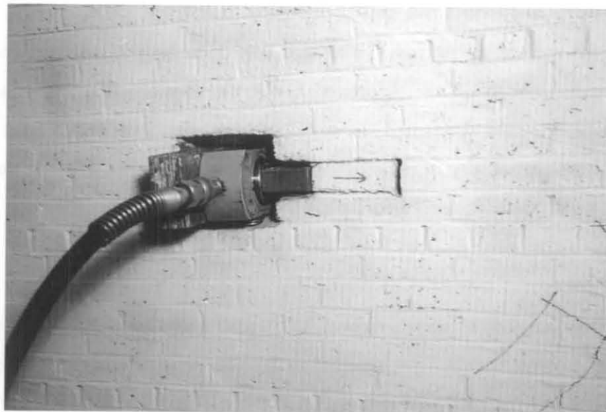
Figure 2.24c Typical Reduced-scale Shove Test
