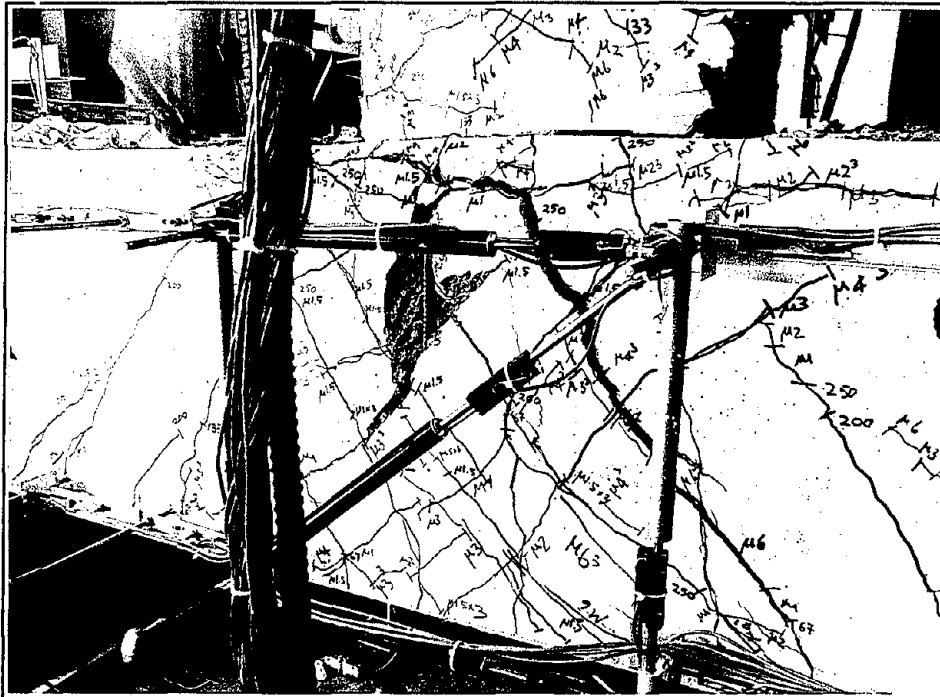
Figure 4.12 Damage on the east face of the joint at \mu_{\Delta} = -6 \times 3 . Note that the damage on the west face appeared less severe.
