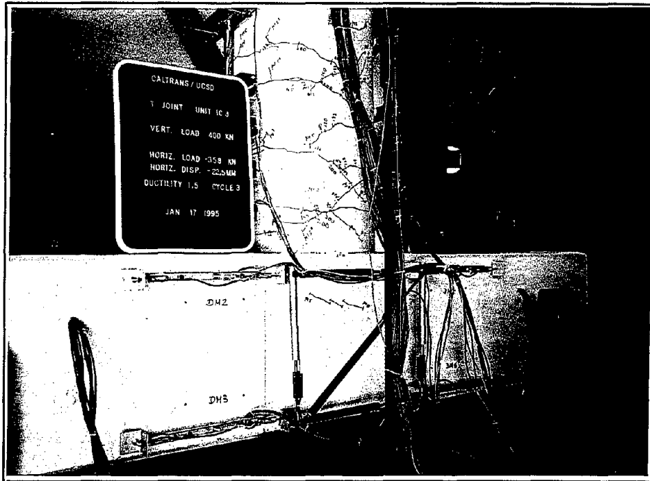
(c) Cracking on the east face of the joint region
