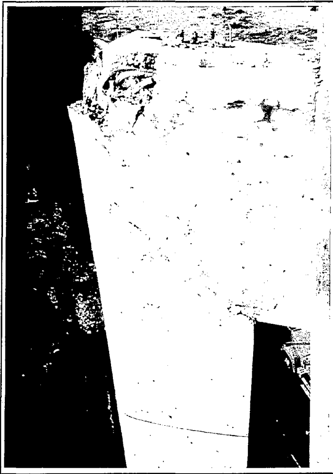
(a) Damage to outrigger knee joint of I-980 Bent #38 in the Loma Prieta earthquake.
