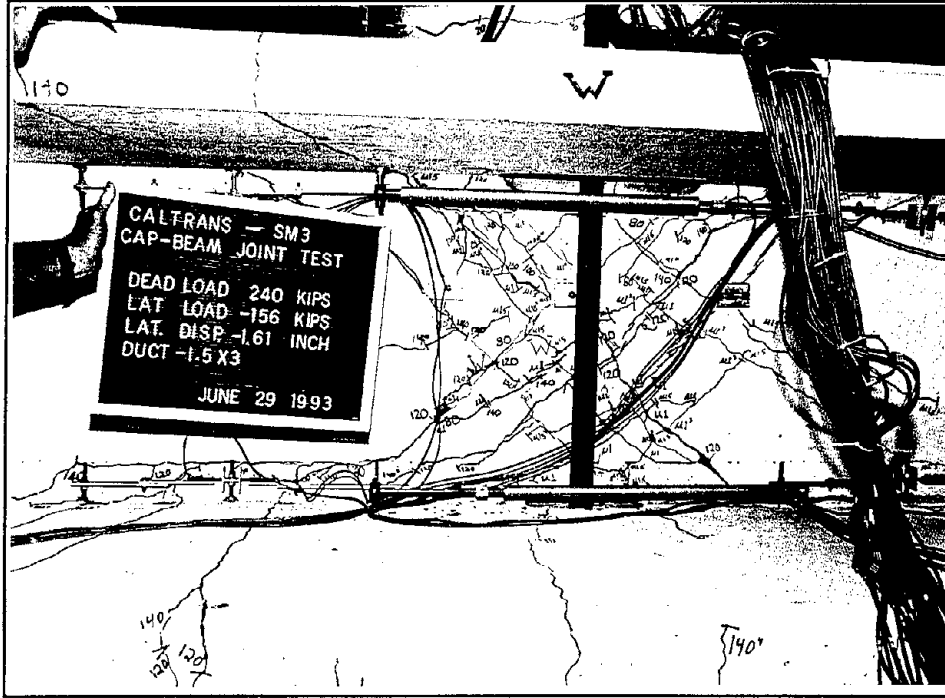
Figure 3.13 SM3 joint shear cracks on west side at \mu_{\Delta} = -1.5 \times 3 .
