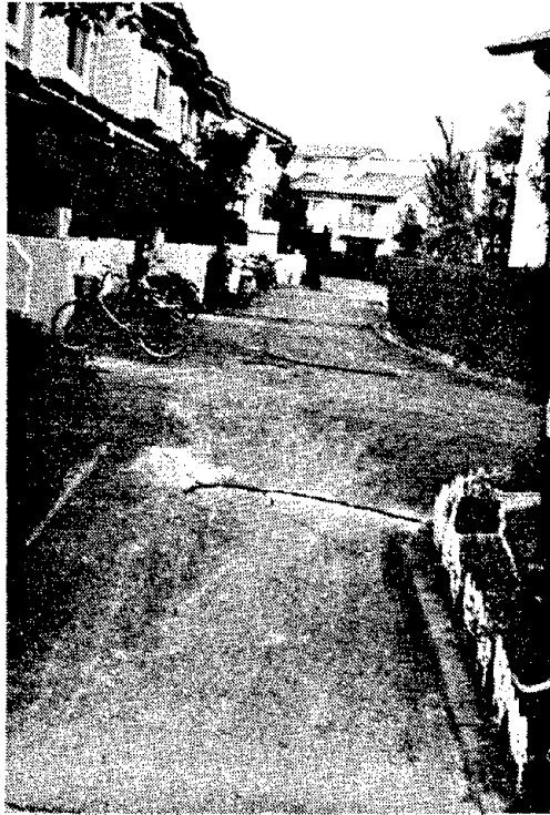
Fig. 4.10 No significant structural damage was evident in this modern residential development in spite of extensive ground deformation due to liquefaction.
