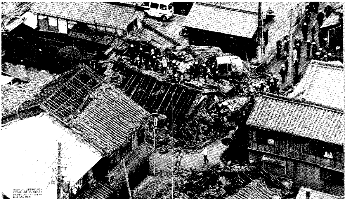
Fig. 5.4 Traditional machiyas in Tsuna-cho, on the northern part of the island of Awaji-shima. Note the lack of diaphragms in the roofs. The machiya at the bottom left resembles a classic Kyoto machiya. The one in the central illustrates the long narrow lot with residence behind. (ill. Asahigraph, Special edition of Kansai Earthquake , February 1, 1995)
