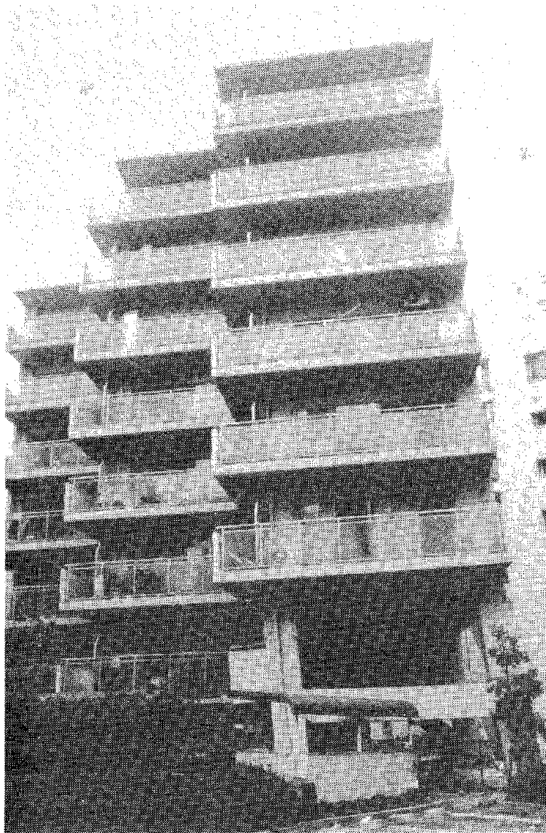
Fig. 6.44 Nine-story building with failed first-story columns
