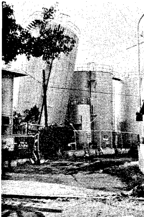
Fig. 4.9 Listing tank in the Nippon Gatx tank farm.
