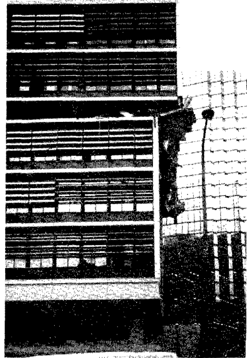
Fig. 6.78 View of end of Annex building showing offset above collapsed story
