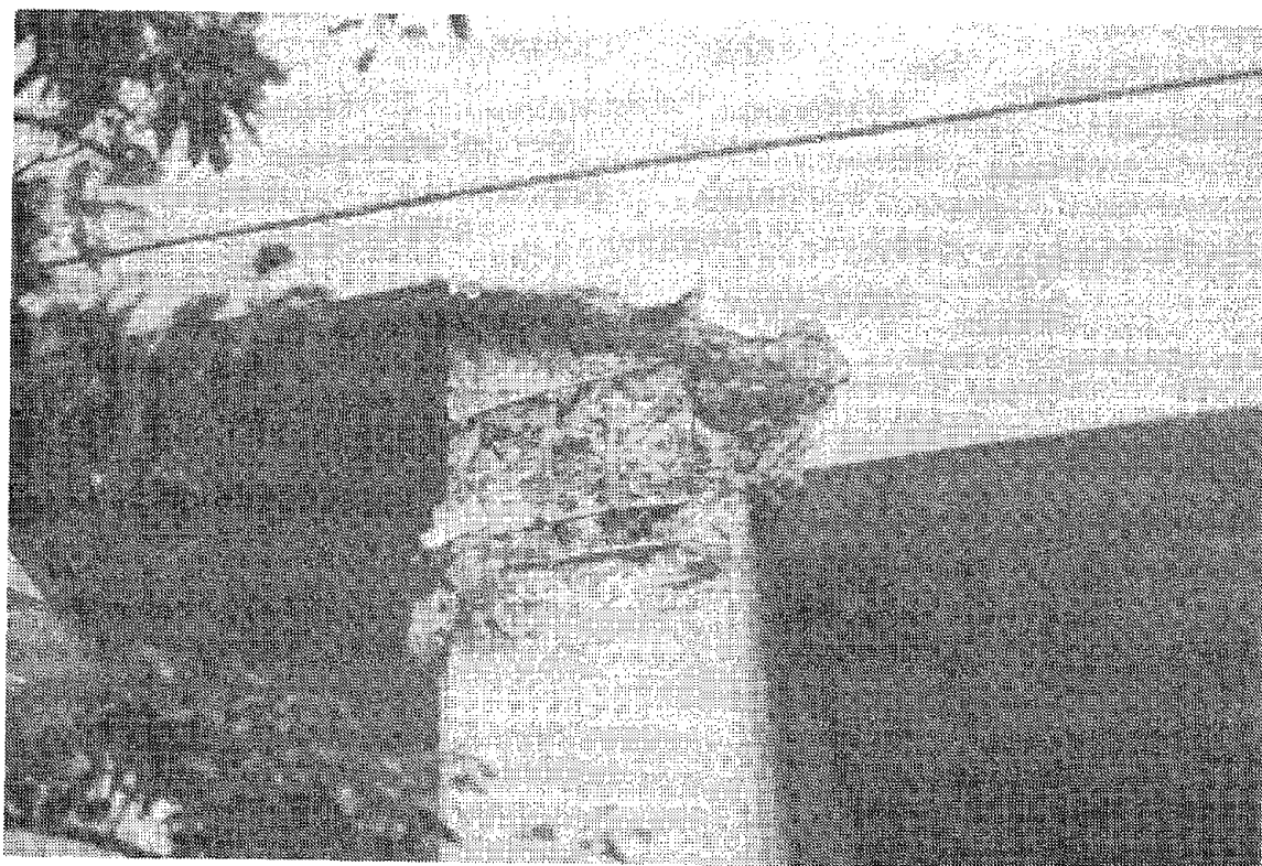
Fig. 6.50 Damage to a modern beam-column joint
