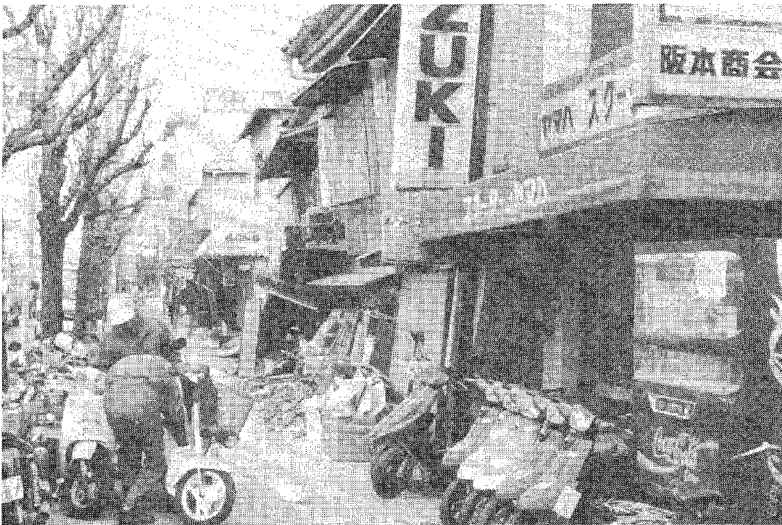
Fig. 5.8 Machiyas still standing but gravely damaged in Ashiya. Each demonstrates the effects of soft stories.
