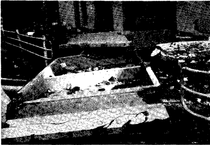
Fig. 6.51 Failure and collapse of precast concrete cladding
