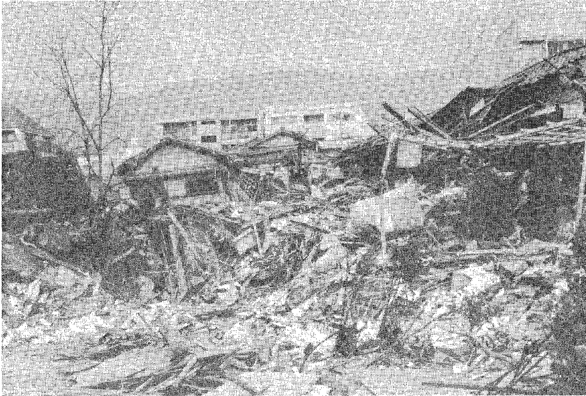
Fig. 5.7 Machiya ruins in Ashiya. The lack of metal fasteners, plywood and plastic and the abundance of small pieces of wood, sand, and terra-cotta make these structures completely recyclable.
