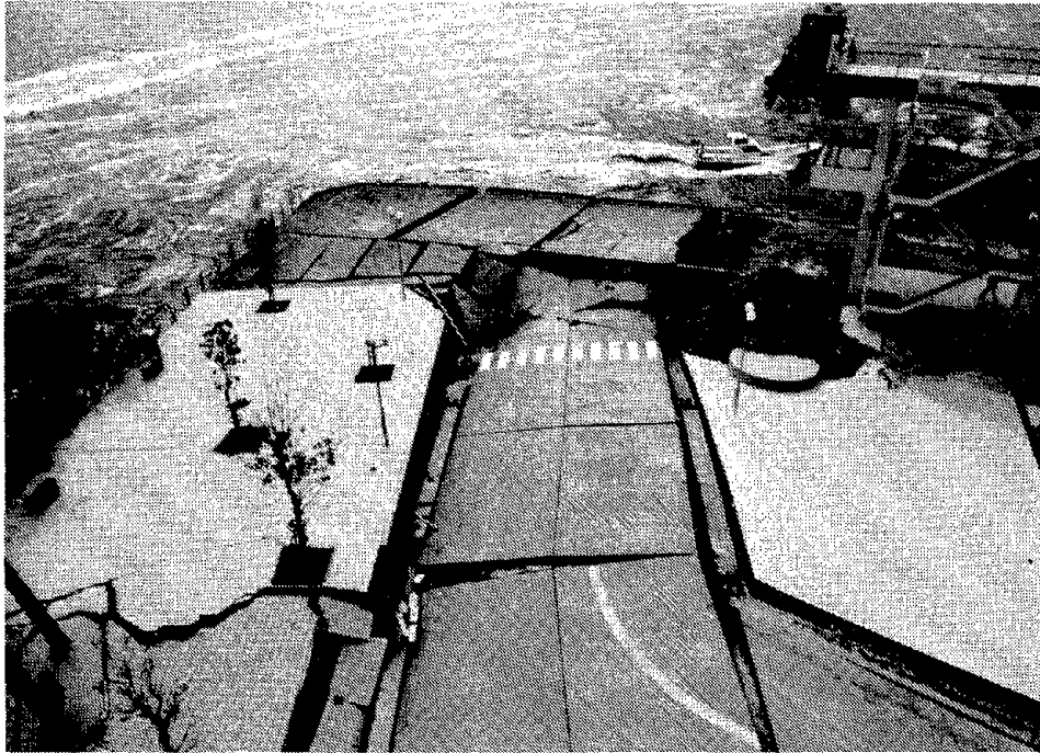
Fig. 7.38 Settlement on northeast side of Port Island bridge
