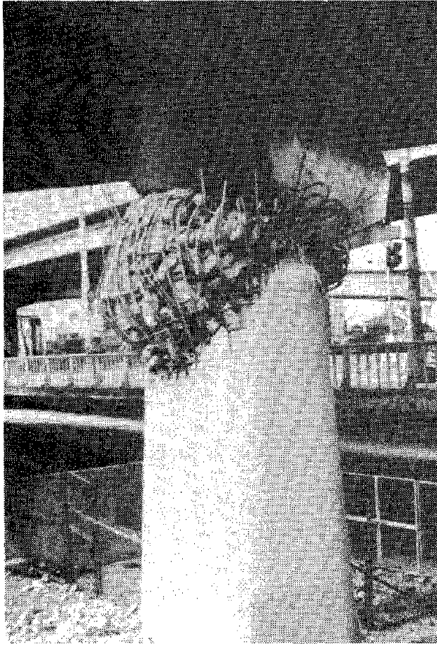
Fig. 7.13 Splice failure just under pier cap
