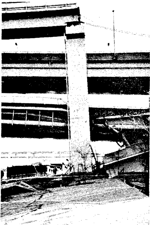
Fig. 4.7 Tilted pier of the Rokko Island causeway.
