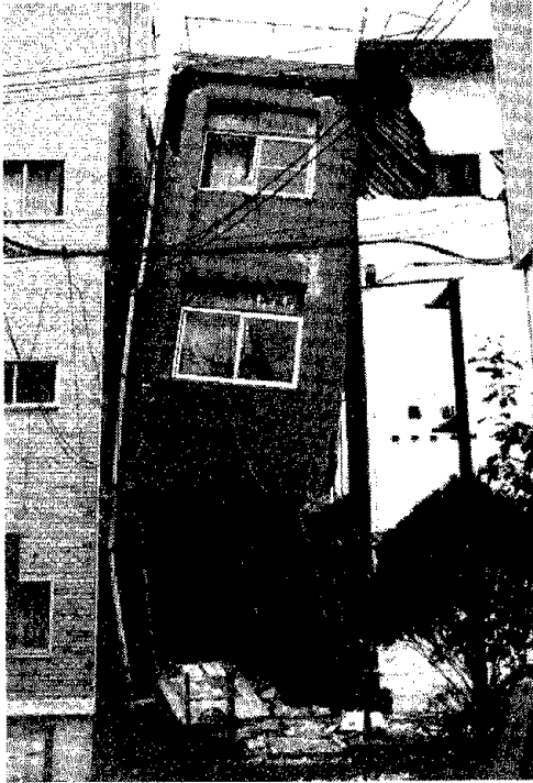
Fig. 6.88 Soft and weak story failure of a steel moment frame building
