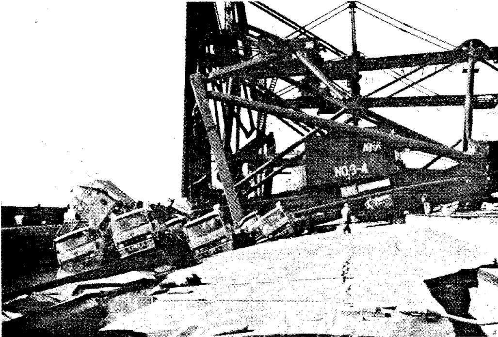
Fig. 4.2 Crane collapsed due to outward lateral movement of the quay wall on Rokko Island. The depth of the resulting graben is \approx 2 m.
