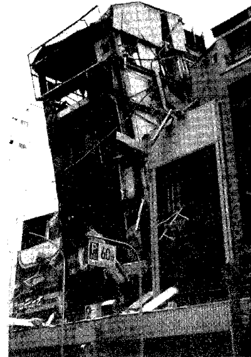
Fig. 6.91 Excessive sway due to fracture of slender braces
