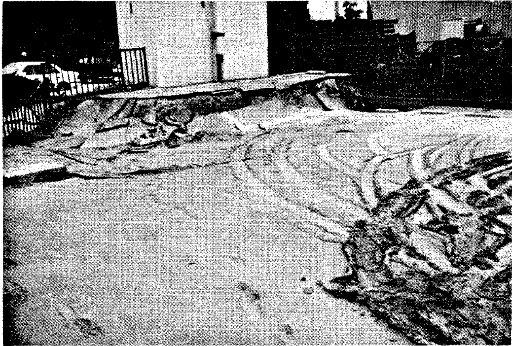
Fig. 4.4 Liquefaction-induced differential settlement ( \approx 40 cm) next to a pile-supported pier of the elevated railway on Port Island.
