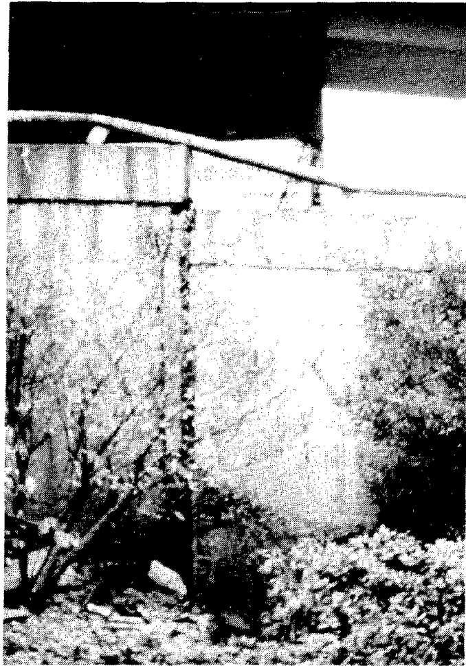
Fig. 7.34 Abutment settlement
