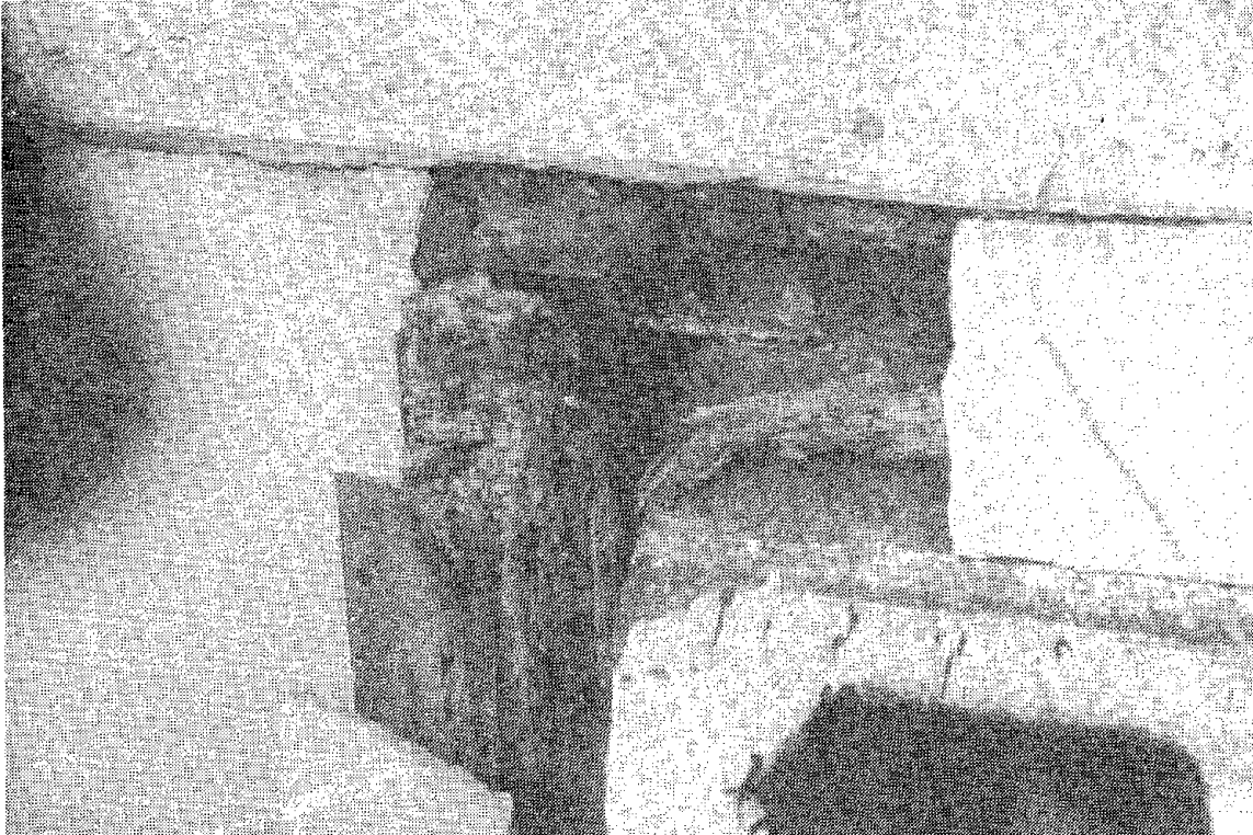
Fig. 5.13 Machiya in downtown Kobe. Detail of termite-damaged connection.
