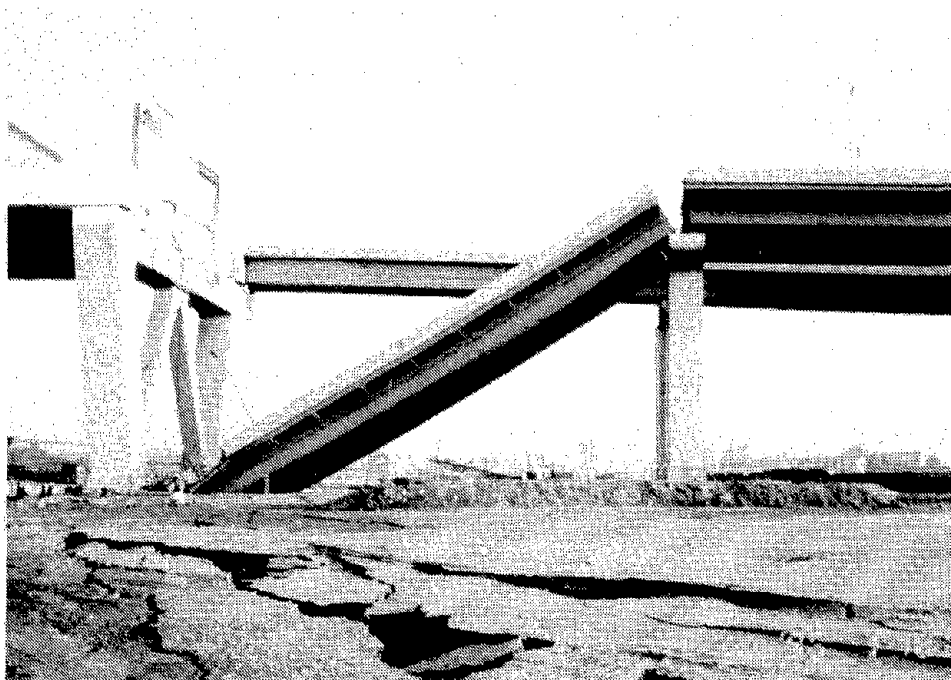
Fig. 7.18 View of collapsed span from the south
