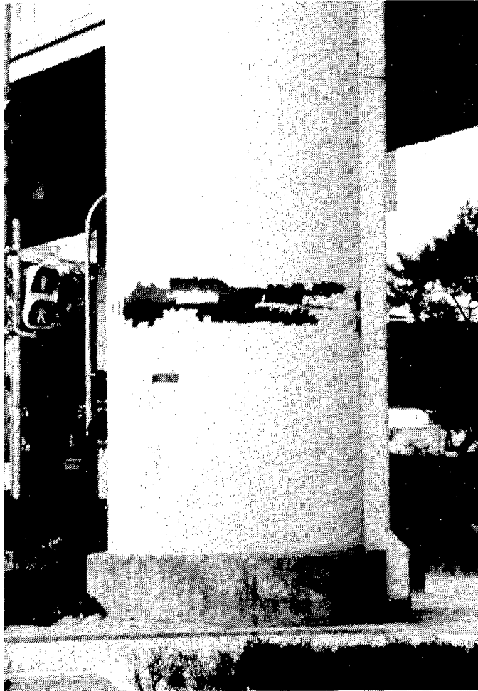
Fig. 7.44 Buckled steel column
