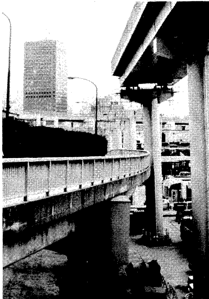
Fig. 7.41 Inclined piers on elevated railway
