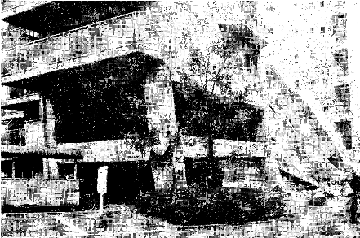
Fig. 6.143 Collapse of elevated walkways connecting apartment blocks
