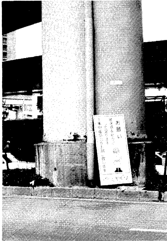
Fig. 7.42 Buckling at base of steel column
