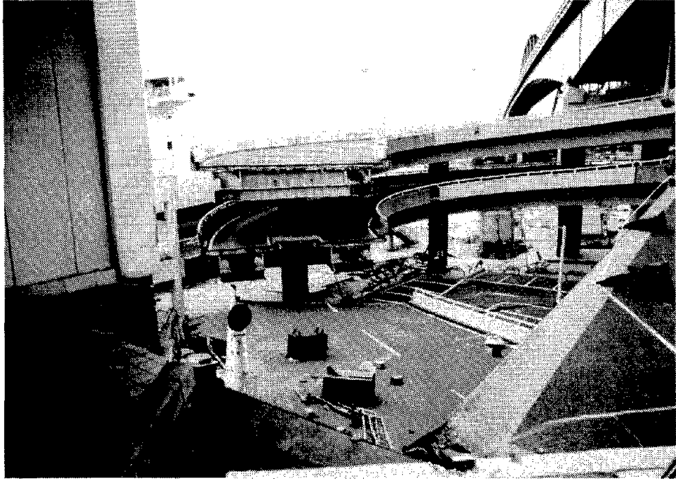
Fig. 7.40 Dropped span in parking structure at north end of Port Island bridge
