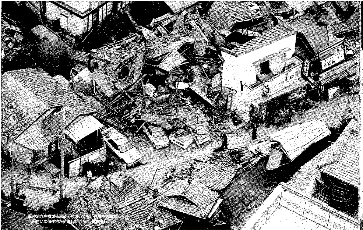
Fig. 5.3 The collapse of machiyas along the Kokudo route 2 in Ashiya. Note the collapses seem to have occurred as buildings twisted under the weight of the tile roofs. (ill.: Asahigraph, Special edition on Kansai Earthquake , February 1, 1995)
