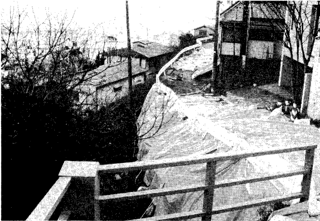
Fig. 4.18 Road embankment deformed by lateral and vertical displacements.
