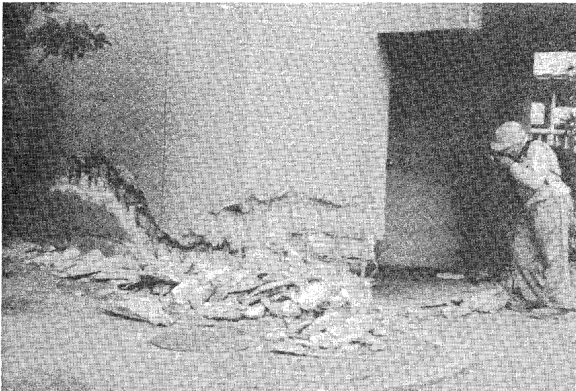
Fig. 6.56 Damage to a reinforced concrete structural wall
