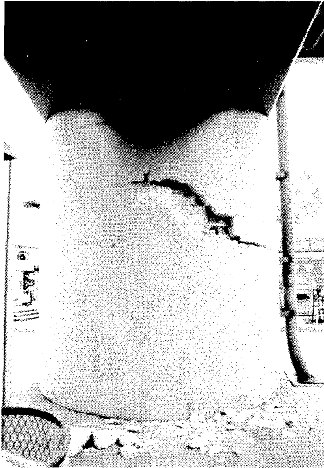
Fig. 7.43 Spalling in large modern column
