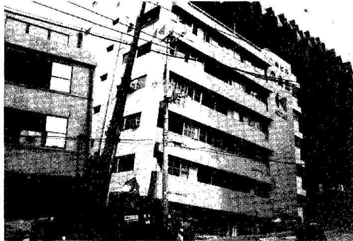
Fig. 6.26 First story collapse
