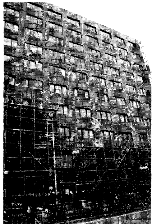
Fig. 6.41 Damage to shear-critical reinforced concrete columns; post-1981 construction
