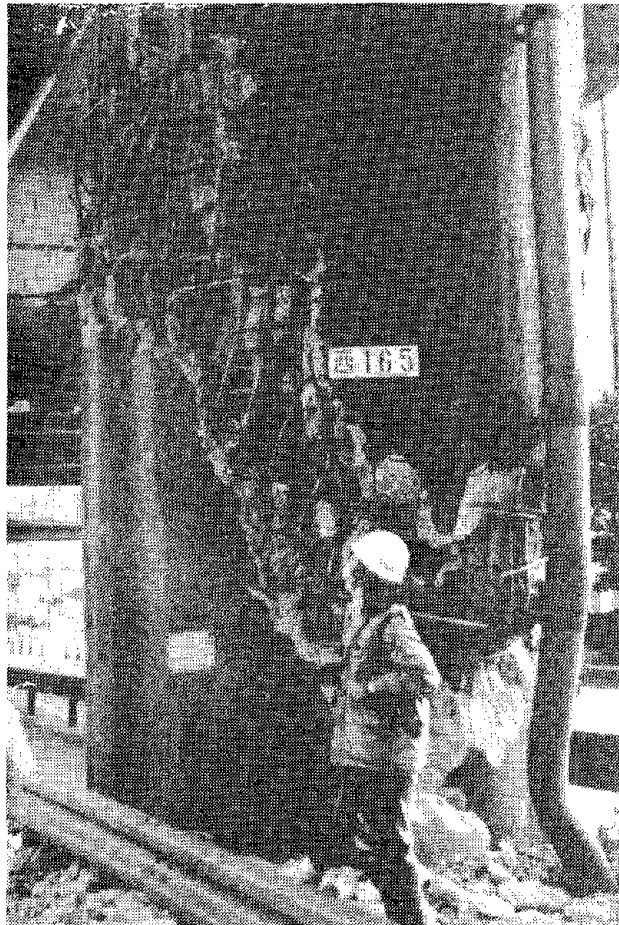
Fig. 7.15 Splice failure followed by shear failure of circular pier
