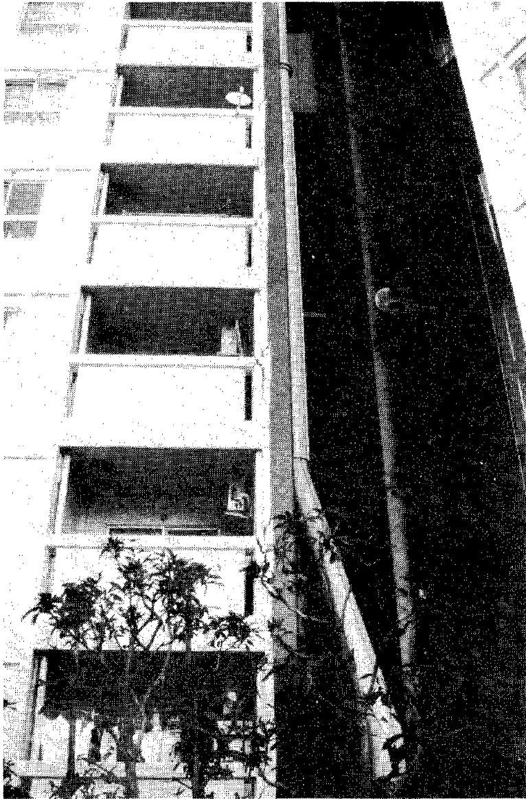
Fig. 6.137 Lightly-damaged precast cladding
