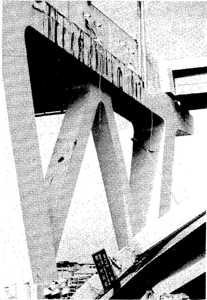
Fig. 7.17 Restrainer failure in approach span to Nishnomiya Ko tied arch bridge
