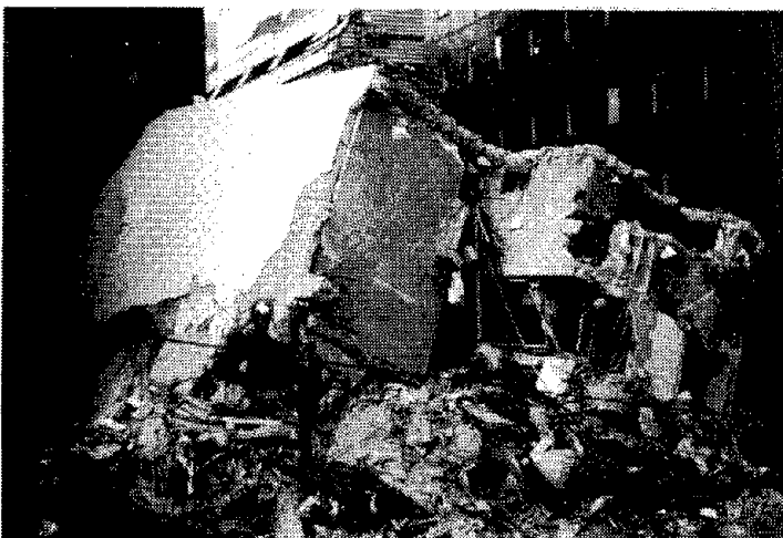
Fig. 6.54 Complete collapse of reinforced concrete building; pre-1971 construction
