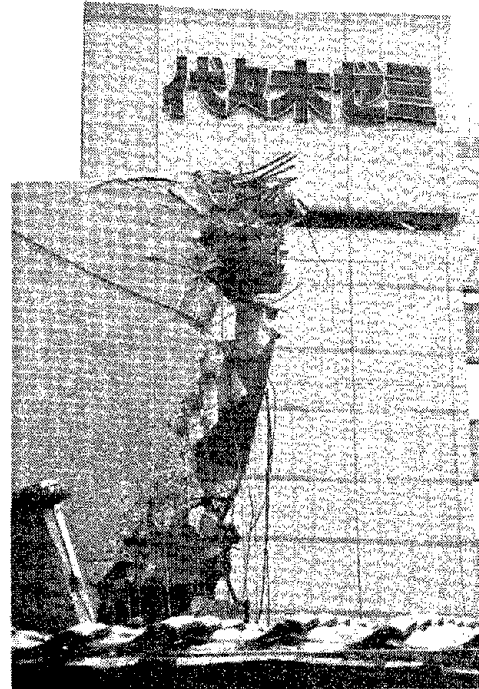
Fig. 6.32 Overturned nine-story building
