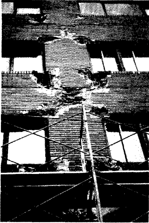
Fig. 6.45 Shear-cracking in a beam-column joint; post-1981 construction
