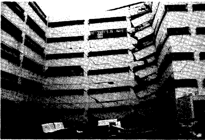
Fig. 6.63 Elevation of courtyard wall in the collapsed building
