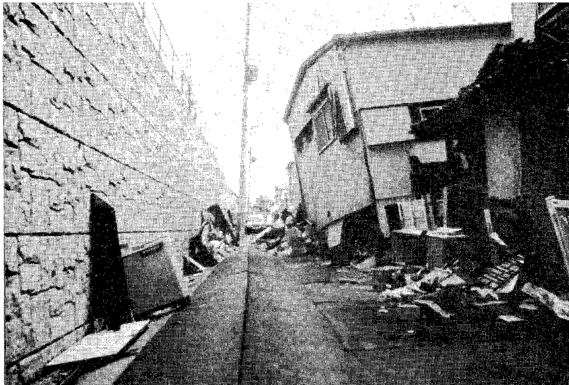
Fig. 4.19 This mechanically stabilized wall experienced only minor deformation in contrast to the extensive damage to the residential structures in the vicinity.
