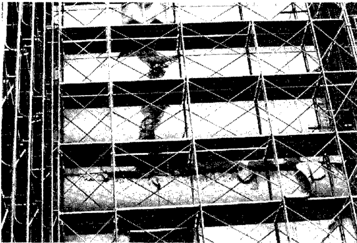
Fig. 6.69 Heavy damage to reinforced concrete structural walls
