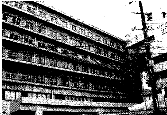
Fig. 6.39 Mid-height story collapse - West City Hospital
