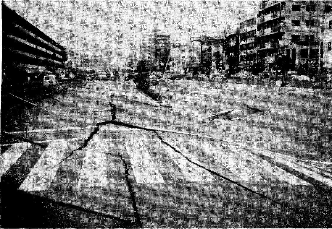
Fig. 4.16 Collapsed street surface over Dakai Station.
