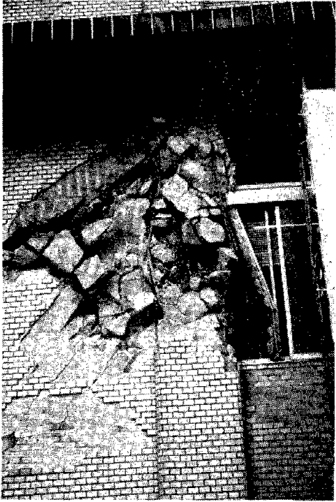
Fig. 6.74 Failed SRC boundary element at the edge of the wall shown in Figure 6.72
