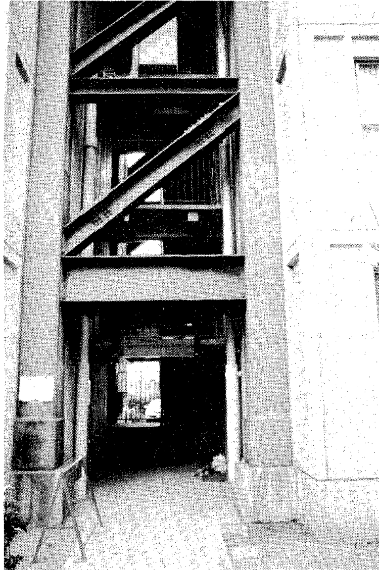
Fig. 6.132 Transition from steel braced frame to steel moment frame
