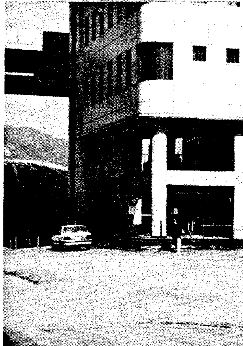
Fig. 4.5 Apparently undamaged pile-supported building. The magnitude of liquefaction-induced differential settlement at the site is \approx 30 cm.
