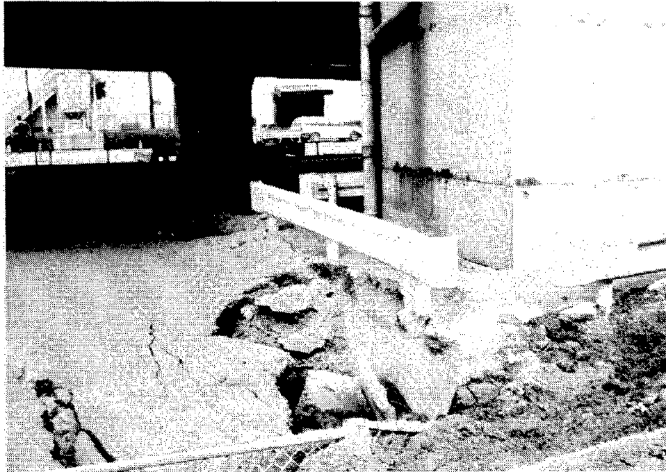
Fig. 7.32 Settlement around piers at south end of Port Island bridge
