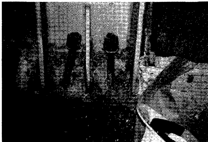
Fig. 6.102 Elongated bolts in a damaged baseplate connection
