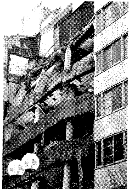
Fig. 6.48 Damage to a haunched beam-circular column joint; pre-1971 construction
