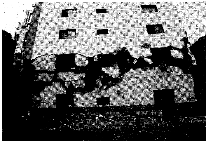
Fig. 6.36 Tension failure of frame-wall - overturned six-story building
