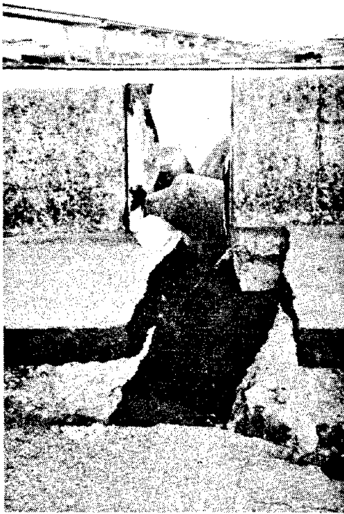
Fig. 4.14 Longitudinal separation of a levee in Ashiya.
