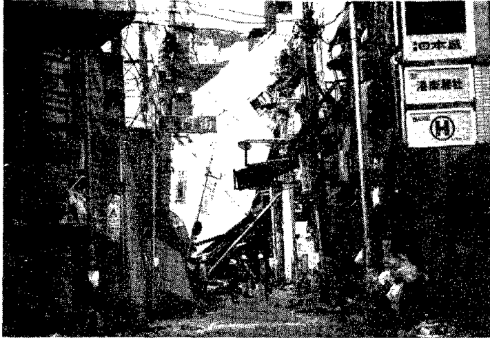
Fig. 6.103 Overturned steel moment-frame building
