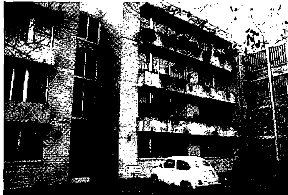
FIGURE 1 DUBLÉ ALMEYDA BUILDING, SANTIAGO, CHILE
