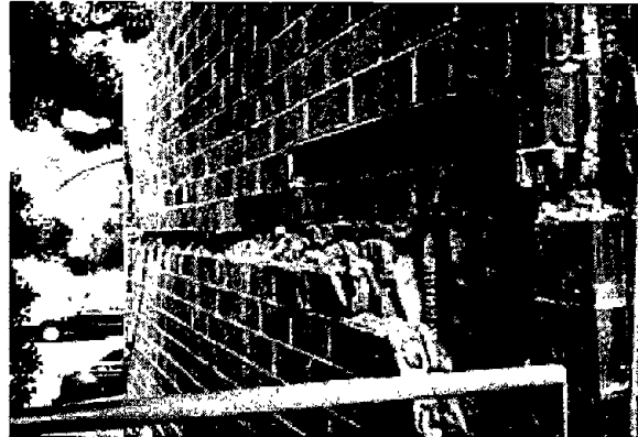
FIGURE 7 CORNER DETAIL OF REINFORCED MASONRY SHOWING CONGESTION
