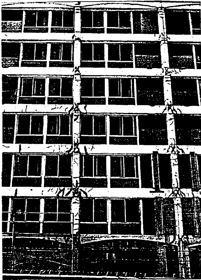
FIGURE 4 EPOXY REPAIR TRACES FOLLOWING NORTHRIDGE EARTHQUAKE
