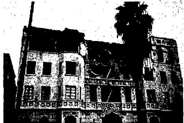
FIGURE 4 URM BUILDING IN SANTA MONICA (1994)
