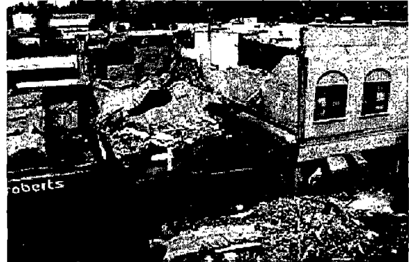
FIGURE 2 OLD URM BUILDING, TOTALLY DESTROYED BY LOMA PRIETA EARTHQUAKE (1989)
