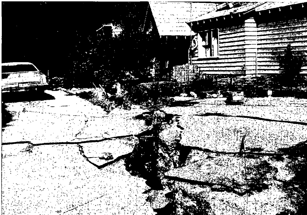
Figure 8.—Segment of Tranbarger fracture (leg A-A', fig. 7A), a 1,200-m-long zone of scarps and cracks in Old Santa Cruz Highway landslide complex. View northwestward from north edge of Summit Road (loc. D, fig. 7A).
