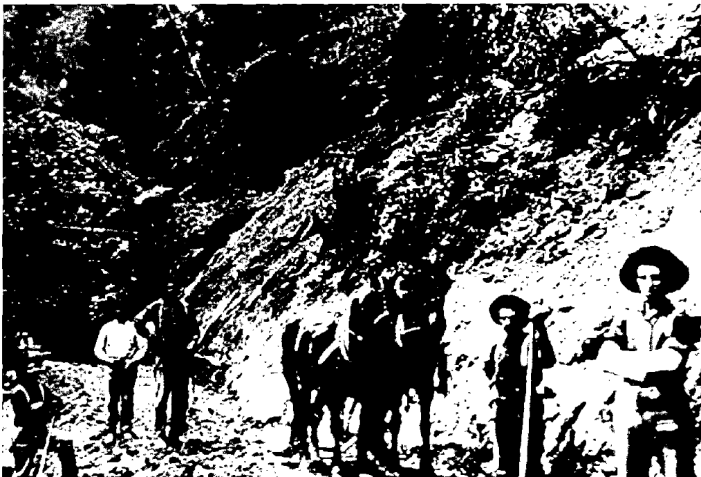
Figure 3.—Workers removing toe of earthquake-induced landslide that dammed Hinckley Creek at Olive Springs sawmill in 1906 (see fig. 4 for location). Landslide killed nine workers at Olive Springs and formed a 20-m-deep impoundment where it dammed the creek. Photograph courtesy of California Department of Parks and Recreation.
