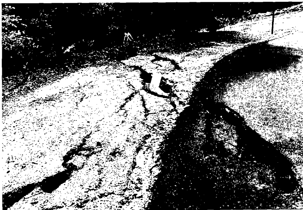
Figure 11.—Part of main scarp of rock block slide on end of ridge near Laurel (see pl. 2 for location). Notebook is 20 by 27 cm.
