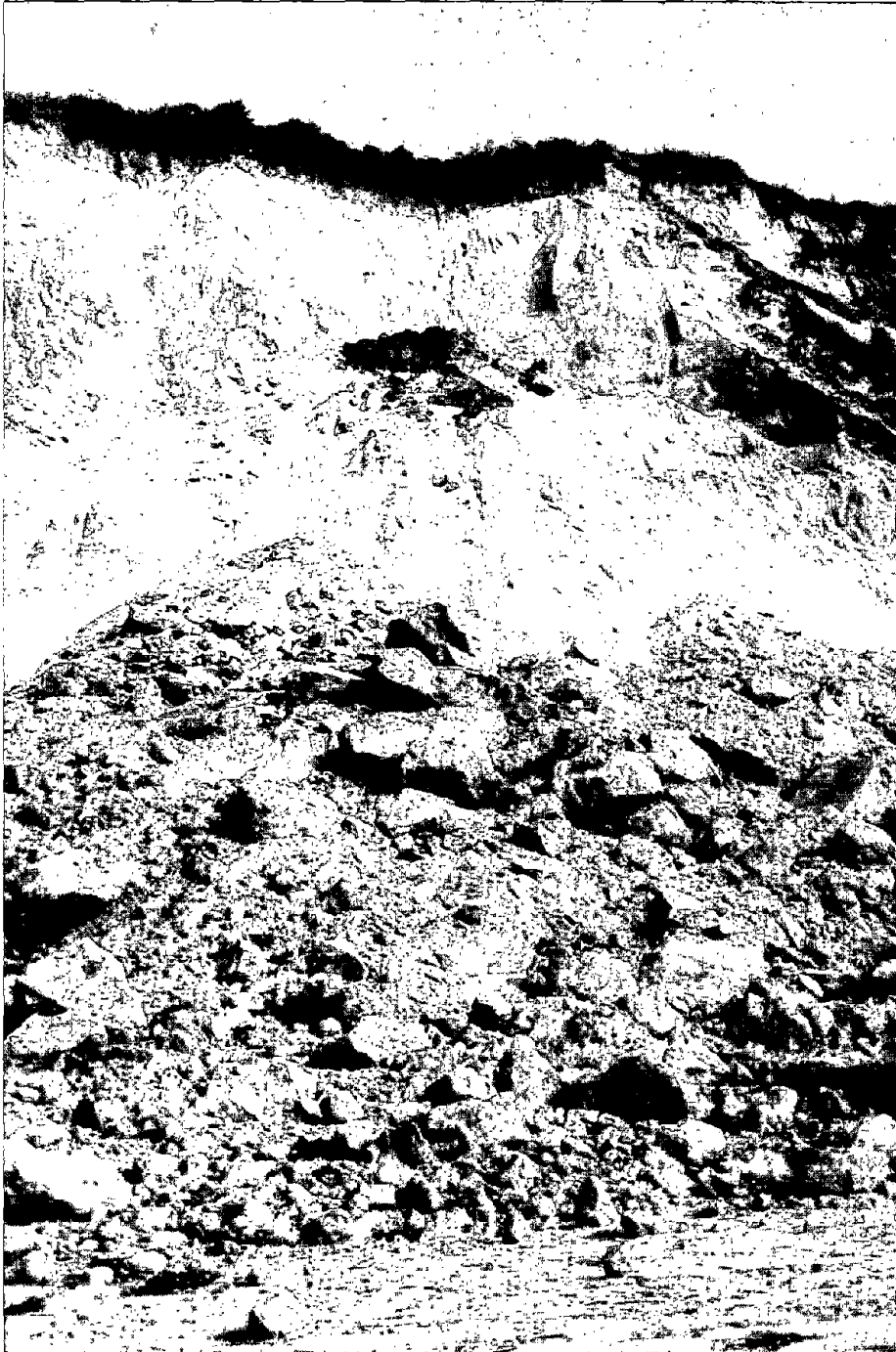
Figure 15.—Coastal landslide about 0.8 km south of mouth of San Gregorio Creek (see fig. 14 for location). Toe of deposit is approximately 60 m wide. Photograph by Mary M. Donato, U.S. Geological Survey.
