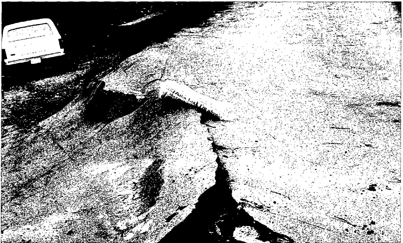
Figure 15.—Internal scarps and compressional features of Villa Del Monte landslide in Deerfield Road area. A , Internal scarps, which are part of a zone about 200 m long. View northeastward from just east of Deerfield Road (loc. K, fig. 12A). B , Internal ridge, consisting of compressed ground, marked by broken and buckled pavement. View northwestward from near east end of Deerfield Road (loc. B' on fig. 12A).
