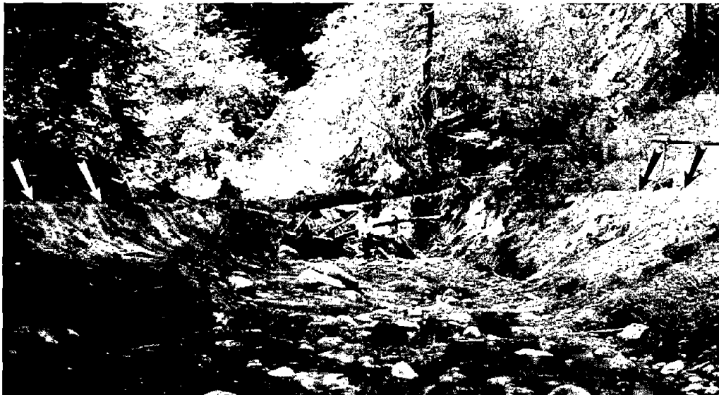
Figure 9.—Downstream view of remnants of 1989 Hinckley Creek landslide dam after it had failed in February 1992. Arrows denote previous shoreline of now-drained 4-m-deep impoundment. Photograph taken May 1992.
