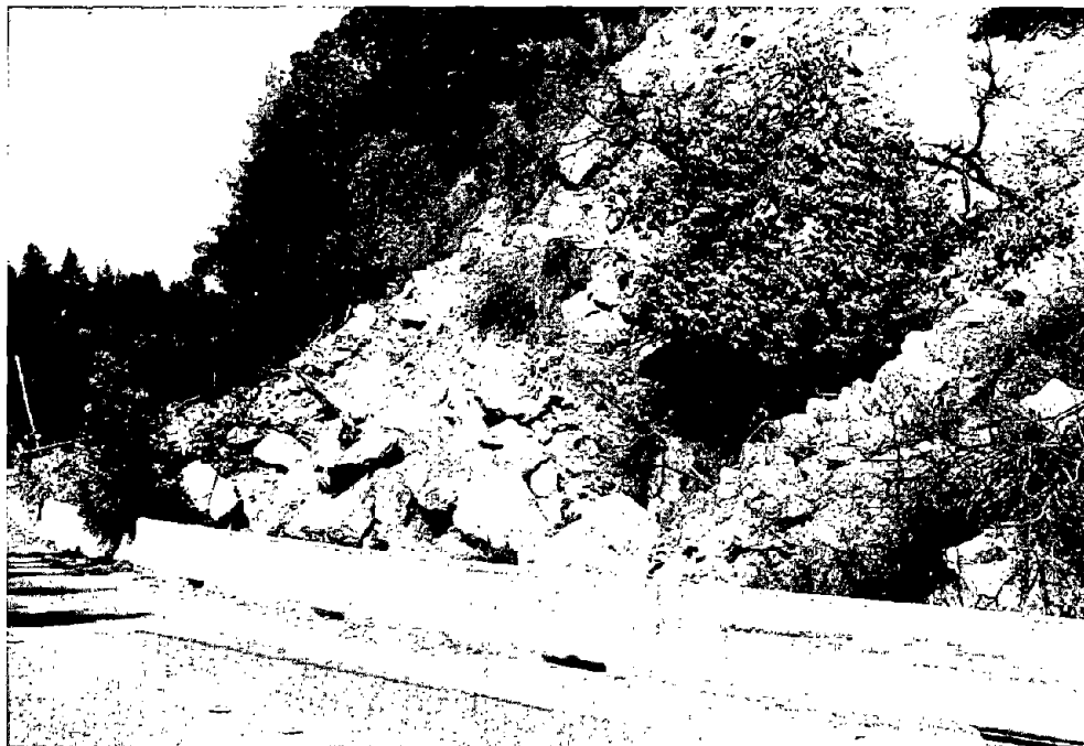
Figure 5.—Part of rock-fall deposit from cut slope above California Highway 17 in Glenwood area (see pl. 2 for location).
