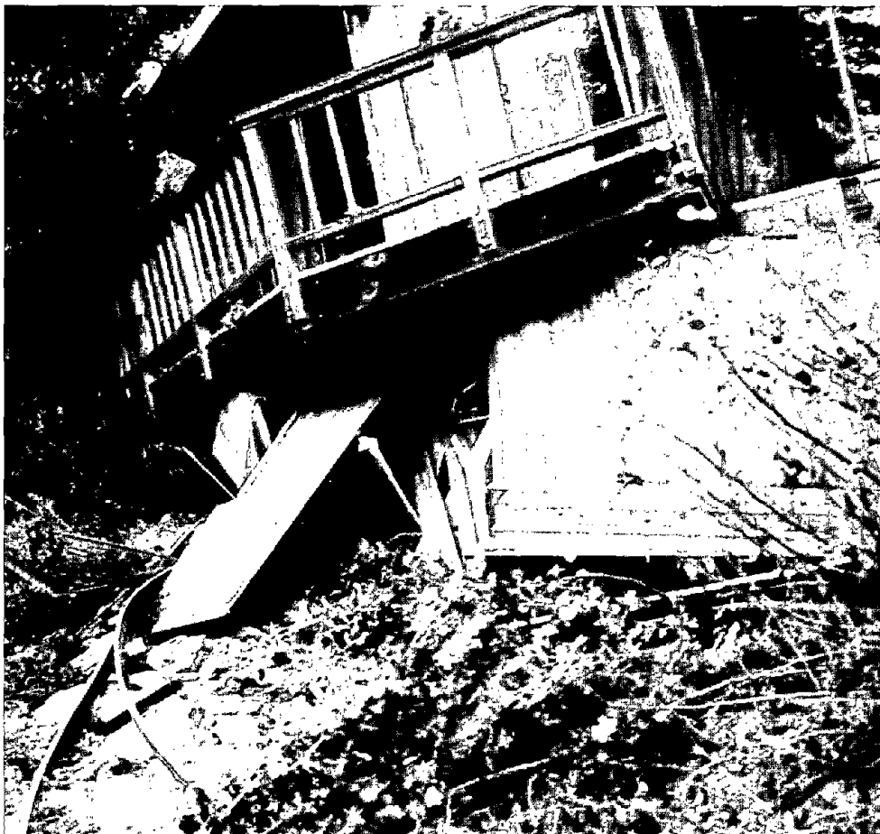
Figure 8.—Severely damaged house on Rebecca Drive landslide (see pl. 1 for location). Main scarp of landslide passes under house. Note ground cracks in foreground.
