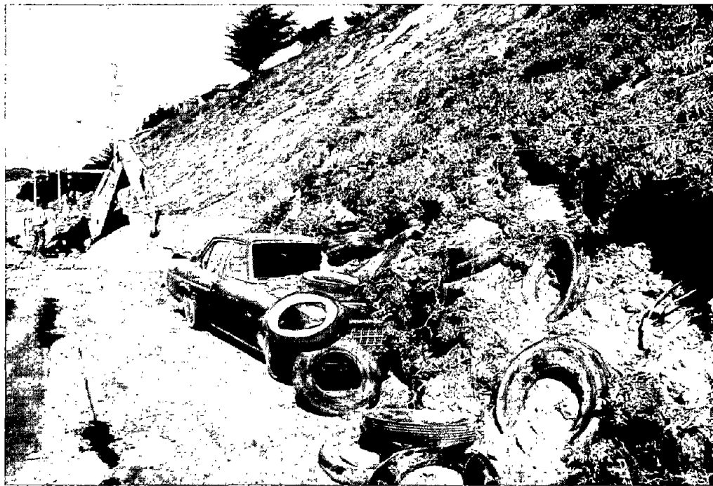
Figure 18.—Weakly consolidated sand of the Aromas Sand disintegrated and flowed downhill to block access and threaten condominiums at base of bluff (see fig. 16). Tires had been placed on slope in an attempt to control erosion.
