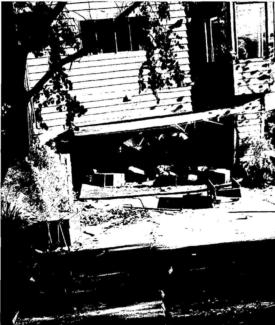
Figure 13.—Ridgecrest fissure and associated landslide along Robinwood Way (see pl. 2 for location). A , Ground crack, also breaking pavement and foundation slab. Crack is nearly linear, trends parallel to long axis of steep, high, narrow ridge, and is immediately upslope from slump shown in figure 13 B . Downslope direction is toward right. B , Rotational slump originating on edge of ridgecrest, immediately below ground crack shown in figure 13 A . Position and orientation of crack and relation to slump indicate that crack is an incipient landslide feature.
