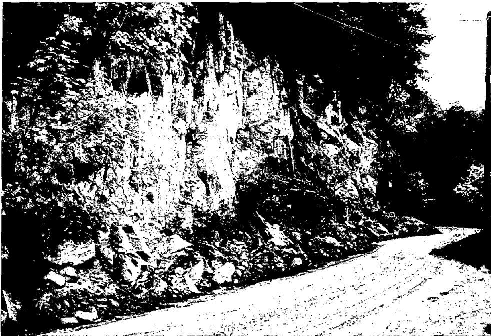
Figure 3.—Rock fall from near-vertical cut along Old San Jose Road, about 0.9 km northwest of Sugarloaf Mountain (see pl. 2 for location). Source rock is weakly to moderately cemented sandstone, broken by conspicuous, through-going joints. Estimated volume of deposit is 500 to 1,000 m 3 .
