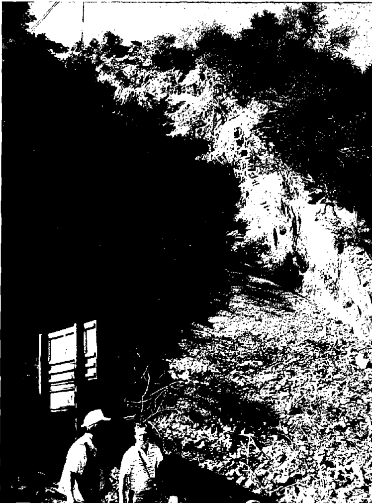
Figure 2.—Part of deposit from complex of rock falls and rock slides along California Highway 17 at Santa Cruz-Santa Clara County line (see pl. 1 for location). Landslide source was in intensely fractured rock.
