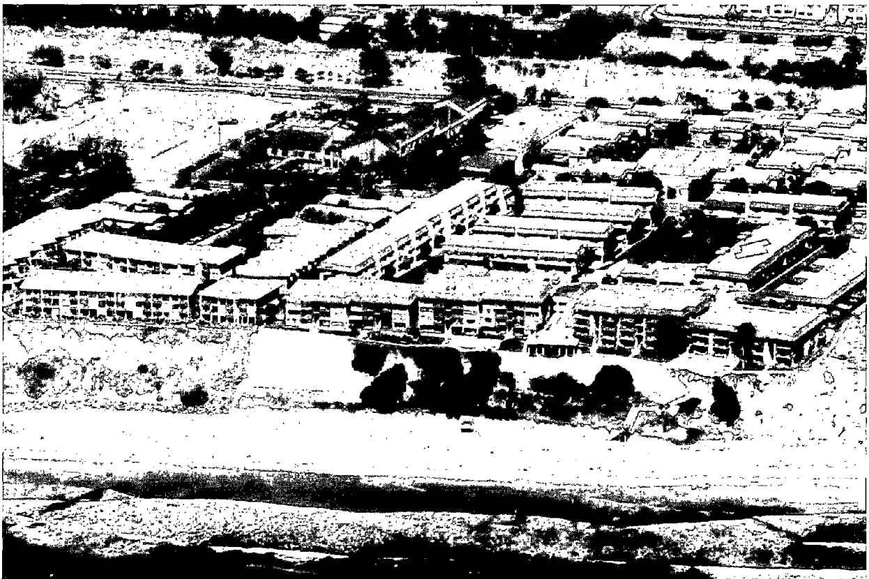
Figure 3.—Intense blufftop development along coast of San Diego County, showing use of seawalls and gunnite to reduce bluff failure.
