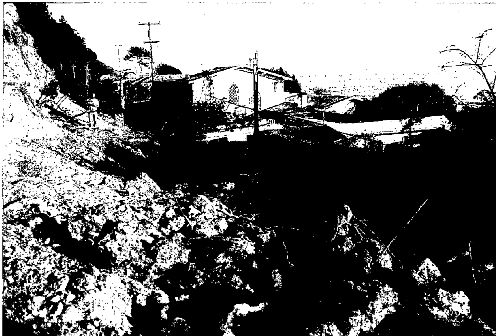
Figure 14.—Base of seaciff in area of figure 12 where material from bluff failure has blocked access to beach-front homes.
