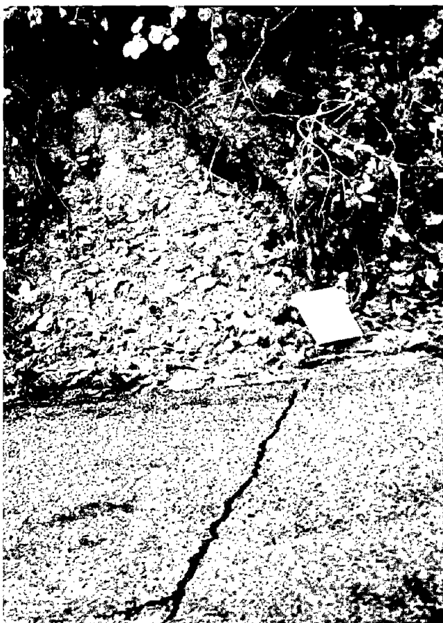
Figure 12.—Lateral margin (left flank) of block slide near Laurel (see pl. 2 for location) defined by crack across road, showing left-lateral movement. Note small rock fall where crack intersects steep cut slope across road.
