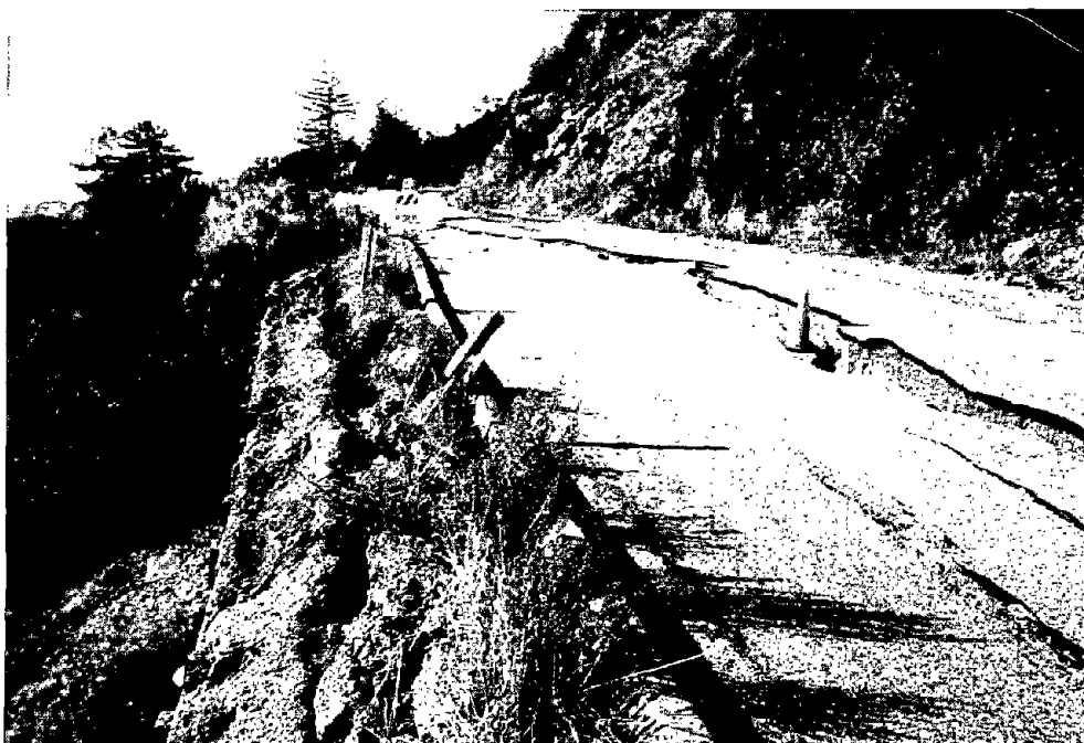
Figure 7.—Small slump in road fill near Bean Hill (see pl. 2 for location). Note arcuate, concave-downslope main scarp nearly parallel to long axis of road. Slumps in fill were most common type of category II landslides in the southern Santa Cruz Mountains. Photograph by David M. Peterson, U.S. Geological Survey.
