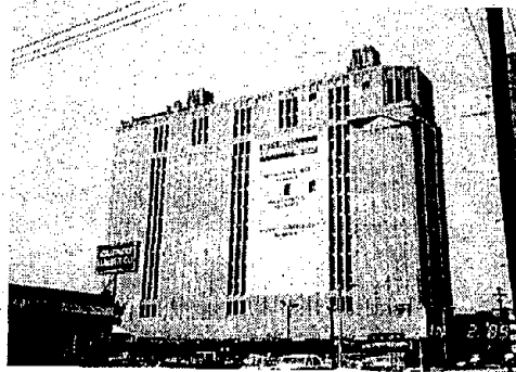
Los Angeles - Hollywood Storage Bldg. (CSMIP Station No. 24236)
