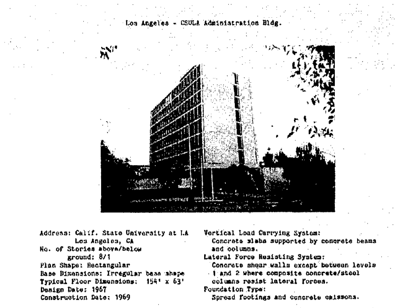
Figure C.15.1a. Details of 8-story CSULA administration building, CSMIP Station No. 24468
