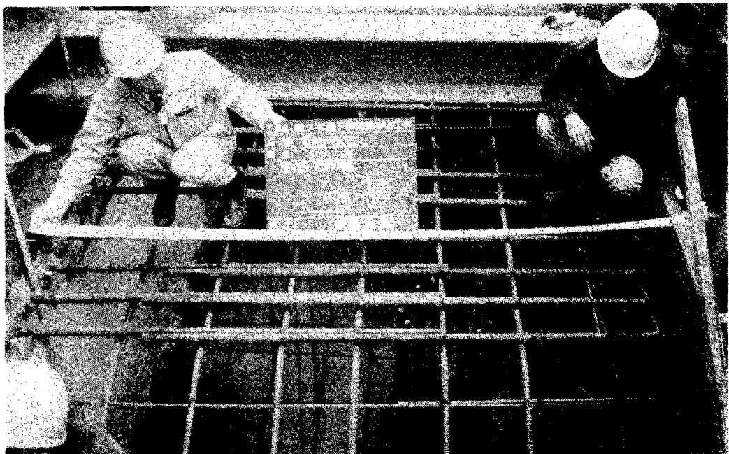
Photo 6 Reinforcement of at the New Footing
