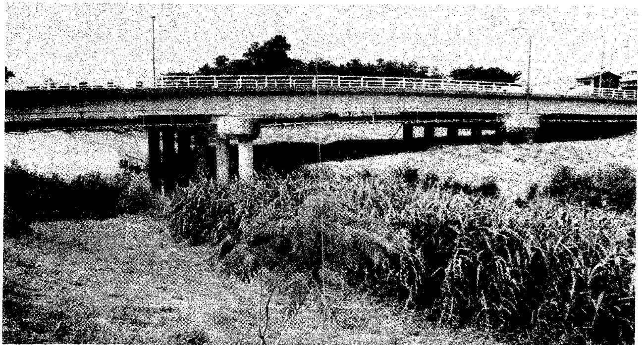
(a) Before the Seismic Strengthening
