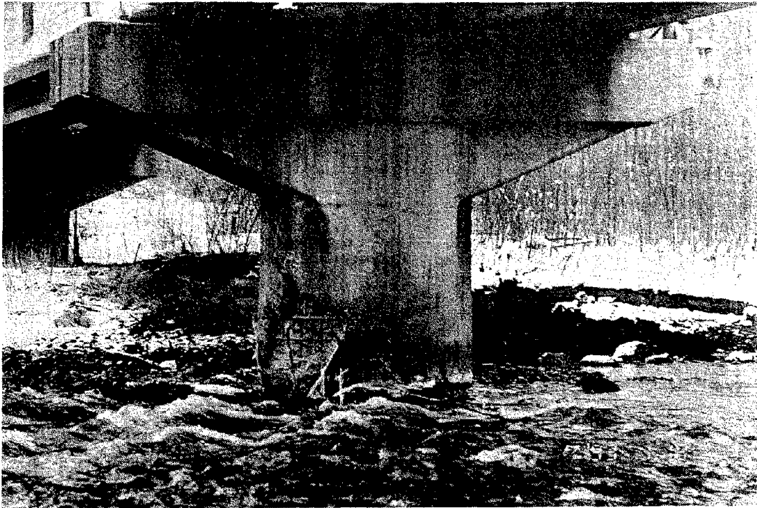
Photo 4 Spalling-off of Cover Concrete and the Bucking of Main Reinforcement of Matsunoe Bridge (Pier P4)
