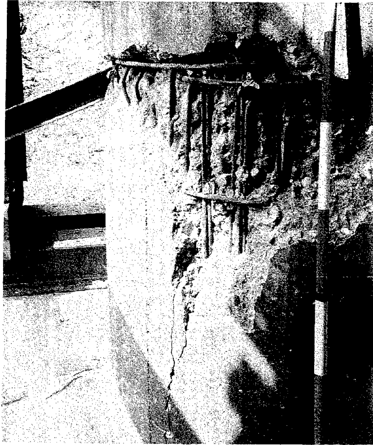
Photo 11 Damage to Pire of Motouriya Bridge
