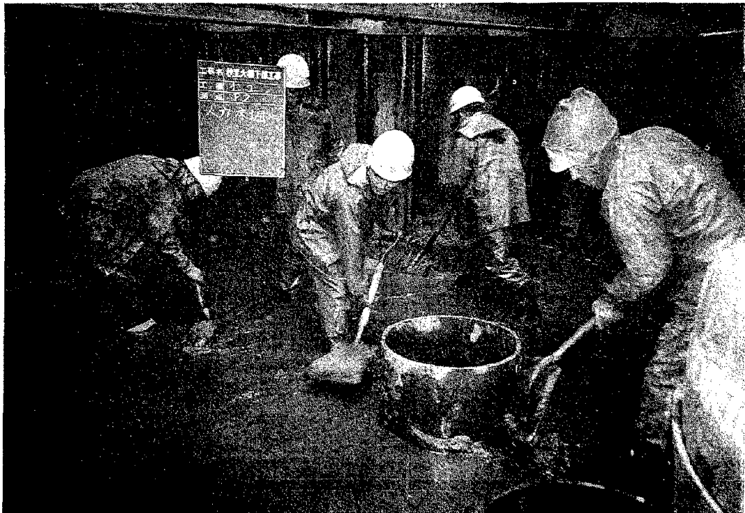
Photo 10 Excavation by Manpower and the Head of New Pile
