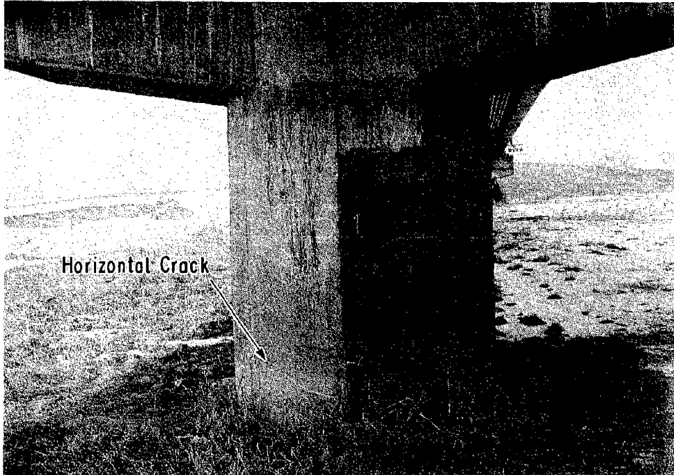
Photo 5 Cracks of Gojukkoku Bridge
