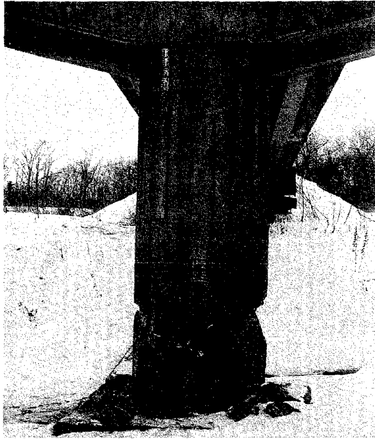
Photo 9 Damage to Pire P2 of Yoda Bridge
