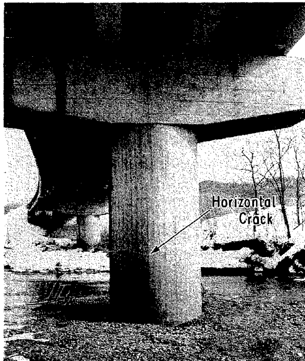
Photo 8 Cracks of Akagawa Bridge (Pire P2)
