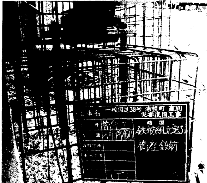
Photo 8 Repairing Abutment of Chokubetsu
