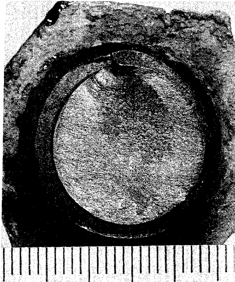
Photo 21 Cutting Surface of Bolts (Hatsune Bridge)
