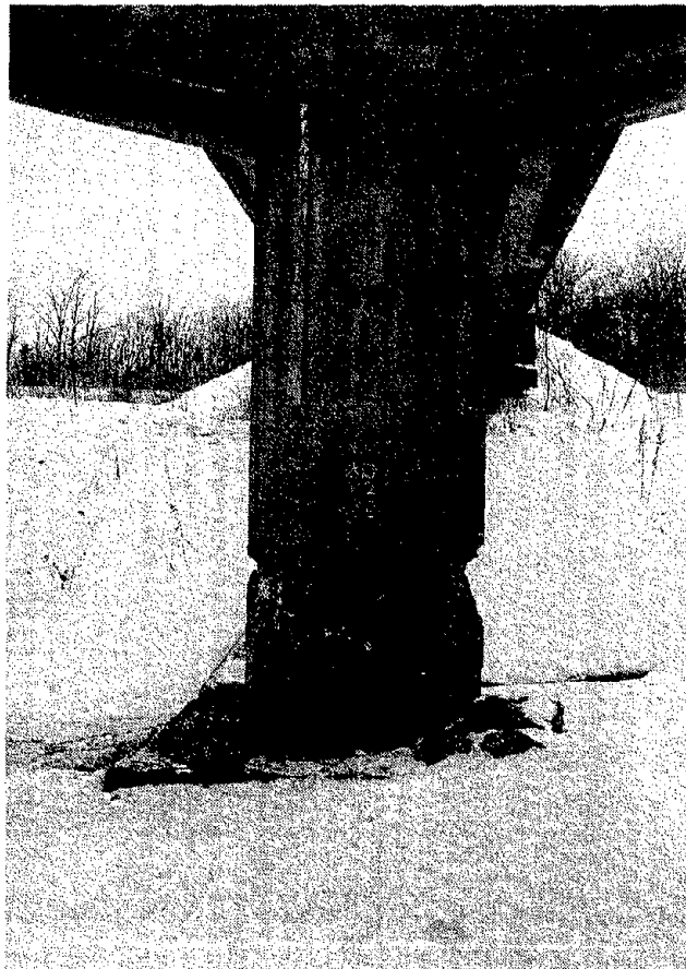
Photo 1 Damage of Yoda Bridge
