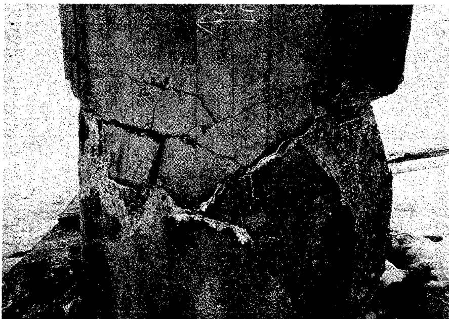
Photo 2 Failure at Termination Point
