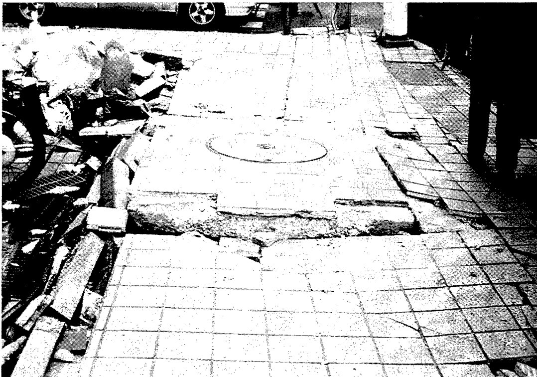
Figure 26 There was relative motion between this manhole and the surrounding soil. The relative motion could have been due to floating of the manhole or subsidence of the soil. Conduits connected to the manhole were damaged. (Kobe, Japan)
