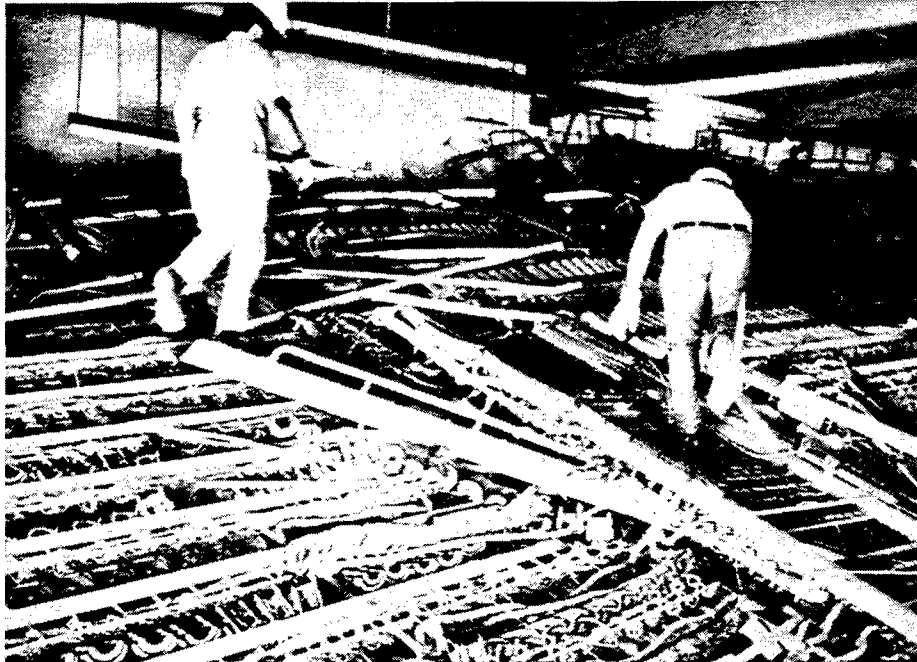
Figure 3 Switching equipment in a CO tipped over when overhead bracing and base anchors failed in a moderate earthquake. The equipment was a total loss and it took several months to replace and install new equipment. It took four days to install temporary lines to provide limited service until regular service could be restored.
