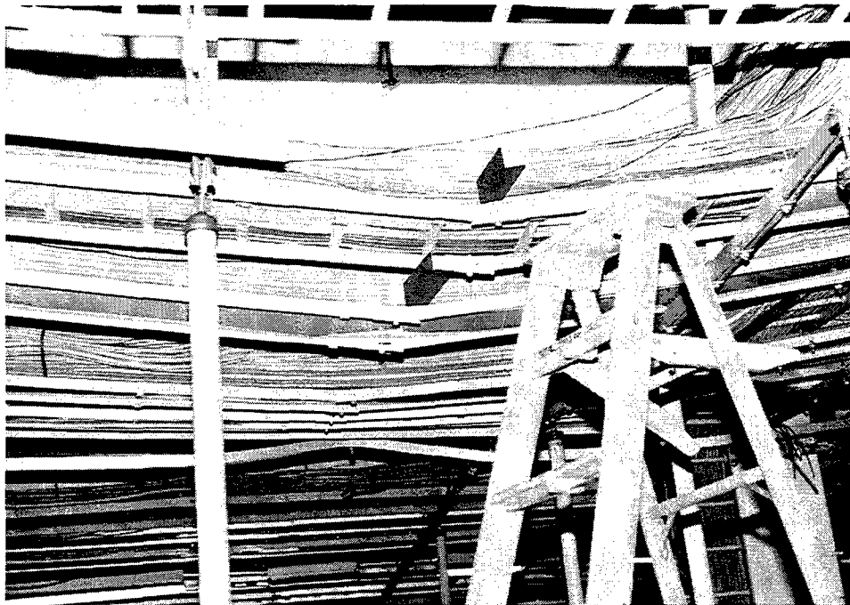
Figure 8 The buckling of the framing system at a splice demonstrated the lack of capacity of the friction clip splice.
