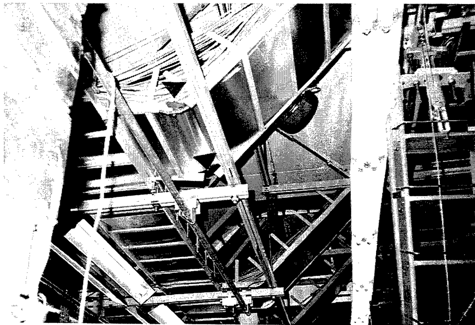
Figure 2 Friction clips used to splice cable racks together have pulled out in earthquakes. A positive structural connection is the preferred method of splicing.
