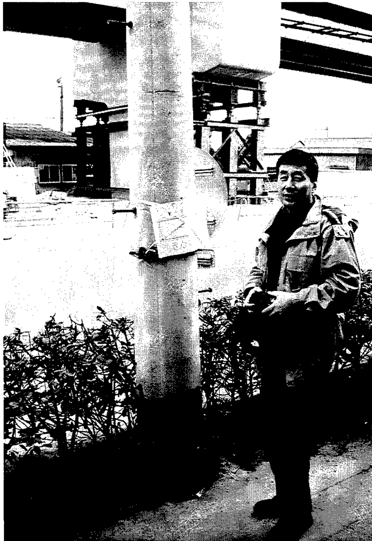
Figure 22 This pole sank about five feet when the soil supporting it liquefied.
