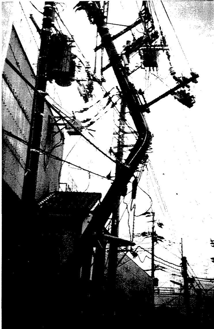
Figure 24 This concrete power pole failed due to induced vibrations in Kobe, Japan earthquake.
