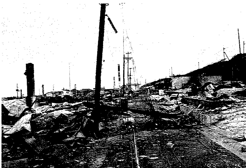
Figure 19 Large areas were destroyed by fire after the Kobe, Japan earthquake. Aerial cables and their wood support poles are vulnerable to fire.
