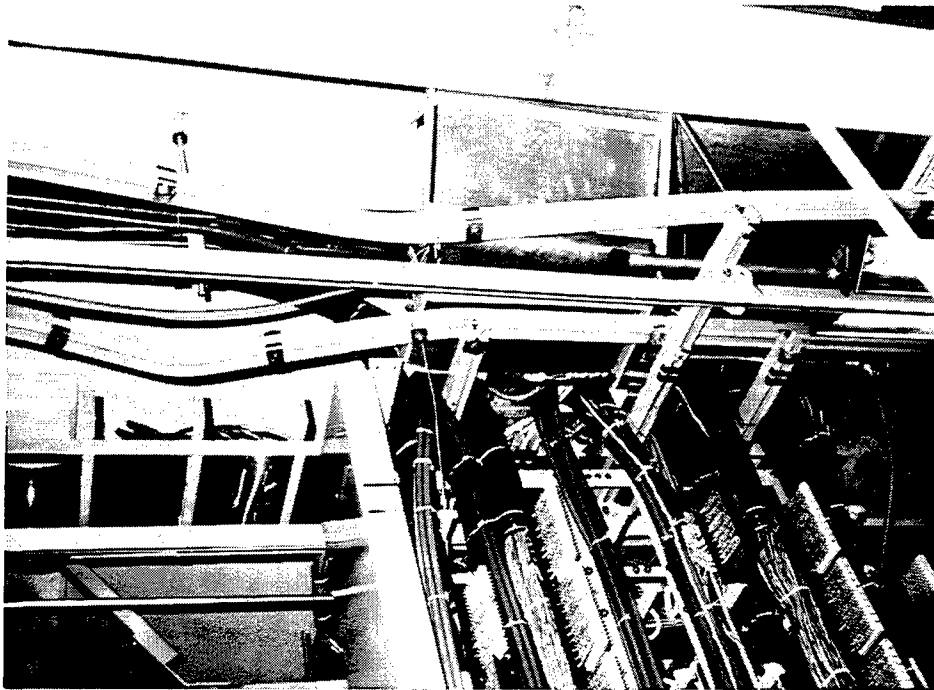
Figure 6 Lateral loads exceeded the capacity of the framing member causing it to buckle. This allows large relative motions of the framing system that can cause impacting of the frame with building columns or exceed the slack provided to conductors.
