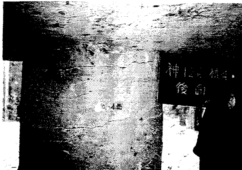
Photo 1 The worst damage found on the pile of the collapsed piltz bridge
