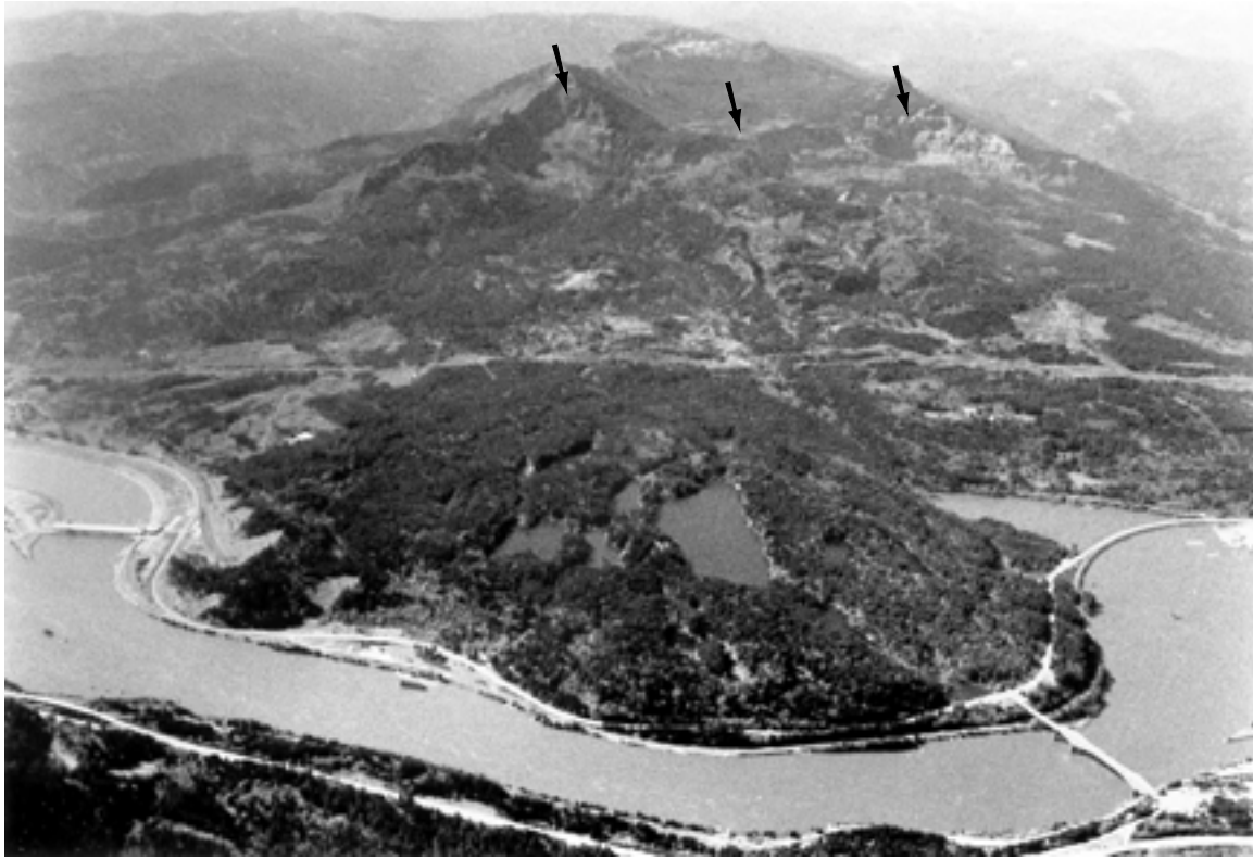
Figure 214. Bonneville landslide area along the Columbia River west of Stevenson, Wash. (pl. 8, loc. 160). Rock fall/rock avalanche activity triggered by the April 13, 1949, earthquake occurred along the steep head scarp (arrows), creating a dust cloud visible for many kilometers along the Columbia River Gorge. Photograph by Derek Cornforth, Landslide Technology, Portland, Oreg.
