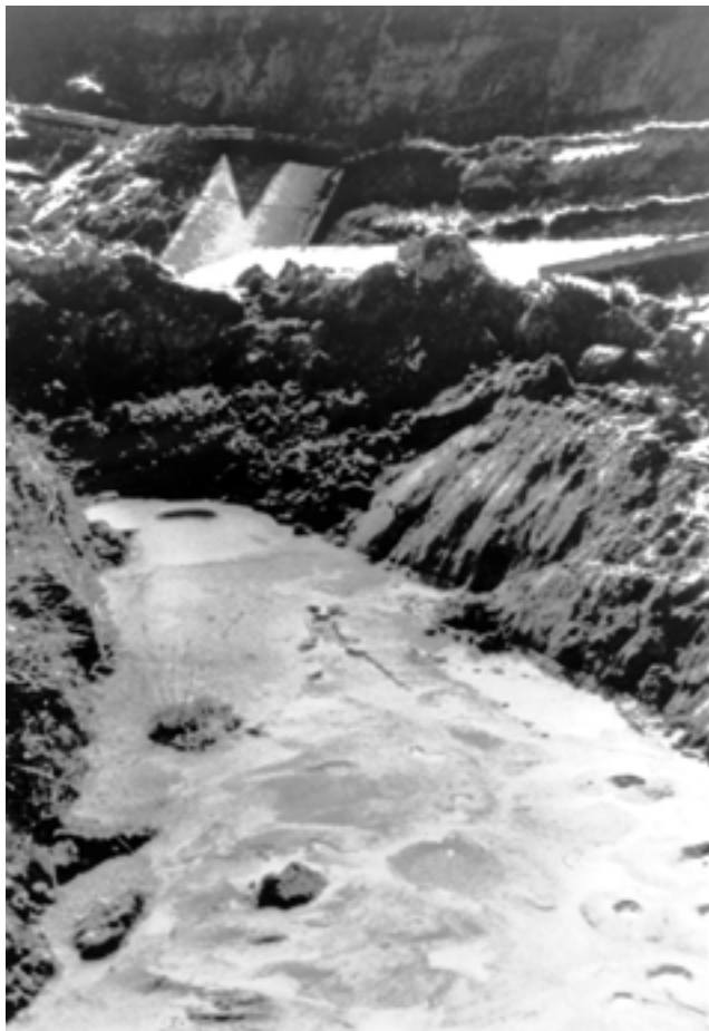
Figure 205. Sand boils near Capitol Lake in Olympia, Wash., related to the earthquake of April 29, 1965 (pl. 5, loc. 48). The sand boils are evidence of soil liquefaction at this ground failure location. Sidewalk slab in background shows scale. Photograph by Gerald W. Thorsen, Division of Geology and Earth Resources, Washington Department of Natural Resources, Olympia, Wash.
