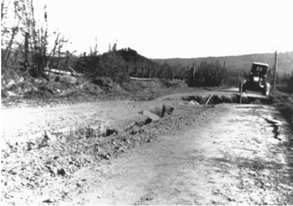
Figure 209. Slump in a 1- to 1.2-m-high road embankment in the Cowlitz River Valley, about 1.6 km southwest of Randle, Wash. (pl. 6, loc. 118). This April 13, 1949, earthquake-induced ground failure occurred in artificial fill underlain by loose liquefiable sand. The earthquake also produced sand boils in an adjacent field. Photograph by Alice Peters, Randle, Wash.
