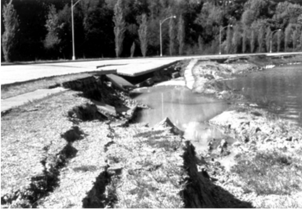
Figure 204. Damage to Deschutes Parkway, Olympia, Wash., resulting from a 1965 earthquake-induced ground failure (pl. 5, loc. 48). The parkway was constructed on granular fill placed on tidal flat muds that are now within the limits of Capitol Lake; failure was probably due to liquefaction. Photograph by Gerald W. Thorsen, Division of Geology and Earth Resources, Washington Department of Natural Resources, Olympia, Wash.
