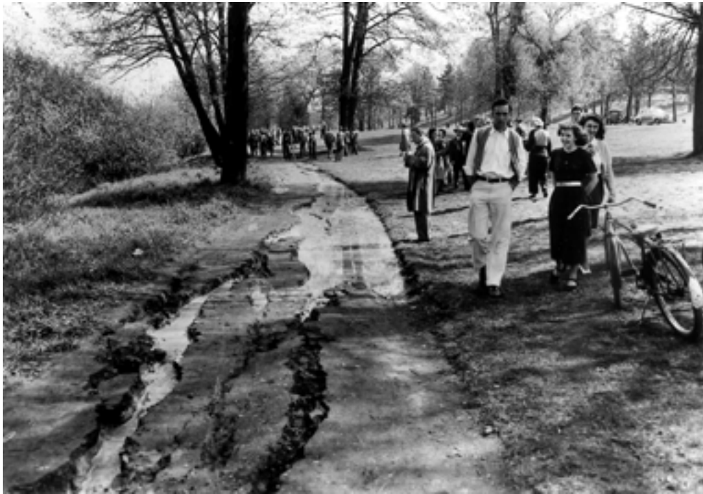
Figure 195. Ground cracks on the southeast side of Green Lake in north Seattle (pl. 4, loc. 33). The cracks opened during or shortly after the April 13, 1949, earthquake and probably resulted from subsidence and lateral movement of ground downslope toward the lake (out of sight to the left of view). Photograph from the Seattle Post-Intelligencer Collection, courtesy of the Museum of History and Industry, Seattle, Wash.
