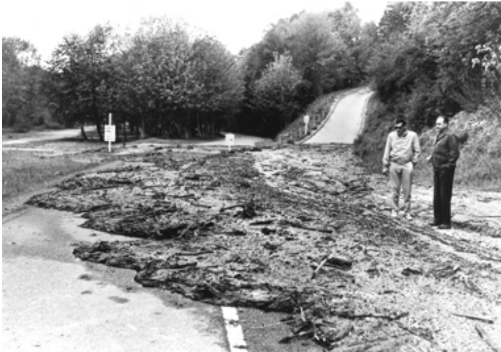
Figure 196. Mudflow covering Carkeek Park Road in northwest Seattle (pl. 4, loc. 36). This mudflow developed as material from an earth slide triggered by the April 29, 1965, earthquake mixed with water and flowed down a Piper Creek tributary ravine. Photograph used by permission of the Seattle Times Co.
