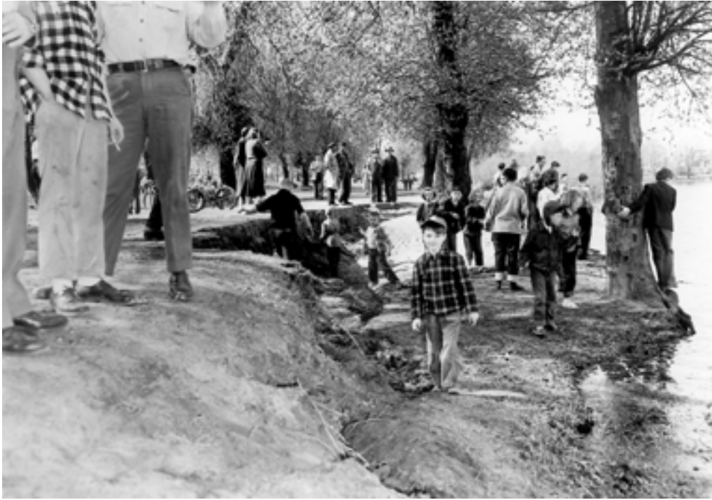
Figure 194. Slump along the shore of Green Lake, north of downtown Seattle. This 1949 earthquake-induced ground failure occurred near the south end of the lake (pl. 4, loc. 33) in an area that subsequently experienced ground failure during the April 29, 1965, earthquake. Photograph from the Seattle Post-Intelligencer Collection, courtesy of the Museum of History and Industry, Seattle, Wash.
