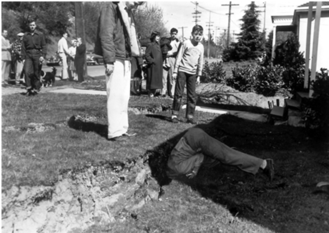
Figure 190. Slumping and settlement in West Seattle (pl. 4, loc. 10) induced by the April 13, 1949, earthquake. The slumping exposed artificial fill (lower left) that underlies the site. Photograph from the Seattle Post-Intelligencer Collection, courtesy of the Museum of History and Industry, Seattle, Wash.
