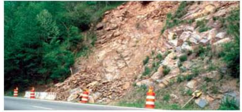
Figure 18. Rockfall near Gatlinburg, Tenn.
