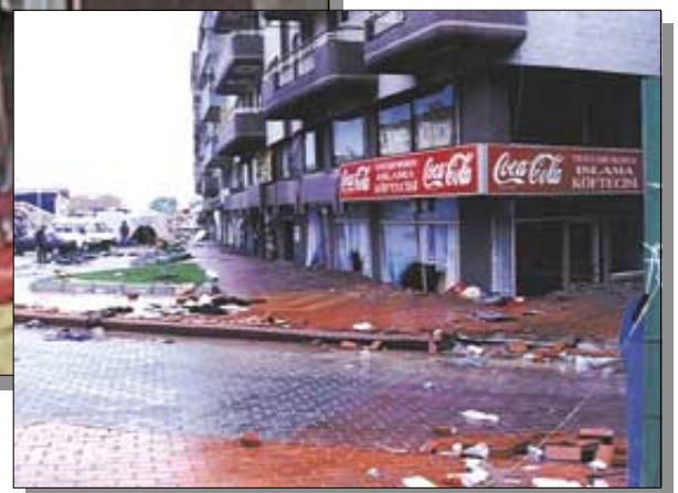
Figure 34. Building in Adapazari that sank 1.5 m uniformly into the ground when the soil beneath it liquefied and was pushed outward from beneath the building. Magnitudes of sinking were proportional to weight of building. Upper photograph by Thomas L. Holzer; lower photograph by National Institute of Standards and Technology.
