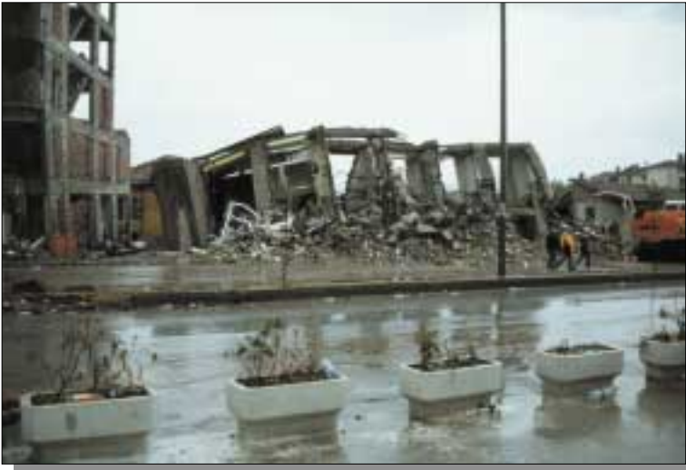
Figure 35. Buildings in Adapazari that either toppled or partially overturned because soil beneath them liquefied and weakened the foundation. Upper photograph by Thomas L. Holzer; lower photograph by Richard S. Olsen.
