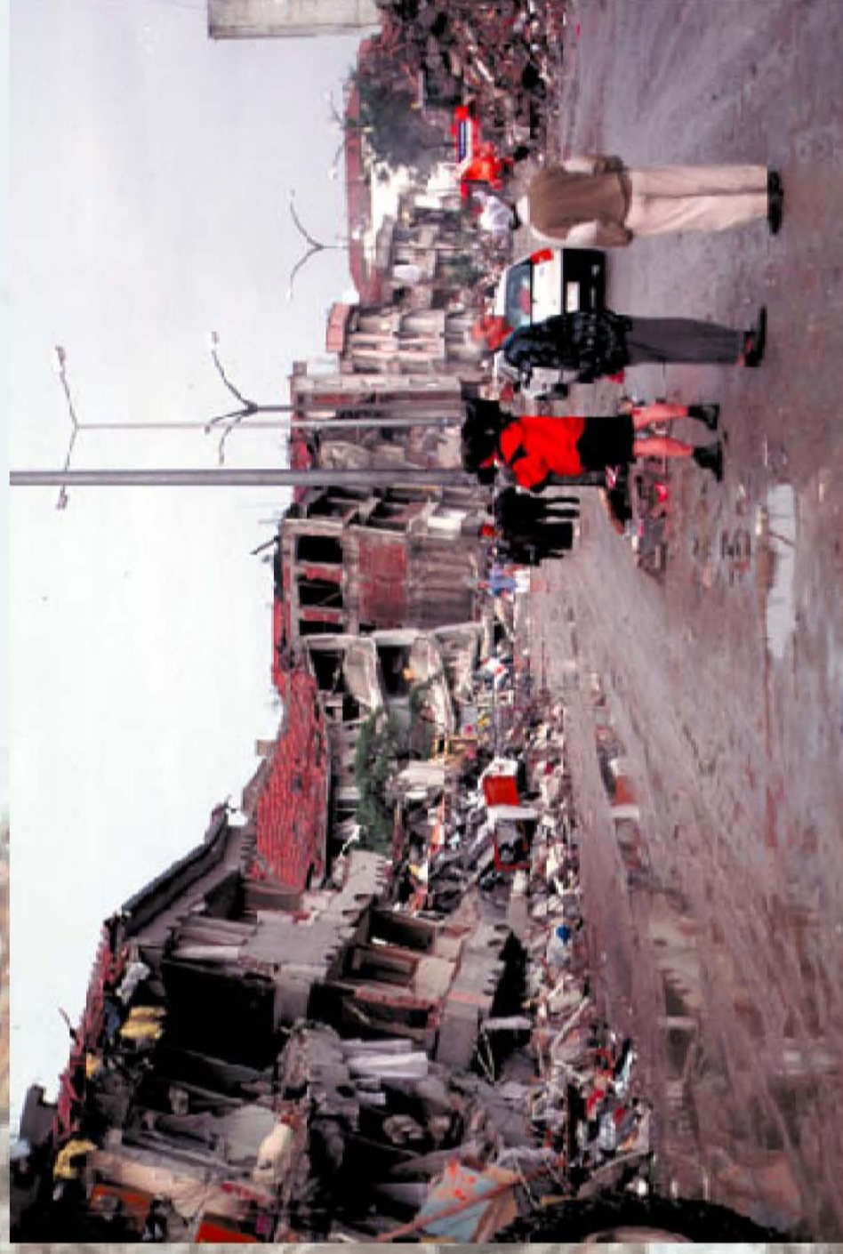
Figure 57. Street scene in Adapazarı following the Kocaeli, Turkey, earthquake. Extensive damage to concrete structures with little or no ductility displaced more than a quarter of a million people from their homes in the epicentral region. Photograph by Thomas L. Holzer.
