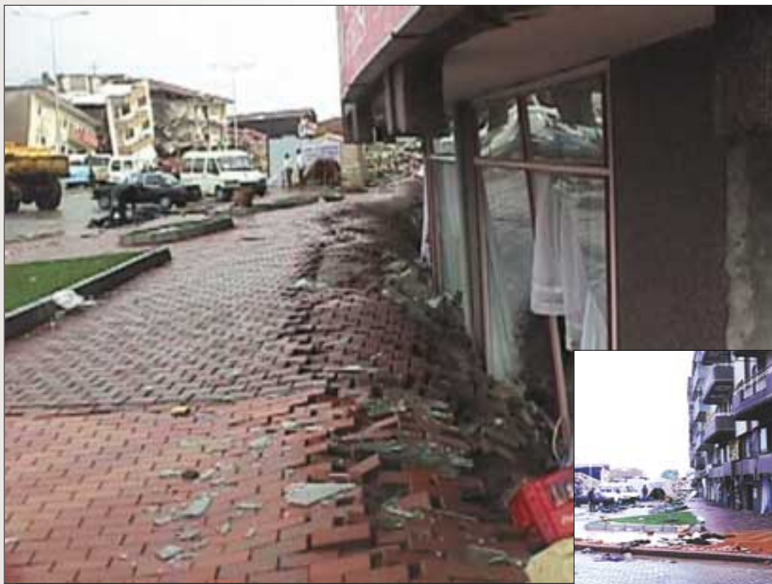
Figure 34. Building in Adapazari that sank 1.5 m uniformly into the ground when the soil beneath it liquefied and was pushed outward from beneath the building. Magnitudes of sinking were proportional to weight of building. Upper photograph by Thomas L. Holzer; lower photograph by National Institute of Standards and Technology.
