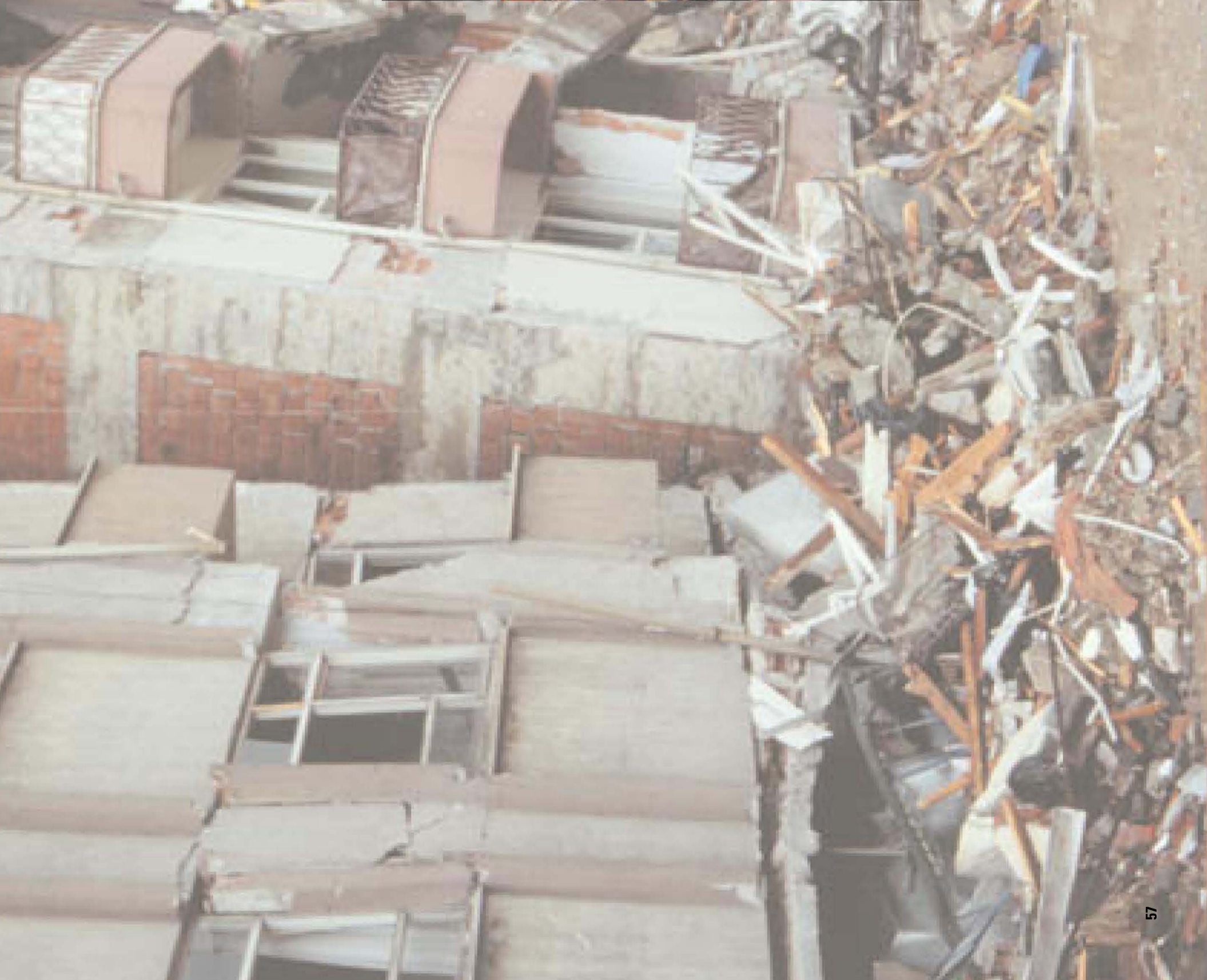
Figure 57. Street scene in Adapazarı following the Kocaeli, Turkey, earthquake. Extensive damage to concrete structures with little or no ductility displaced more than a quarter of a million people from their homes in the epicentral region. Photograph by Thomas L. Holzer.
