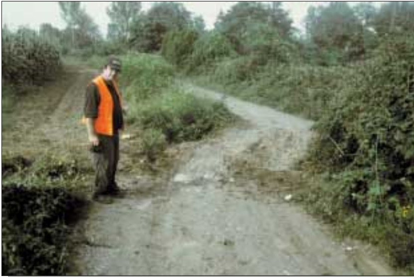
Figure 19. Road offset right laterally 4.66 m near Arifiye. Photograph by Robert Langridge.
