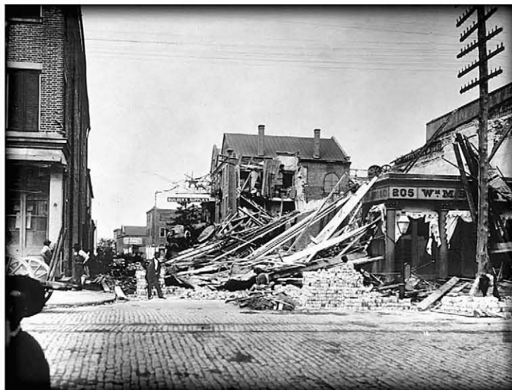
Figure 7. Location map (A) of the Charleston-Georgetown-Bluffton area in South Carolina and photograph (B) of damage from the August 31, 1886, earthquake. The 1886 earthquake produced significant liquefaction. Studies of paleoliquefaction features along the Coastal Plain of South Carolina and North Carolina have found evidence of multiple episodes of strong ground shaking during the past 3,000-5,000 years, but the faults that generated the earthquakes remain unidentified.
