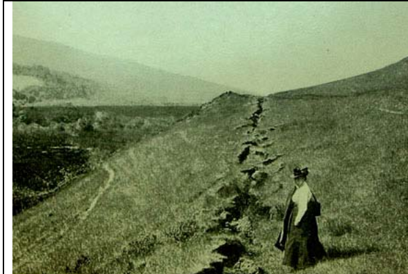
Figure 9-4. Photograph by Gilbert (1907) of surface rupture along the fault near Point Reyes Station. The view is looking northwest toward marshlands at the south end of Tomales Bay. The photograph illustrates a classic example of a sidehill bench. Note the extent of timber removal on Inverness Ridge in the distance.
