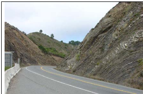
Figure 8-16. Road cuts along Highway 1 expose interbedded layers of Paleocene-age deep sea fan deposits (turbidites). This view is looking east from a small pull off at the top of the ridge of San Pedro Mountain. Note that this pull off is not recommended as a fieldtrip stop because of high traffic volume along the highway. Coastal travelers can more safely access similar deposits of Cretaceous age at Bean Hollow State Beach or near Pigeon Point south of Half Moon Bay.
