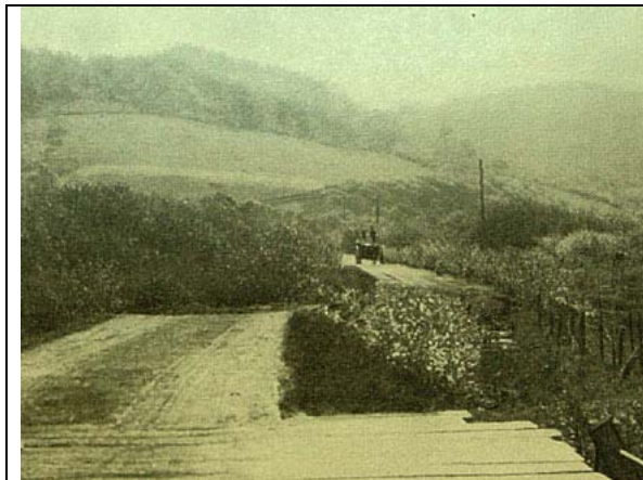
Figure 9-6. This view of an offset road near Point Reyes Station shows 20 feet of horizontal slip cause by the 1906 earthquake. Photograph by Gilbert (1907).
