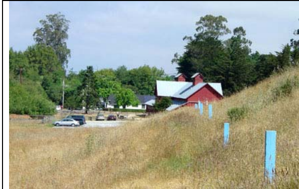
Figure 9-9. Blue posts mark the trace of surface rupture by the 1906 earthquake. The Shaffer Ranch barn was built on the trace of the fault and was damaged by the earthquake. This view is looking north from the offset fence exhibit area along the Earthquake Trail.
