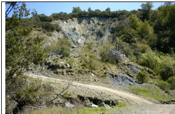
Figure 3-3. An active landslide along the Limekiln Trail causes trail closure during wet seasons. In recent winters the road has been offset by several meters. During dry months the slide area is relatively safe to examine but be aware that rocks and soil in steep slopes may be unstable from recent movement. The landslide formed in deeply weathered serpentinite, but fresh blocks of rock material have accumulated in the stream at the toe of the slump.
