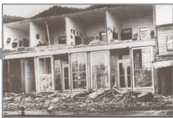
1906—Damage in Healdsburg
