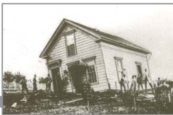
1868—Damage in Hayward
