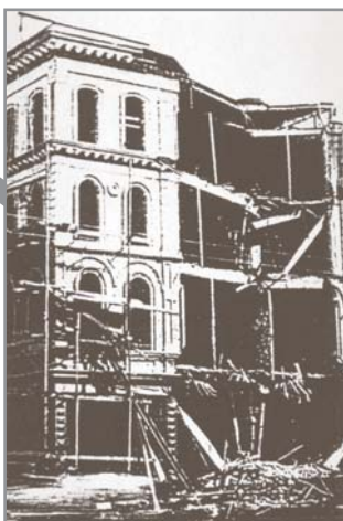
1865—Damage in San Francisco
