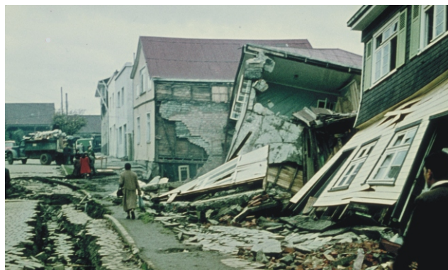
Cracked street and variably damaged buildings, Valdivia.
