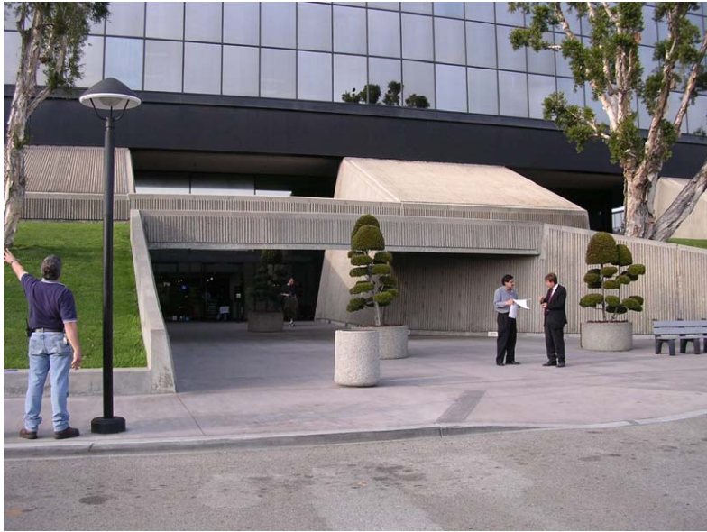
Figure 4. Massive concrete piers at the base of the building, extending from the ground floor to the second floor. The steel moment frame begins at the large black band (plate girder) directly above the piers.
