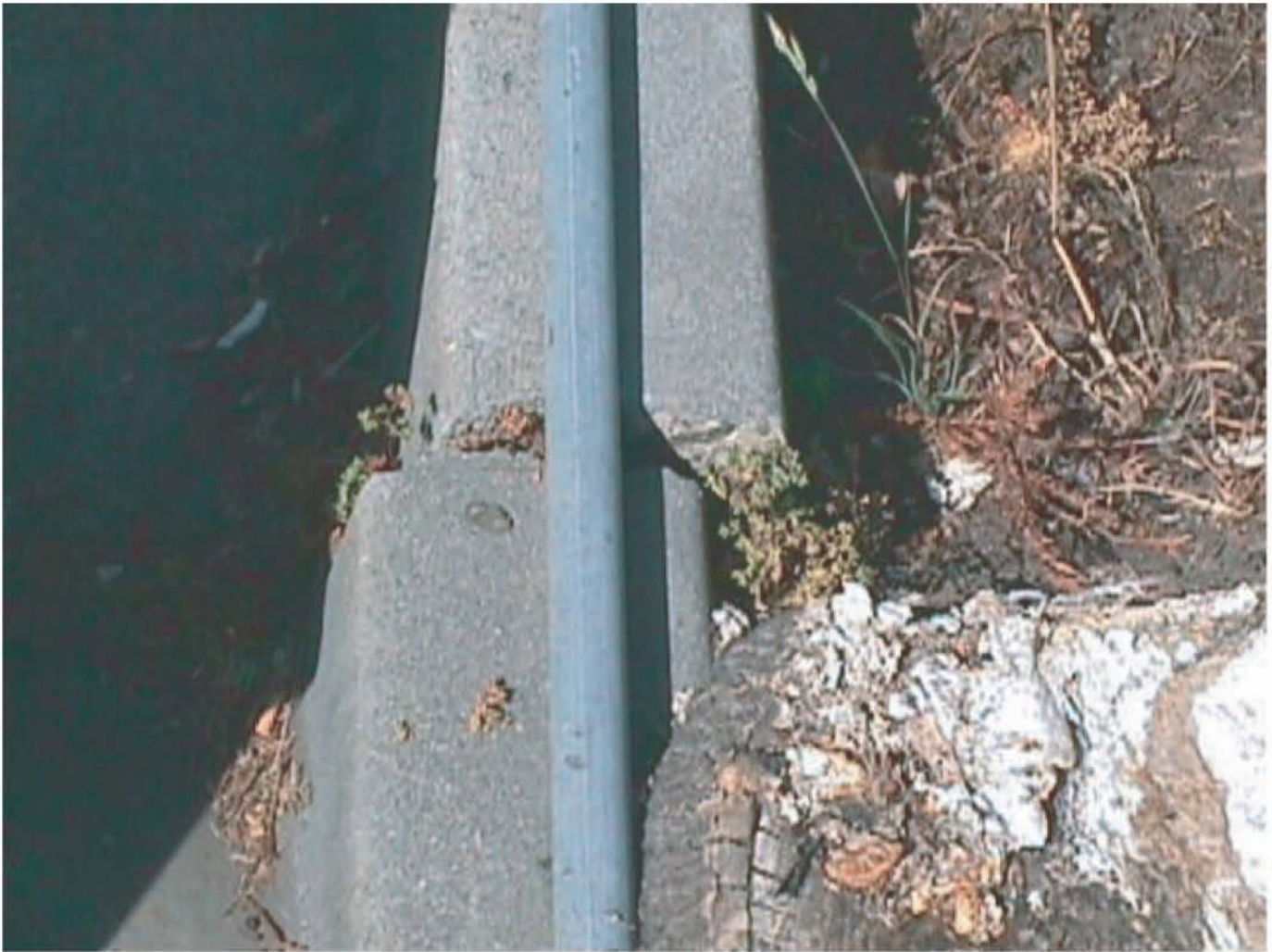
Figure 3-1. Photograph of evidence of right lateral creep on the mapped active strand of the Hayward Fault. This offset curb is in the parking lot between A and B streets in downtown Hayward.
