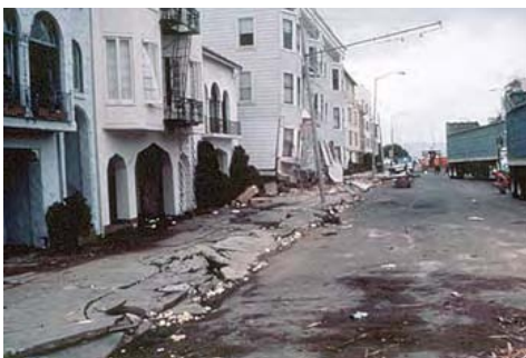
Sandy soils can shake so much that they liquefy, causing buildings to sink and buried pipes to break. In steep hilly terrain, landslides can also be triggered (USGS photo).
