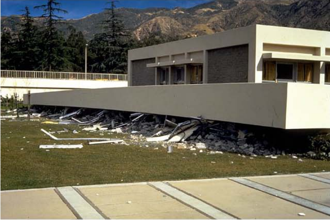
Figure 4-8. Second story of psychiatric unit, Olive View Hospital, 1971, pancaked over first story. This and other damage at Olive View Hospital emphasized the poor seismic performance of NDRC construction.
