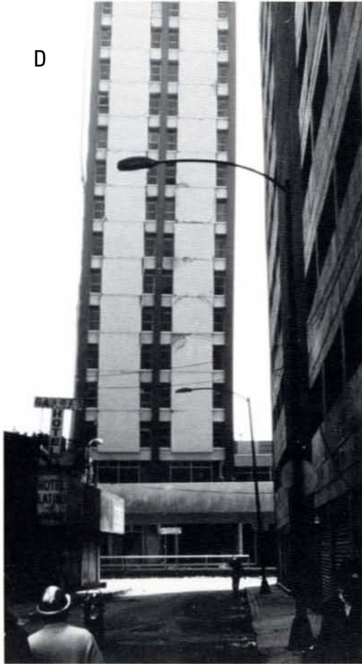
Figure 4-7. Damage in Mexico City, September 19, 1985, from an earthquake some 200 km distant. (A) Collapse of a 21-story building on top of a 14-story building in the Pino Suarez complex. Three towers are left standing with extensive damage to the two 21-story towers. Source: Bob Reitherman; (B) Failure in the welds connecting the flanges and webs of built-up box column possibly led to local flange-buckling of the column and eventual collapse. Source: Bob Reitherman. (C) Debris of tower collapse spilled on to the streets. Source: Mehmet Celebi, USGS. (D) This 21-story steel building remained standing, but was leaning six feet out of plumb at the roof level due to yielding that resulted in a permanent interstory drift (Source: Jim Beck, Caltech). Such permanent tilting would most likely render the vertical transportation system (elevators) unusable due to misalignment. In addition, doors to staircase shafts may be jammed due to deformation of the frames, possibly hampering evacuation efforts.
