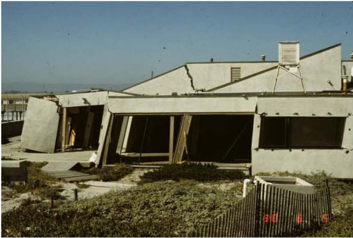
Figure 3-24. Photo of the Moss Landing Marine Laboratory facility, Monterey County, CA, destroyed as a result of about 1.2m of displacement due to liquefaction-induced lateral spreading caused by the M 6.9 1989 Loma Prieta earthquake. Ground motions at this site were sufficiently low that the structure would likely have survived the earthquake with minimal damage had the lateral spreading not occurred. Photograph by John Tinsley, U. S. Geological Survey.
