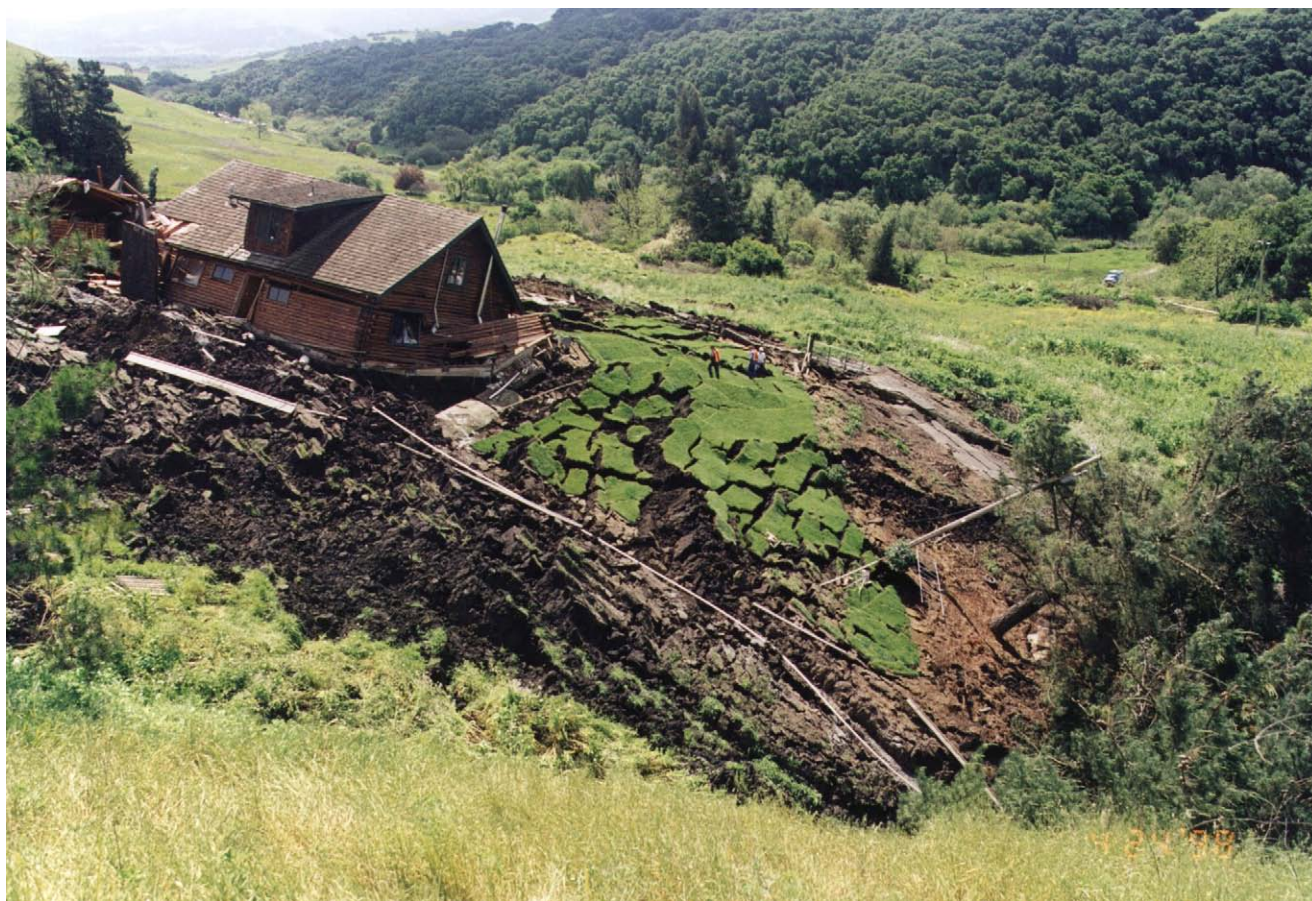
Figure 2-1. Reactivated deep-seated landslide (earth flow) near town of Aromas, northern San Benito County, that cut natural gas service to 60,000 Santa Cruz County residents on April 23, 1998. Photograph by W.R. Cotton.
