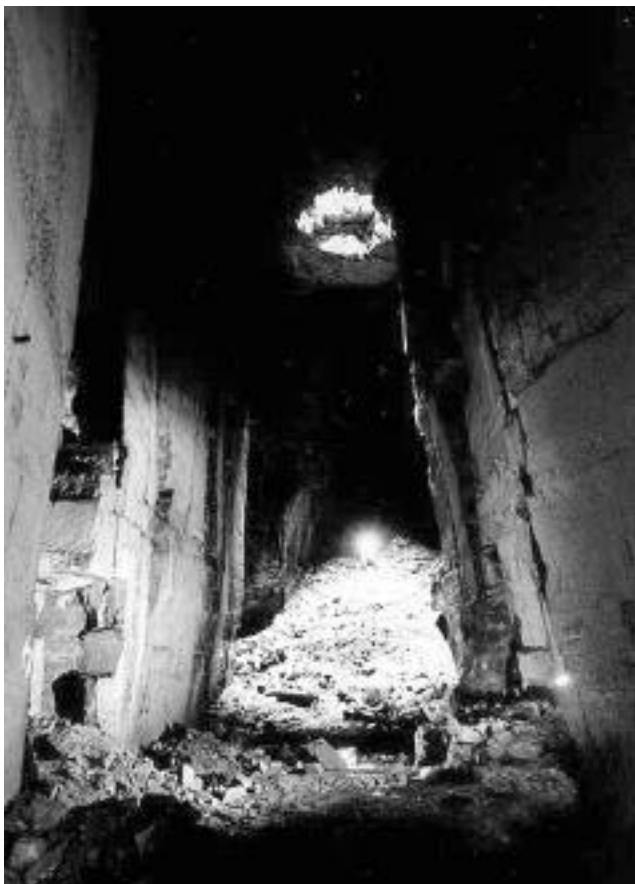
Fig 10. Recent photograph of the interior of the "Box Cathedral," a large cavern in Wiltshire, England, that was worked by hand from a vertical shaft, beginning in 1830. This room has an unsupported span of 40 ft (13 m), a length of 200 ft (61 m), and a height of 90 ft (27 m).
