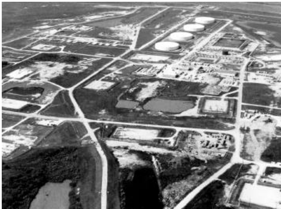
Fig 3. Aerial photograph of the surface features at Bryan Mound, Louisiana, a site of the Strategic Petroleum Reserve. Note the large tanks and ponds that are typical of a storage site.
