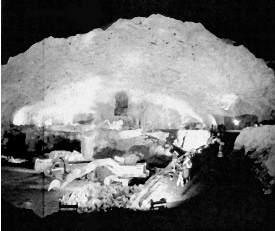
Fig 11. Photograph of the interior of the Olympic sports hall at Gjøvick, Norway, during construction in 1991 [from Wheeler, 1992]. The main hall has an unsupported span of 61 meters, among the largest constructed in hard rock, a length of 90 m, and a height of 25m, at a depth of 25-50 m.
