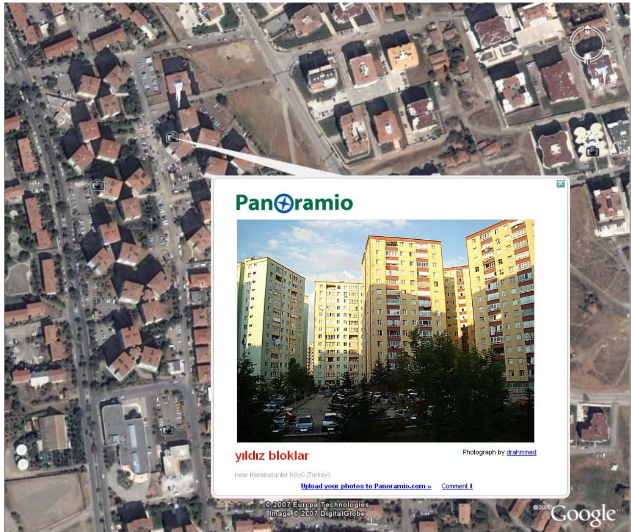
Figure 16. Photograph showing typical multistoried reinforced concrete apartment buildings with masonry infill walls in Ankara, Turkey
